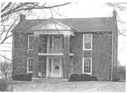
Nave-Brown House (JS-144) Built 2 nd quarter of the 19 th century
