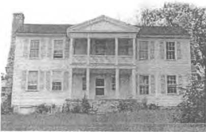
Matthews House (JS-96) Built 1825-1850, log structure, dogtrot plan
