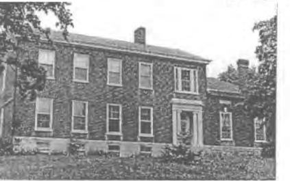
Chaumiers des Prairies (JS-169) Greek Revival portion 1820-1840
