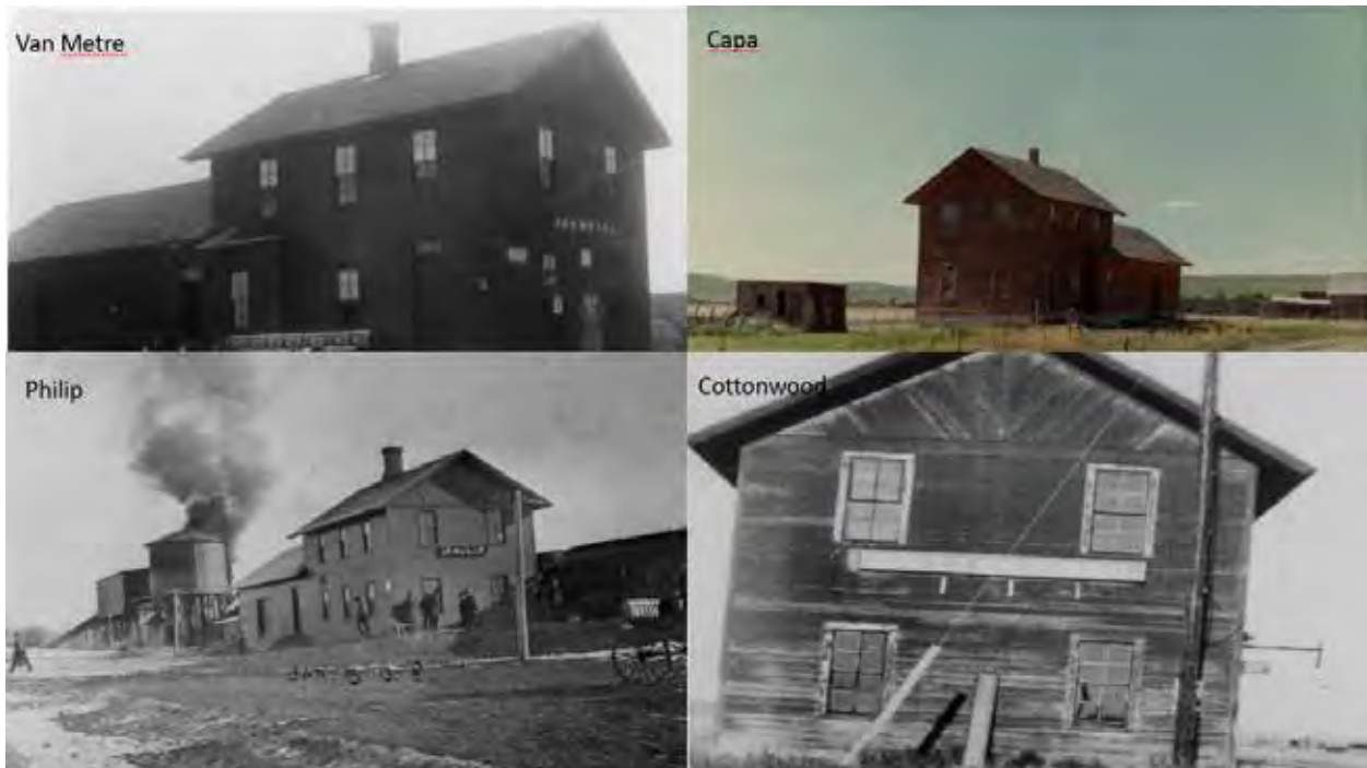
The Van Metre, Capa, Cottonwood, and Philip depots, all of which had decorative stick work in the gable. (Photos Courtesy South Dakota State Historical Society Archives)
