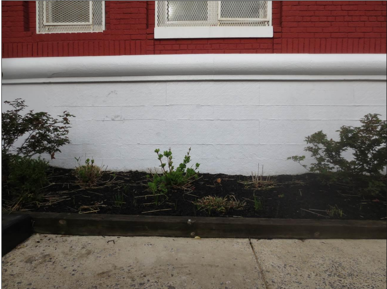
Exterior: Detail of foundation on façade, looking west
