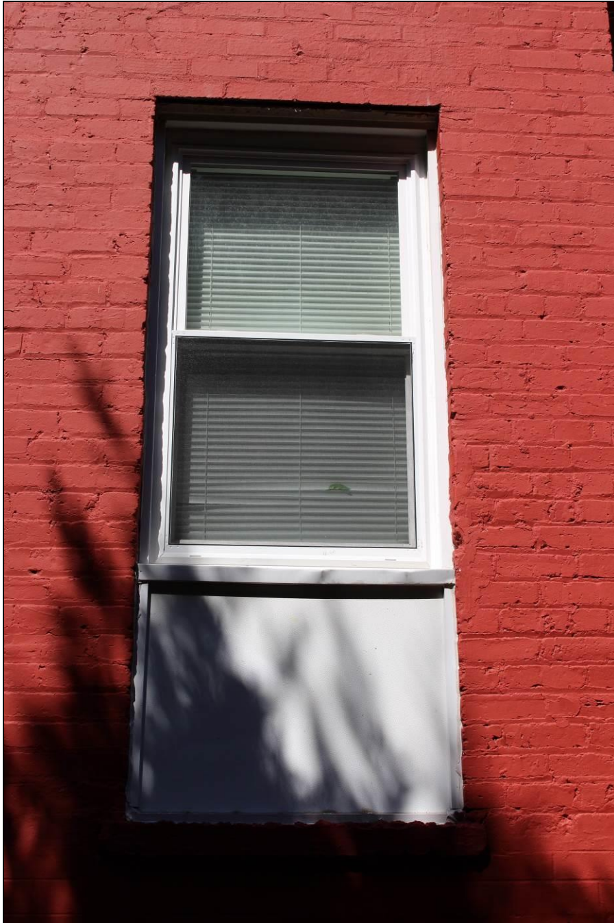
Exterior: Window detail on south elevation
