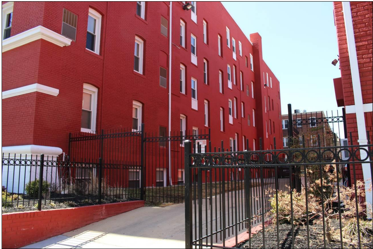
Exterior: North elevation, looking southwest
