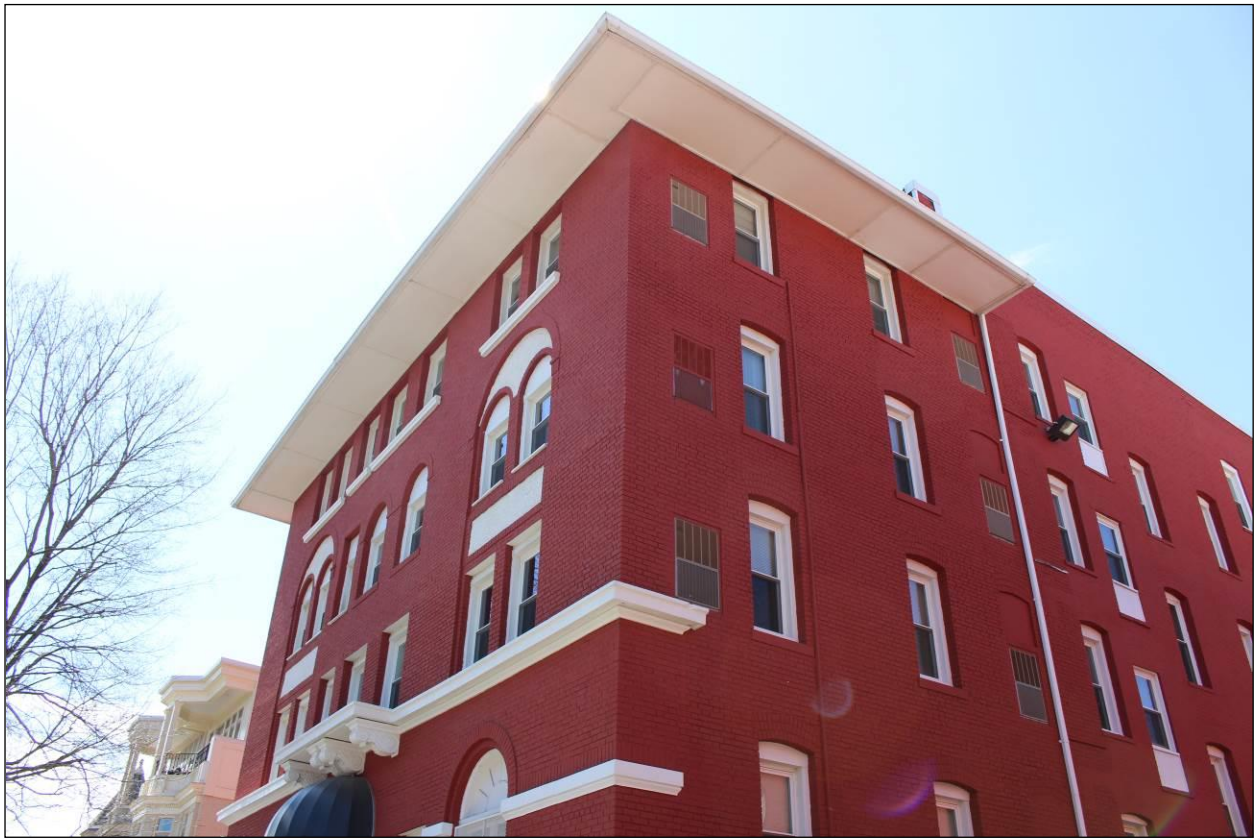
Exterior: Northeast corner and façade, roof detail, looking southwest
