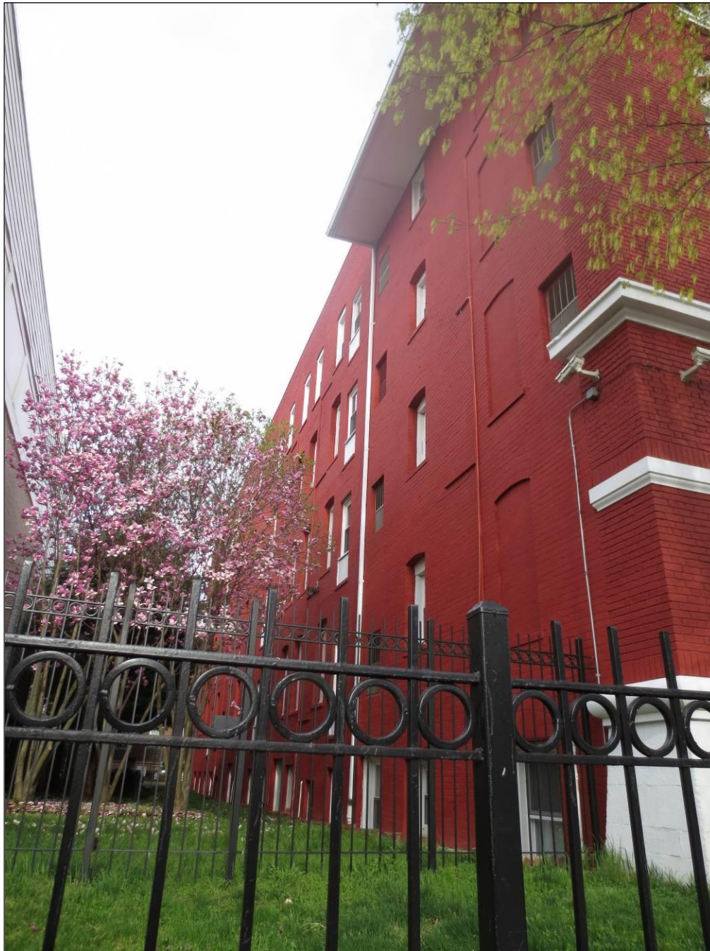
Exterior: South elevation and side yard, looking west
