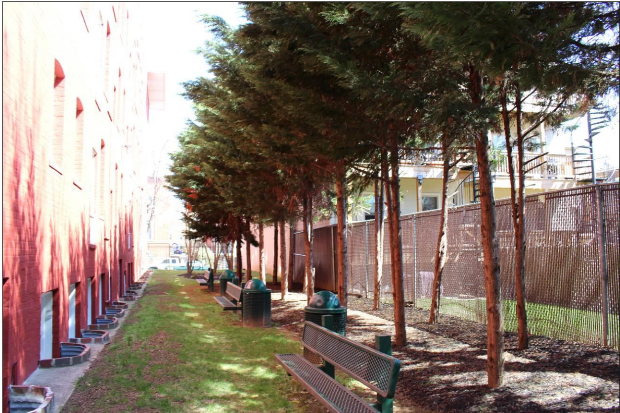
Exterior: South elevation and side yard, looking east
