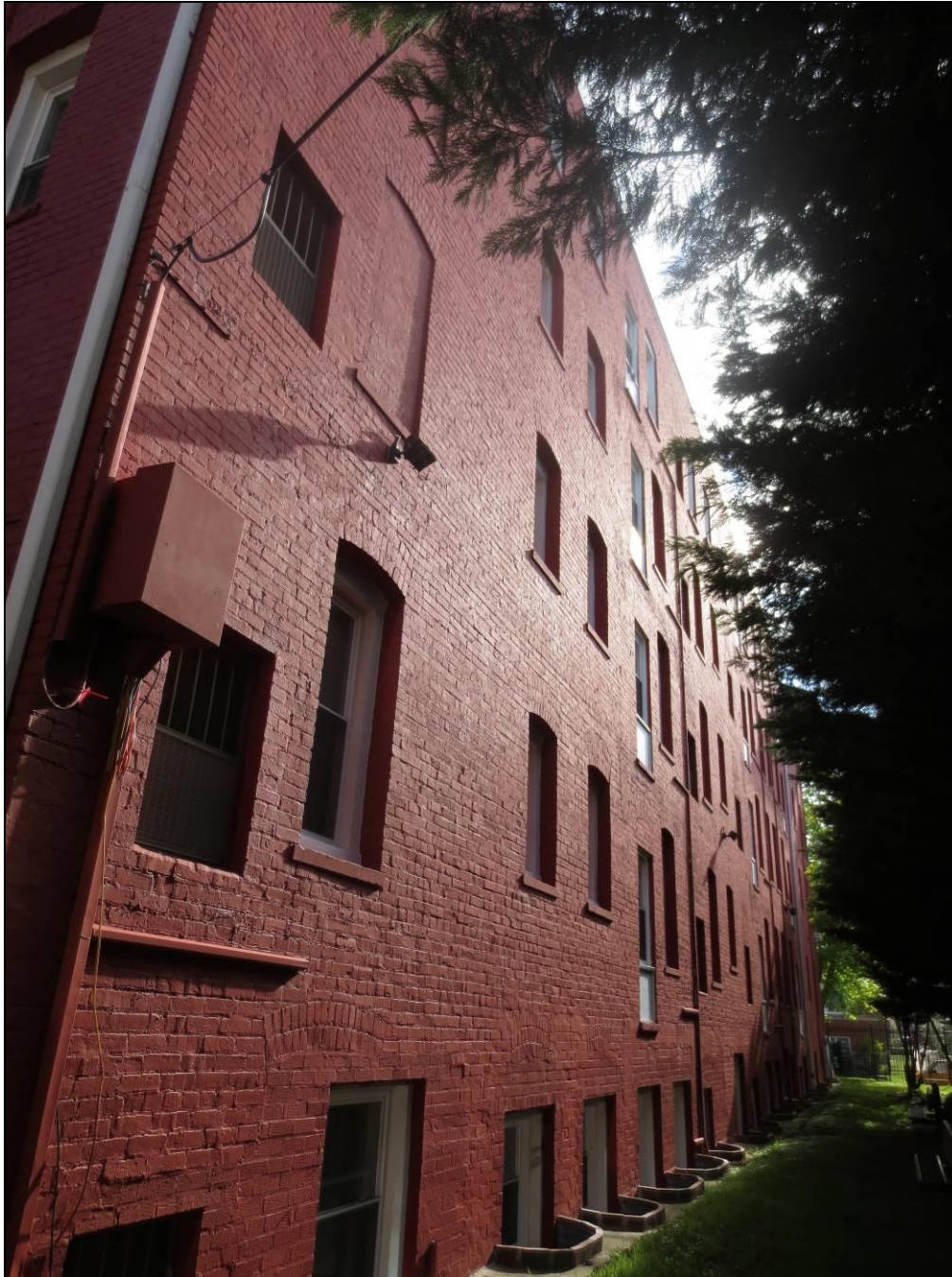
Exterior: South elevation, looking northeast
