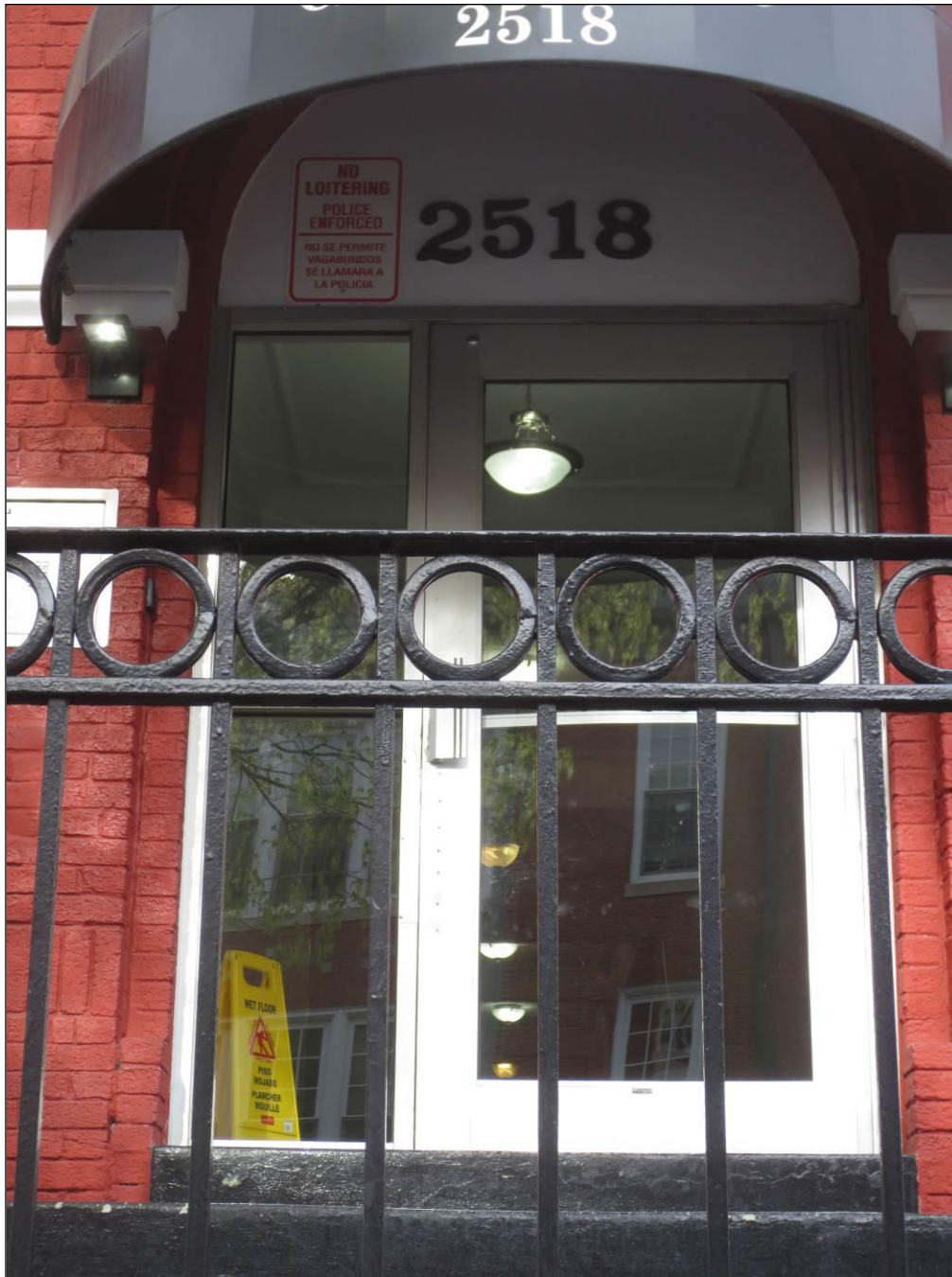
Exterior: Detail of front entry on façade, looking west
