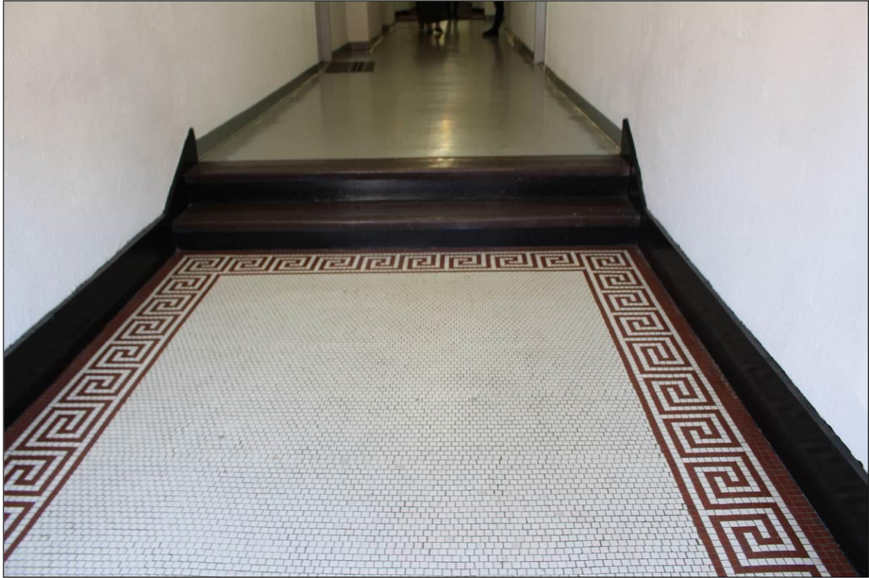
Interior: Detail of entry vestibule mosaic floor, looking west
