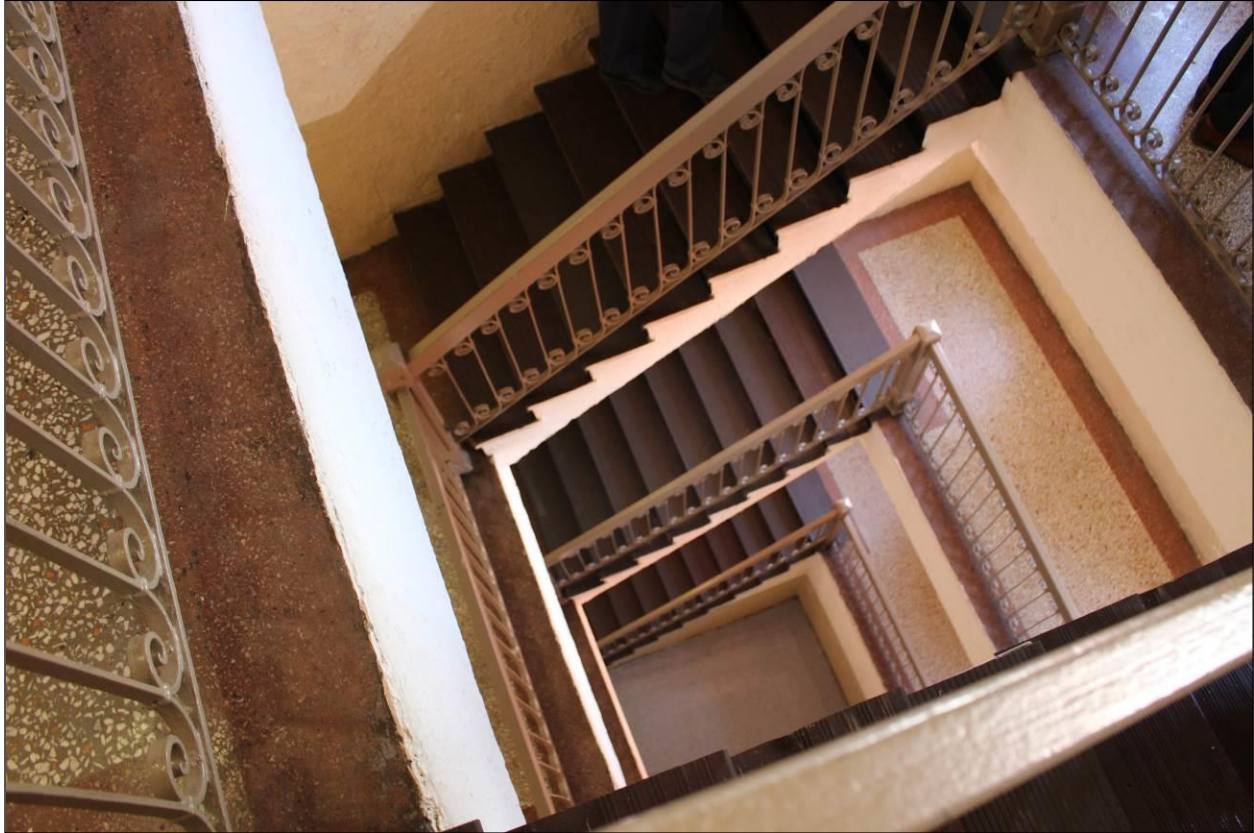
Interior: Detail of stairwell from fourth floor, looking down
