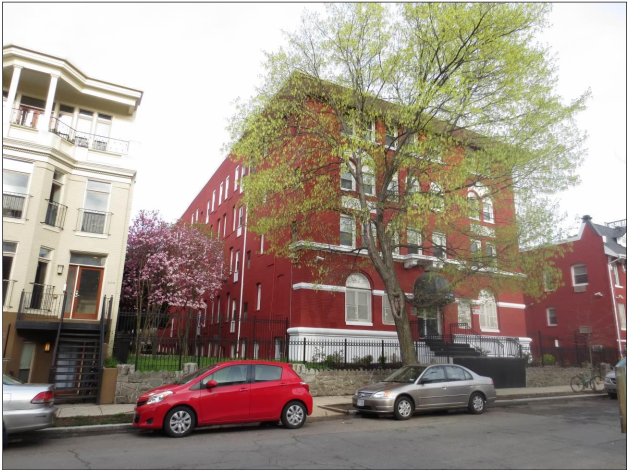
Exterior: Façade and south elevation, looking northwest
