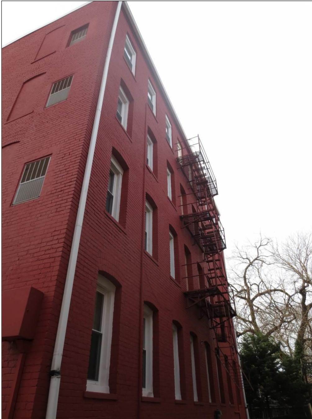
Exterior: Rear (west) elevation, looking southeast
