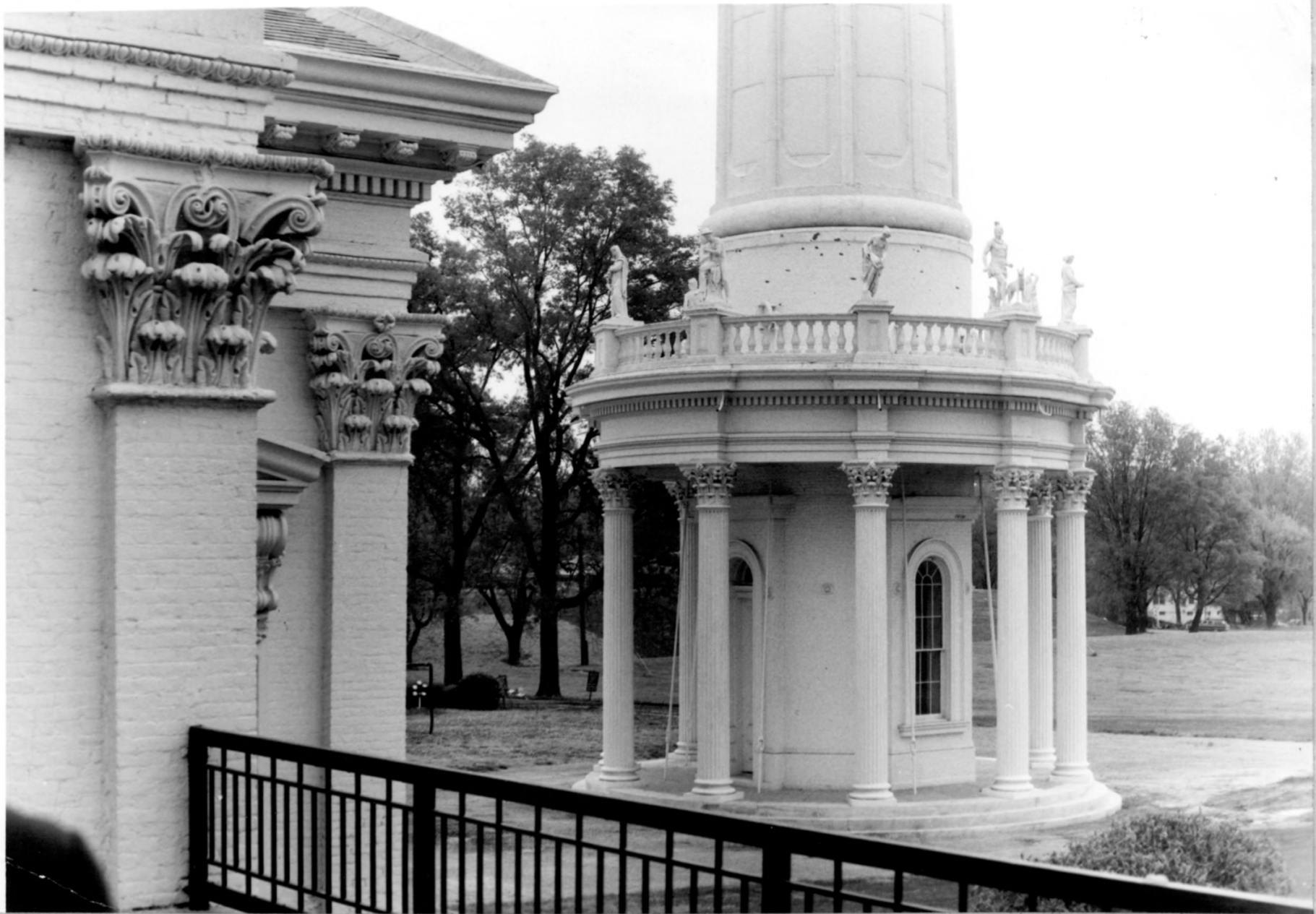
Louisville Water Company Pumping Station, Louisville, Kentucky
