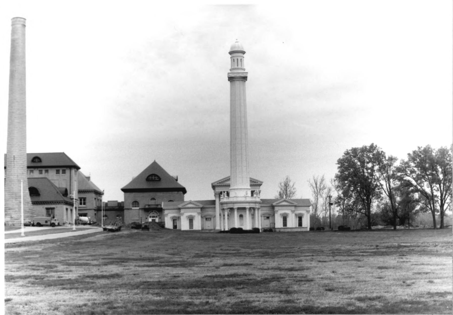
Louisville Water Company Pumping Station, Louisville, Kentucky
