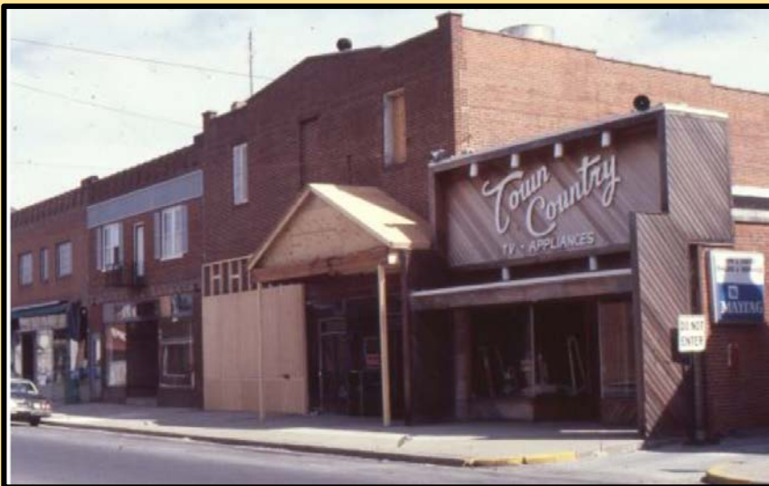
1974 façade renovations - fur strips and plywood cover Carrara Glass, plate glass store windows, and main entrance is modified
