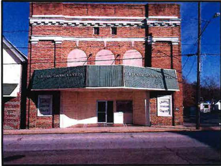
Waller Theatre – Laurel, DE Renovated and now functions as a senior center.
