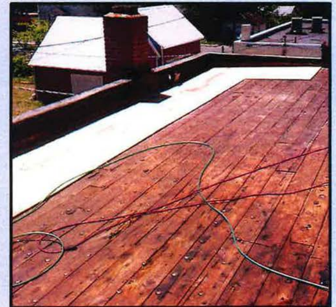
Original milled-planed wooden roof with glazed tile flashing
