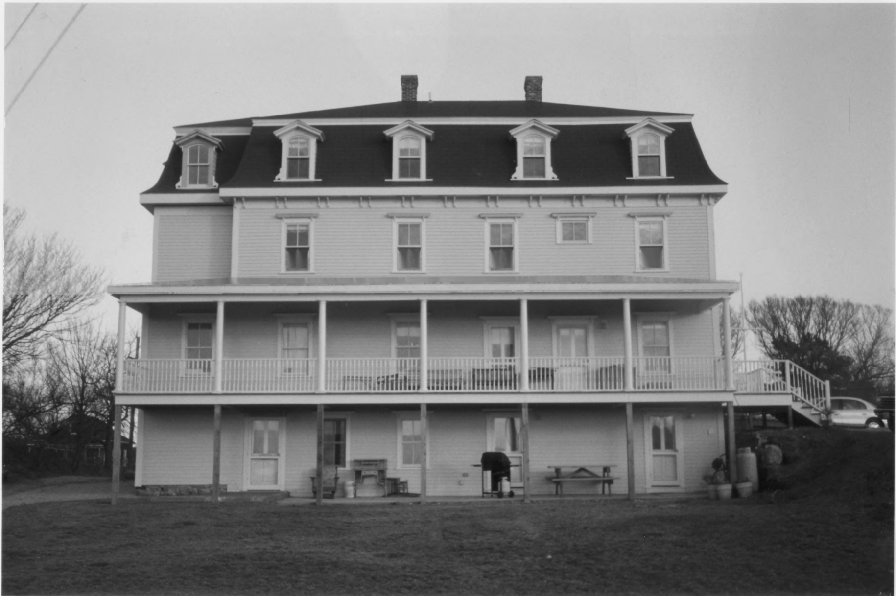
Hygeia House Washington County, New Shoreham, RI Photo #2 of 5
