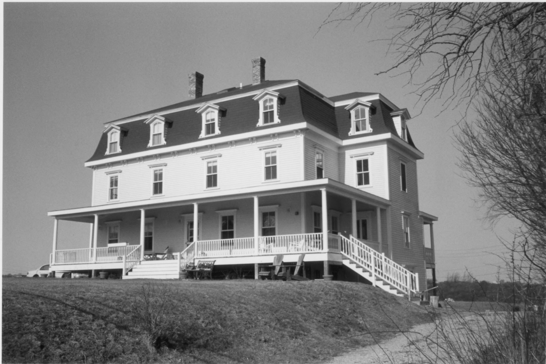
Hygeia House Washington County, New Shoreham, RI Photo # 1 of 5
