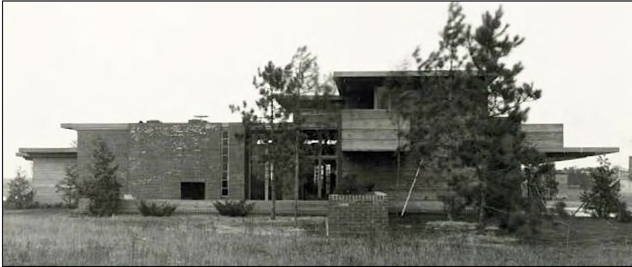
Figure 3: Schwartz House exterior, Northwest elevation, 1939.
