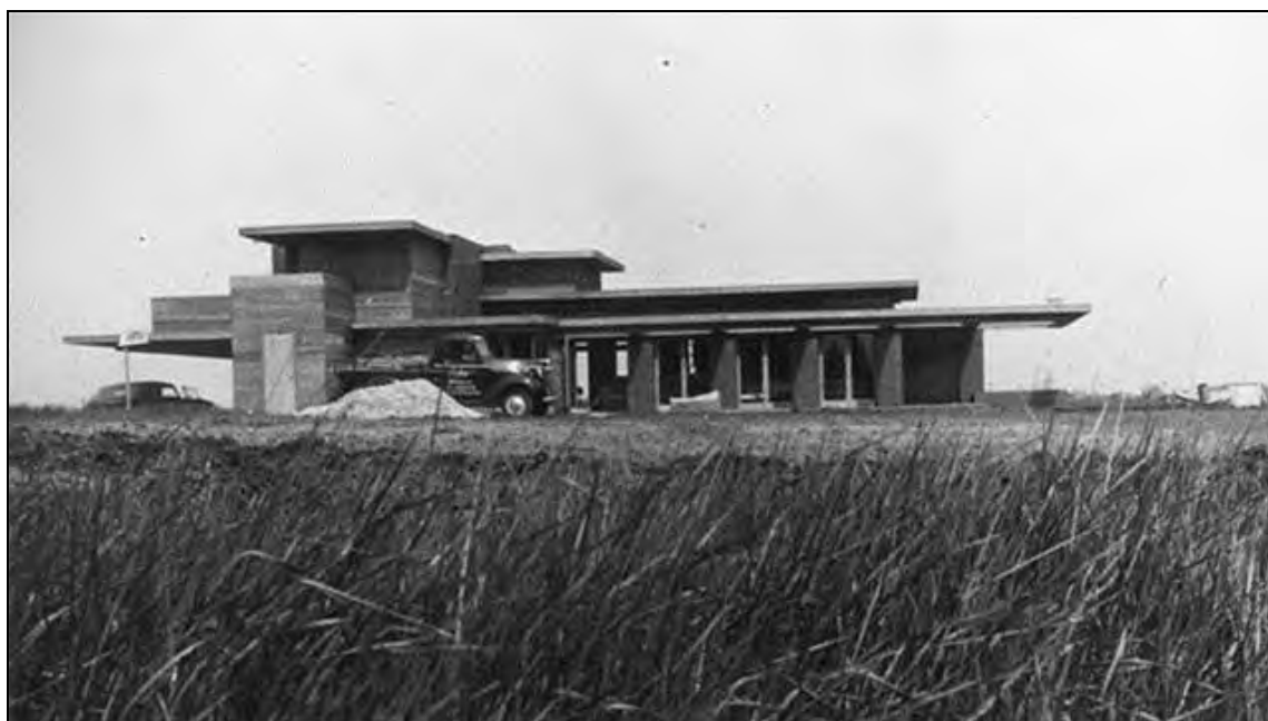
Figure 2: Schwartz House under construction, Southeast elevation, 1939.
