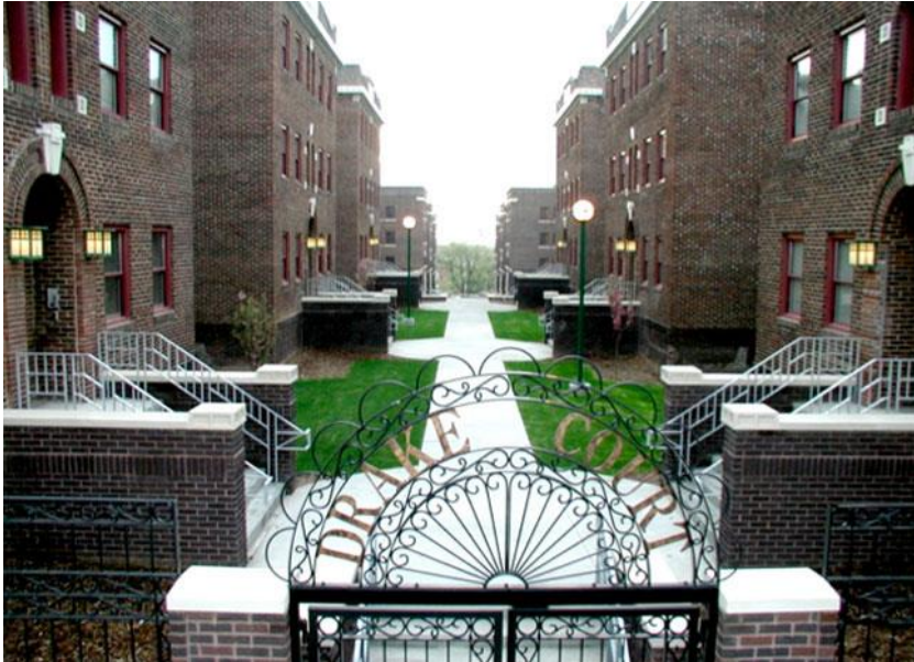
Drake Court Apartments built by the Drake Realty and Construction Company located at Jones Street between 20 th and 23 rd Streets. Drake Court was a complex consisting of multiple buildings facing a courtyard. The Apartments were constructed between 1916 and 1921. The complex was listed in the NRHP in 1980 and amended in 2014)
