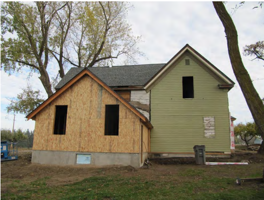
3 of 22: West façade/rear of farmhouse in Oct 2014
