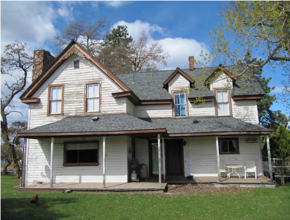
6 of 22: East Facade of farmhouse in 2013 prior to rehab
