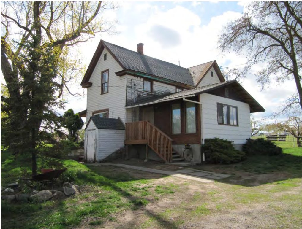
7 of 22: Northeast corner of farmhouse in 2013 prior to rehab
