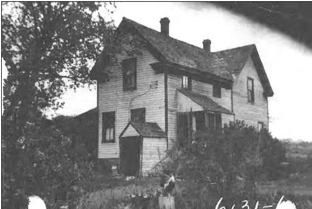
1930 photograph of Palmer Farmhouse, northwest rear corner
