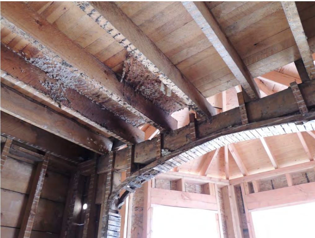
13 of 22: Uncovered arch in bay window area during rehab
