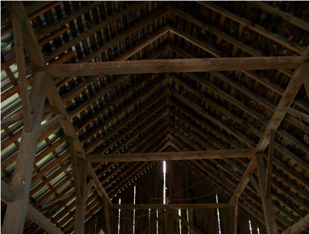
18 of 22: Interior of barn
