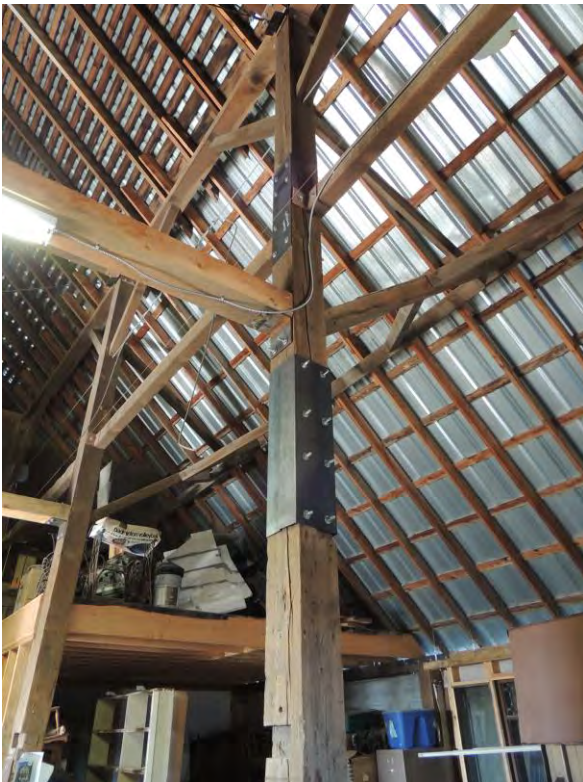
19 of 22: Interior of barn showing new support elements
