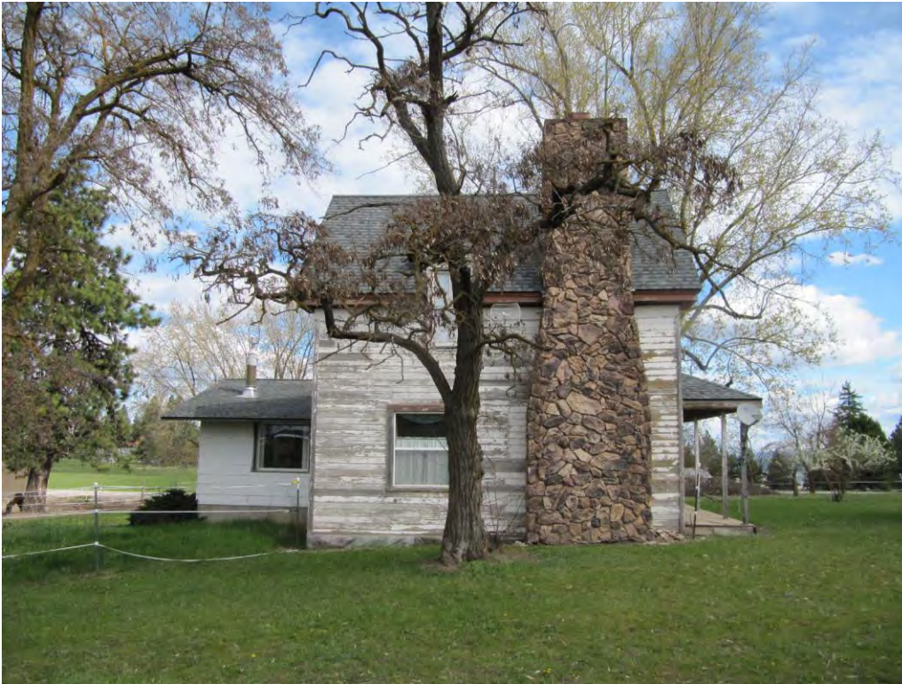
8 of 22: South face of farmhouse prior to rehab
