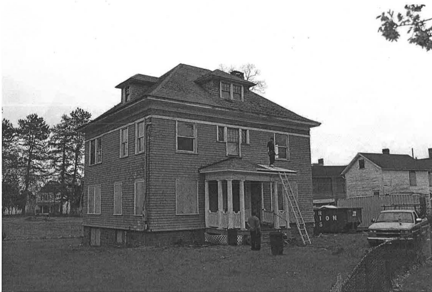
West (front) and north (side) elevations of 1914 Swift house from Love Lane. Camera facing southeast. Photograph 13 of 18.
