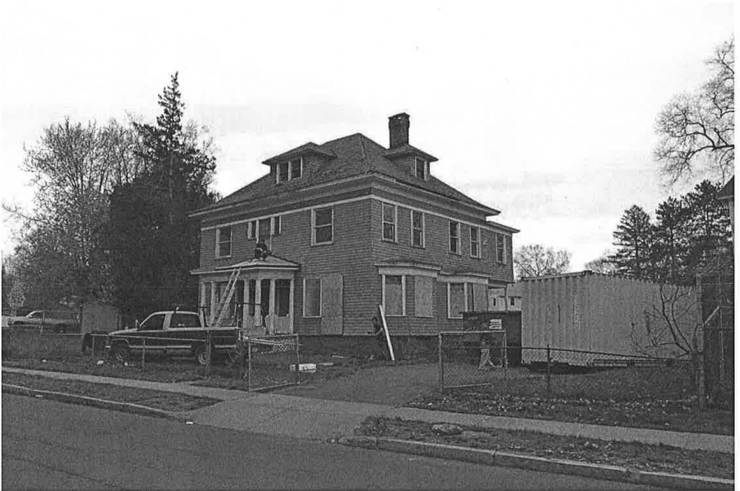
West (front) and south (side) elevations of 1914 Swift house from Love Lane. Camera facing northeast. Photograph 14 of 18.
