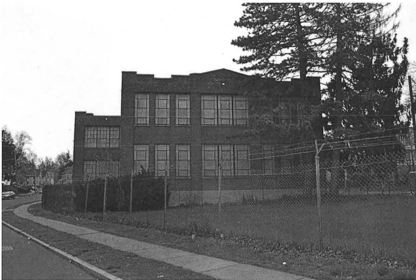
South (front) elevation of factory from Love Lane, showing 1929 block with side ell. Camera facing north. Photograph 5 of 18.
