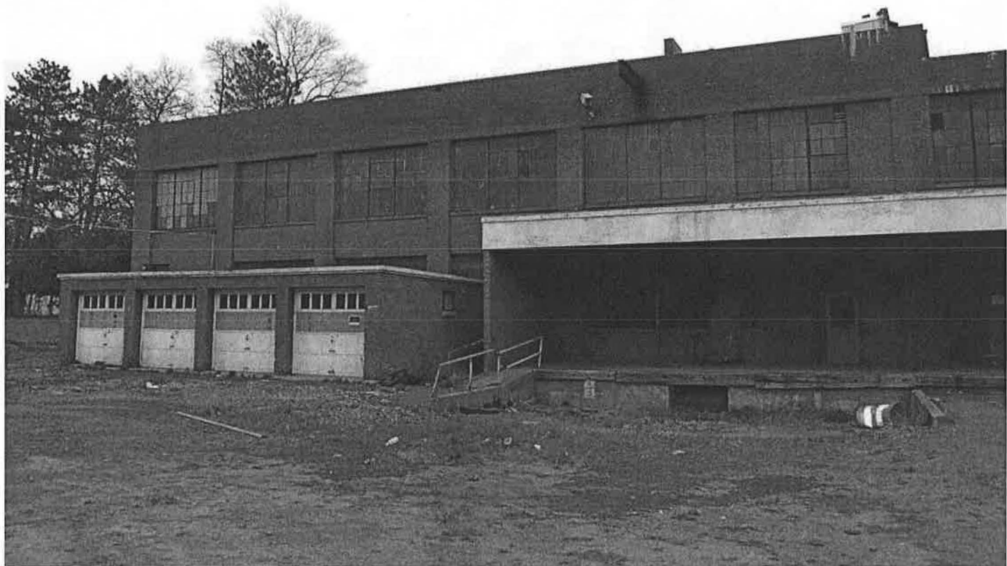
West (front) and south (side) elevations of 1941 garage from Love Lane, 1948 block at rear. Camera facing northeast. Photograph 17 of 18.
