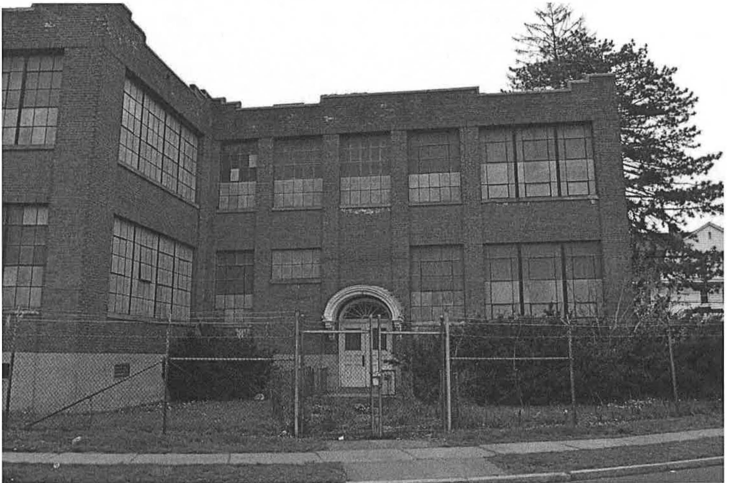
West (side) elevation of factory from Love Lane, showing primary entry in 1929 block. Camera facing east. Photograph 8 of 18.
