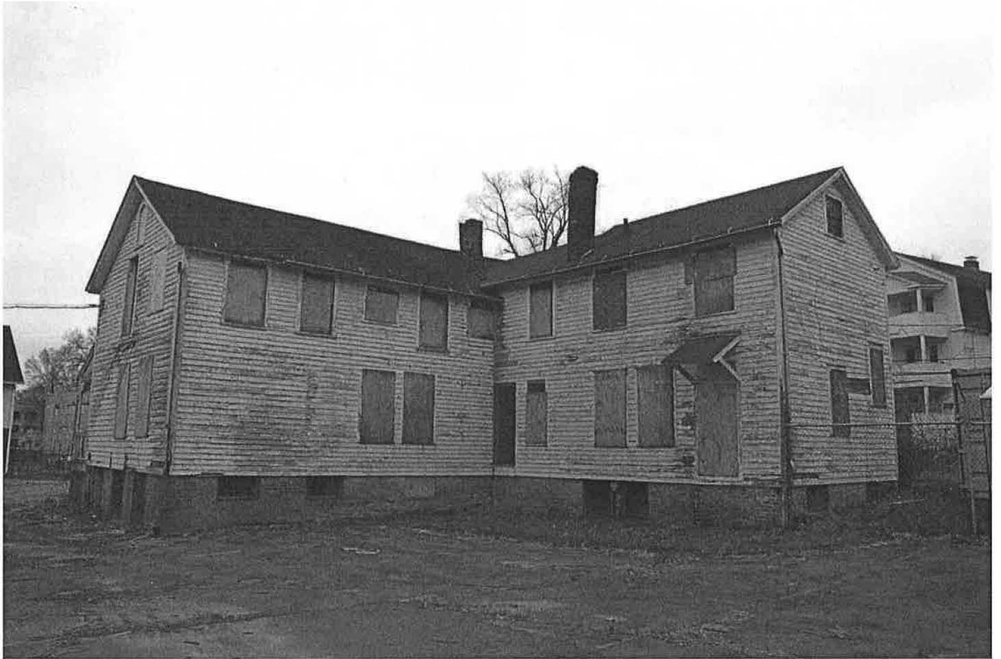
North (rear) and east (side) elevations of Swift homestead (c. 1887) from interior of property. Camera facing southwest. Photograph 12 of 18.
