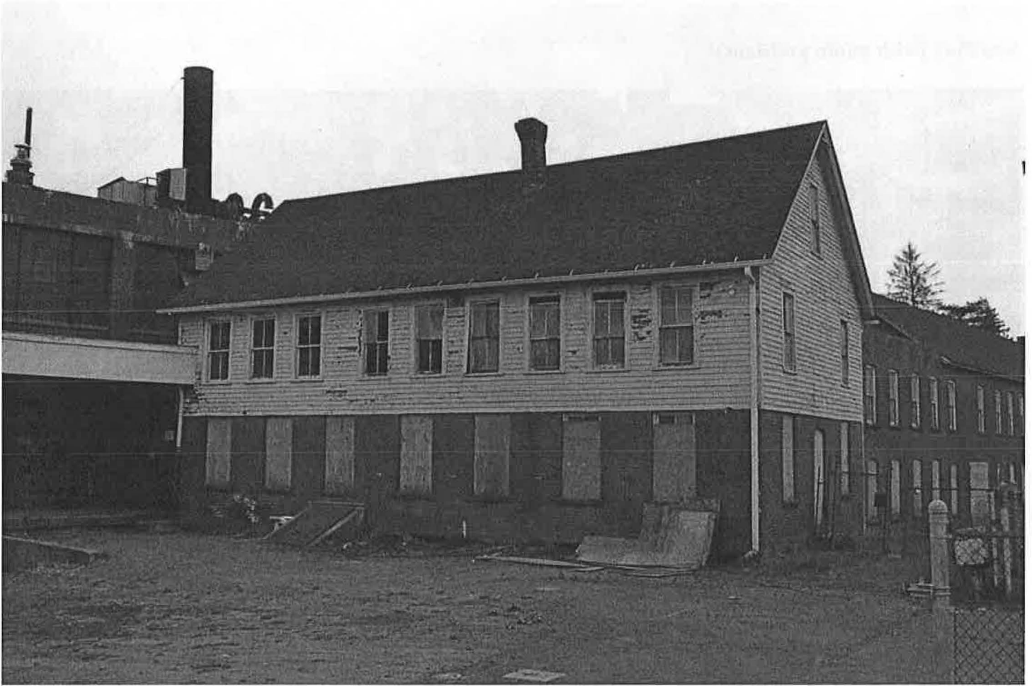
North (front) and west (side) elevations of original workshop (c. 1890) from Love Lane. Camera facing southwest. Photograph 1 of 18.
