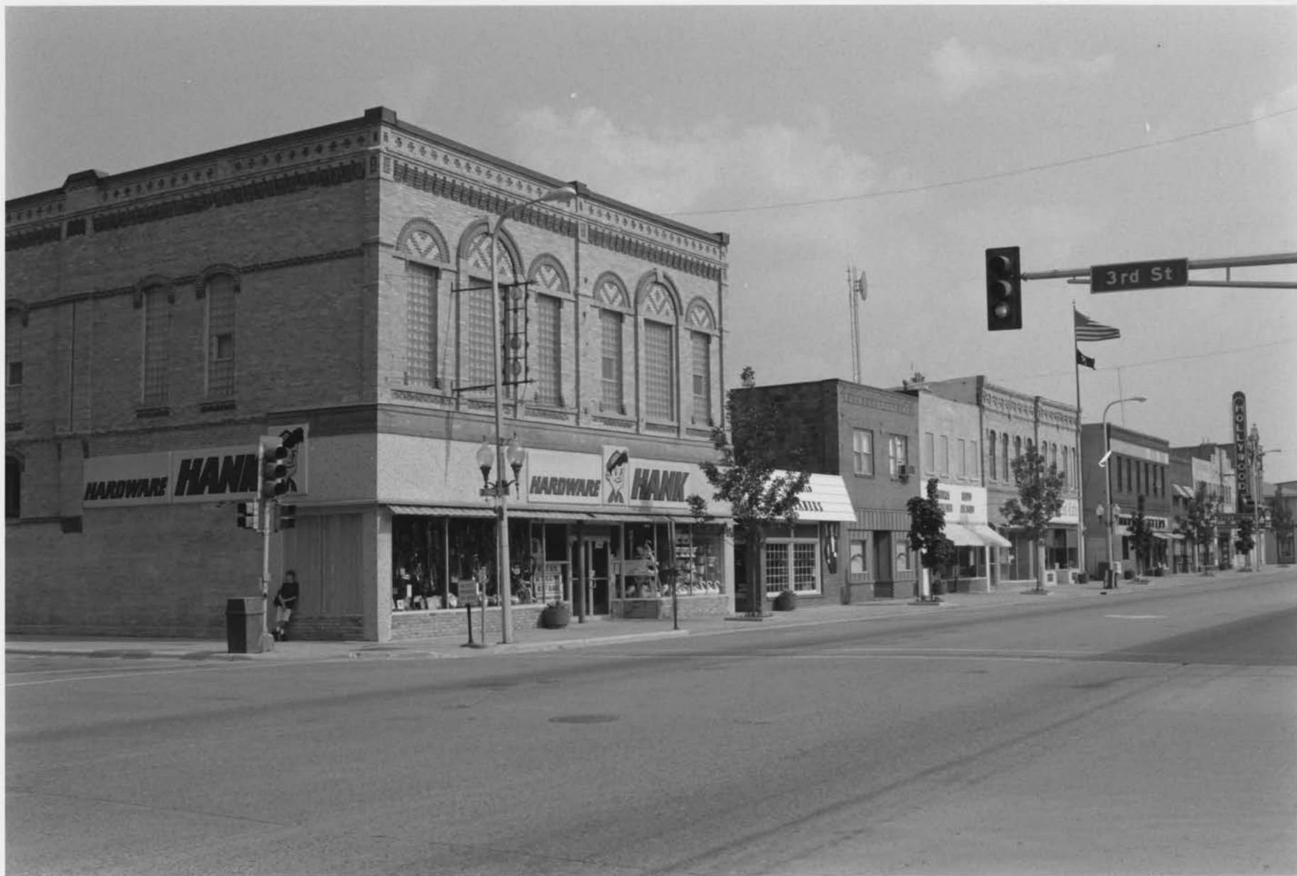
Streetscape: Looking SE at East side of Sibley Ave. #242 is on left. Litchfield Commercial Historic District meeker Co., MN 012576-4A
