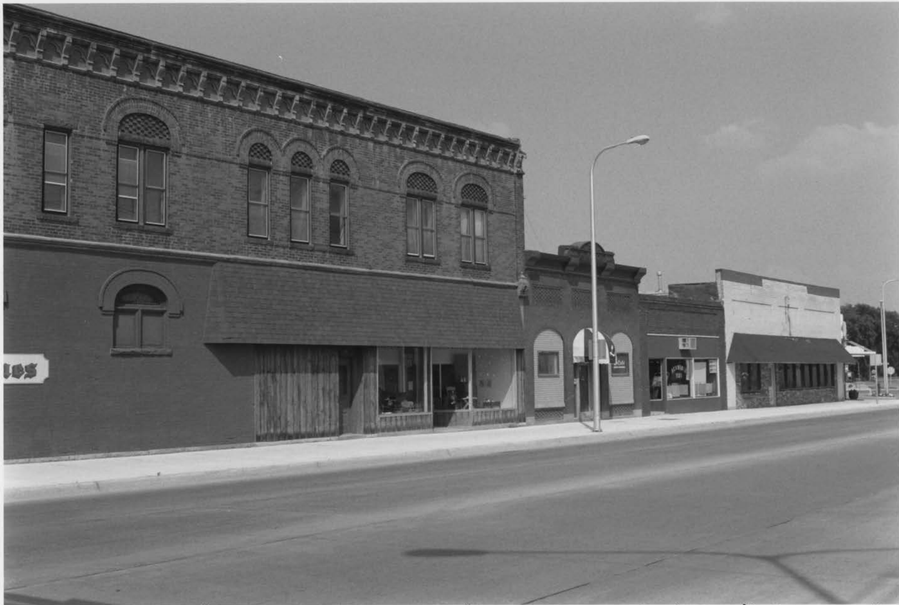
Streetscape: Looking NE at Northside of Depot St. East; # 100 is seen on Left Litchfield Commercial Historic District meeker co., mn 010578-2
