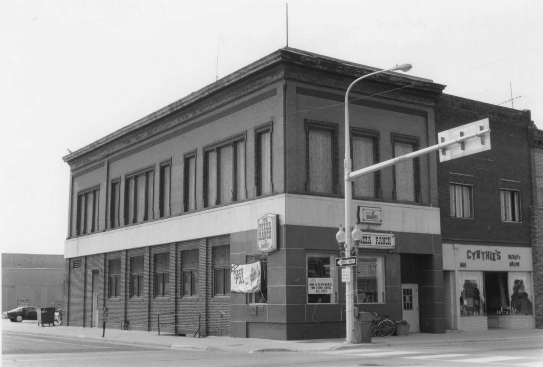
First National Bank, 201 N. Sibley Ave. Litchfield Commercial Historic District Meeker Co., MN 010571-9
