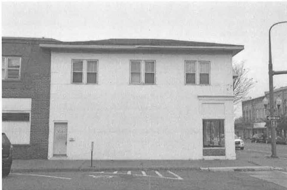
Photo 4. The north facade (2017, facing southeast).
