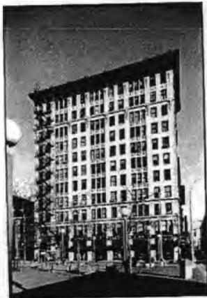
The Republic Building
