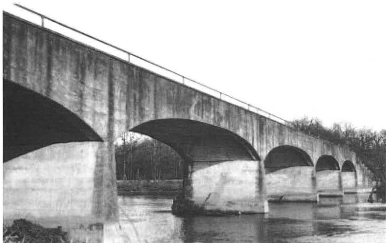
Spring River Bridge, looking east, March 1939.
