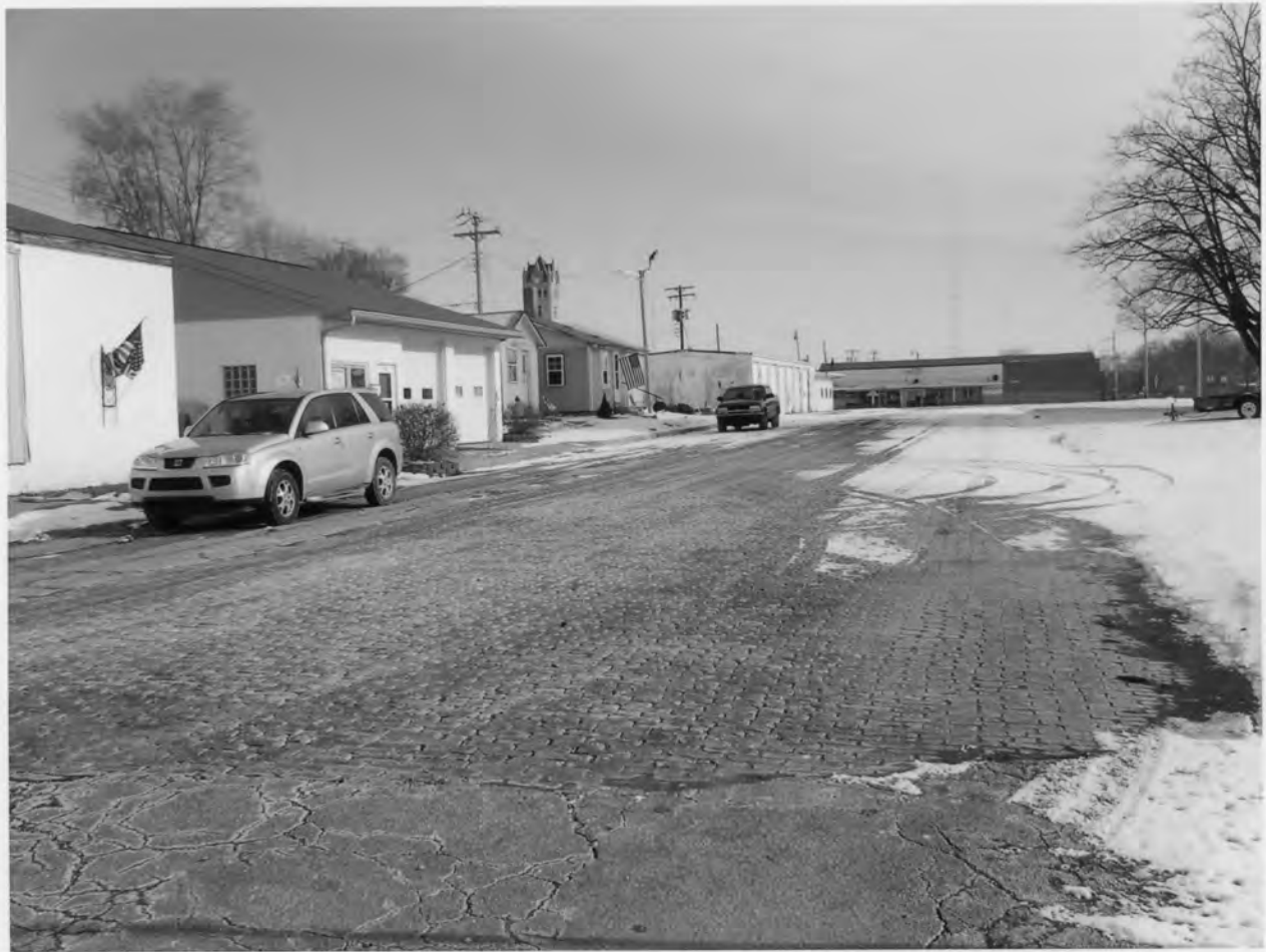
Greenfield Residential Historic District, Hancock Co., IN #0023
