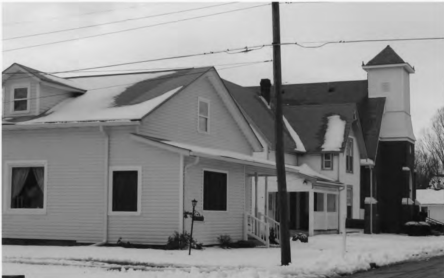
Greenfield Residential Historic District, Hancock Co., IN #0032
