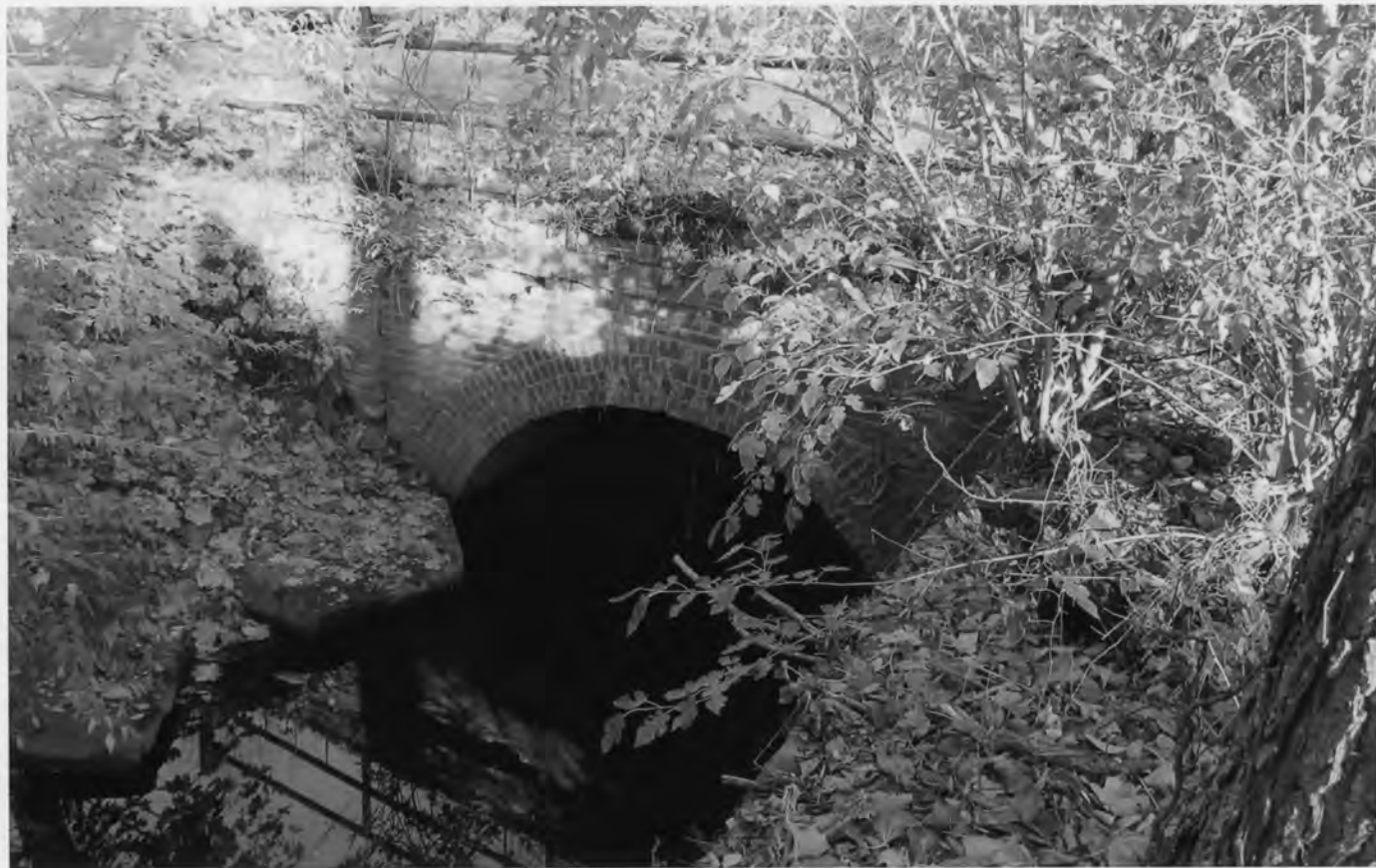
Greenfield Residential Historic District, Hancock Co., IN #0002
