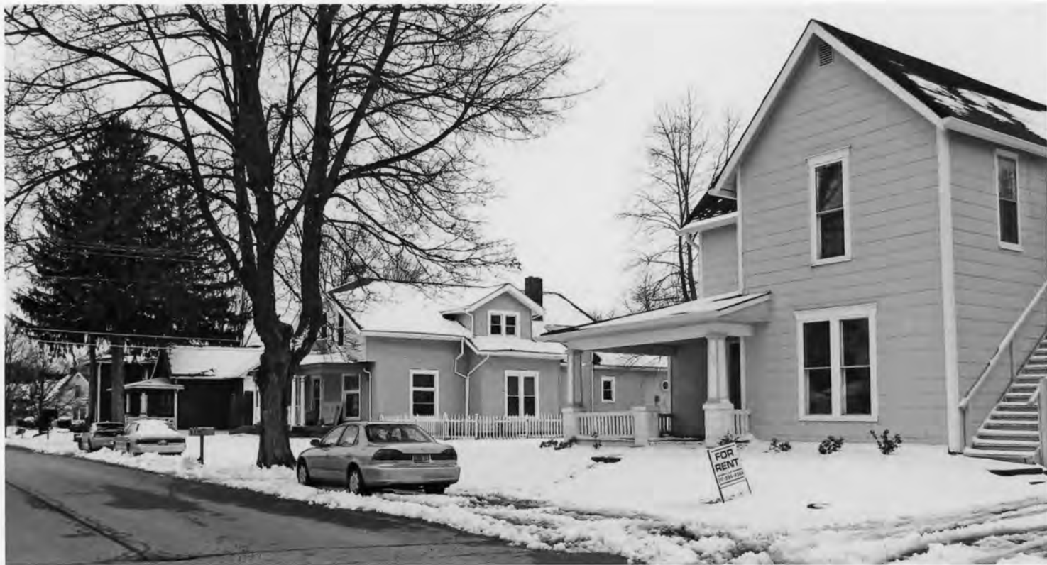
Greenfield Residential Historic District, Hancock Co., IN #00324
