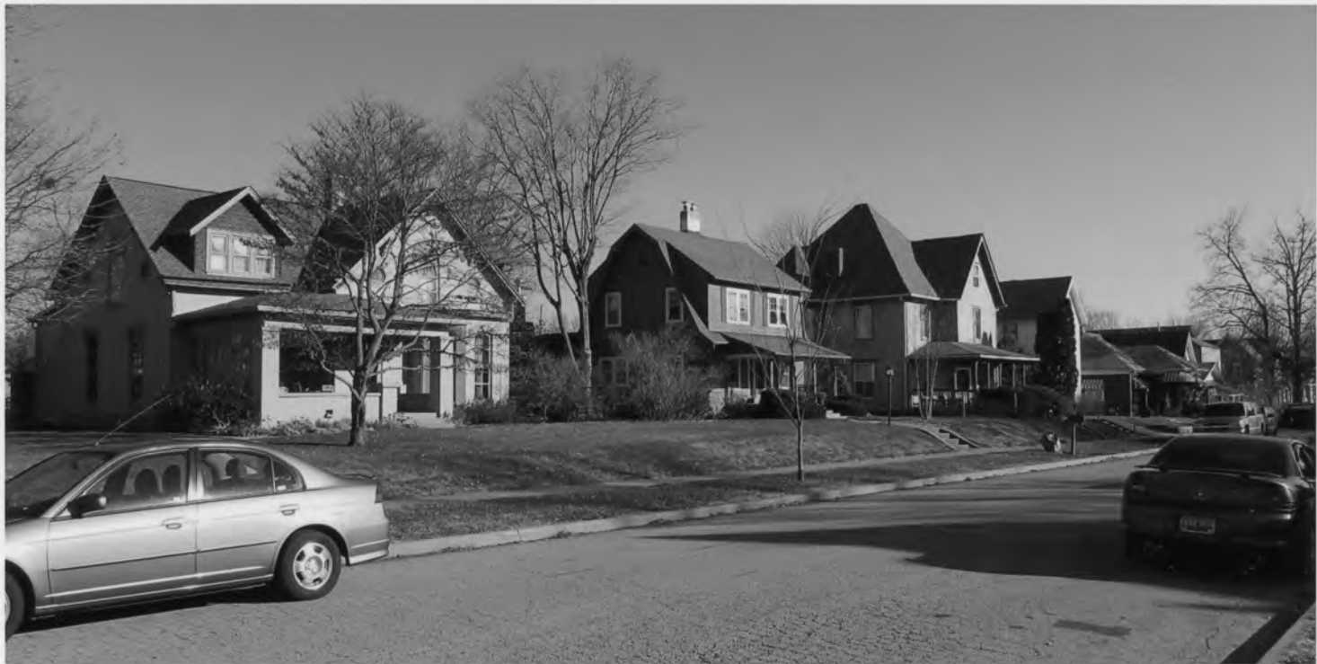
Greenfield Residential Historic District, Hancock Co., IN #0005
