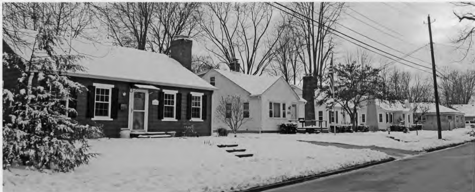
Greenfield Residential Historic District, Hancock Co., IN #0003
