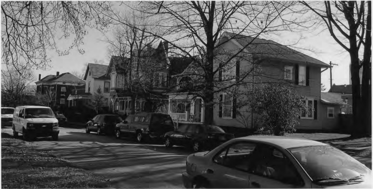
Greenfield Residential Historic District, Hancock Co., IN #0008
