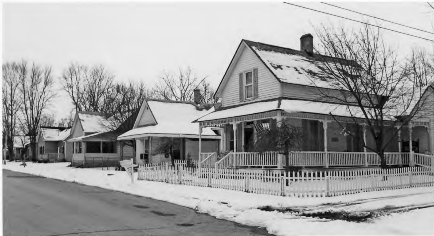
Greenfield Residential Historic District, Hancock Co., IN #0033
