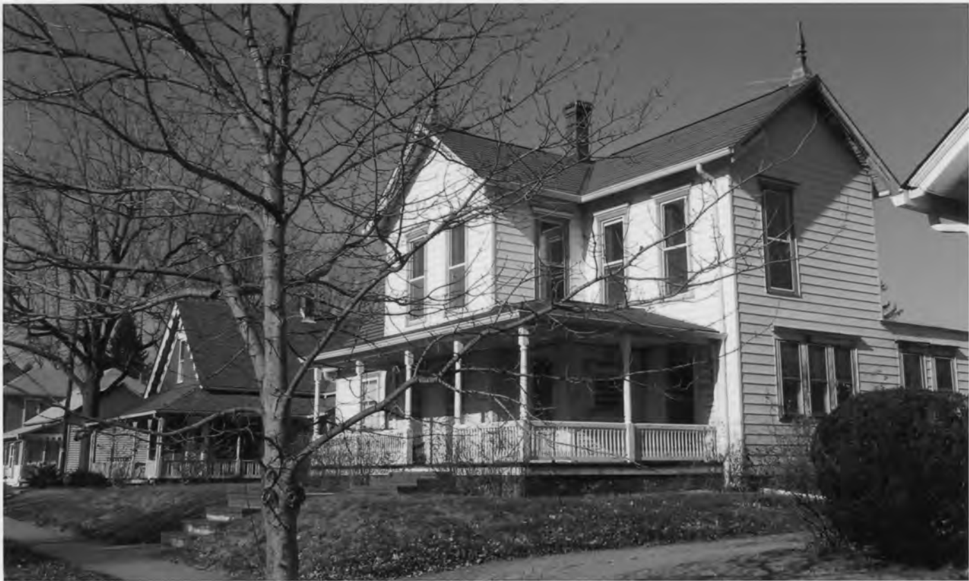
Greenfield Residential Historic District, Hancock Co., IN #0007
