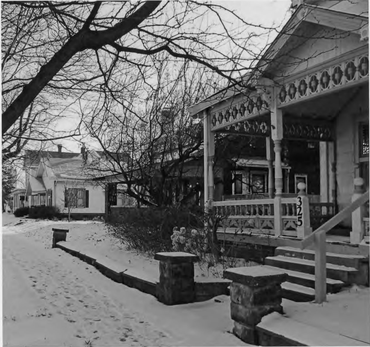
Greenfield Residential Historic District, Hancock Co., IN #0022
