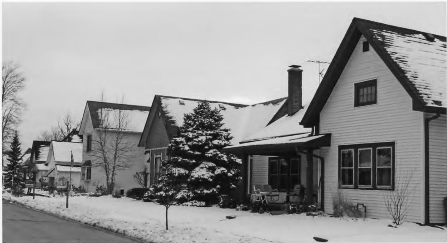
Greenfield Residential Historic District, Hancock Co., IN #0028
