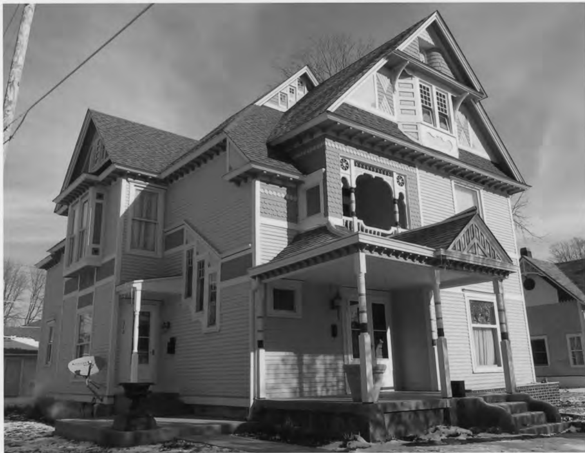
Greenfield Residential Historic District, Hancock Co., IN #0017
