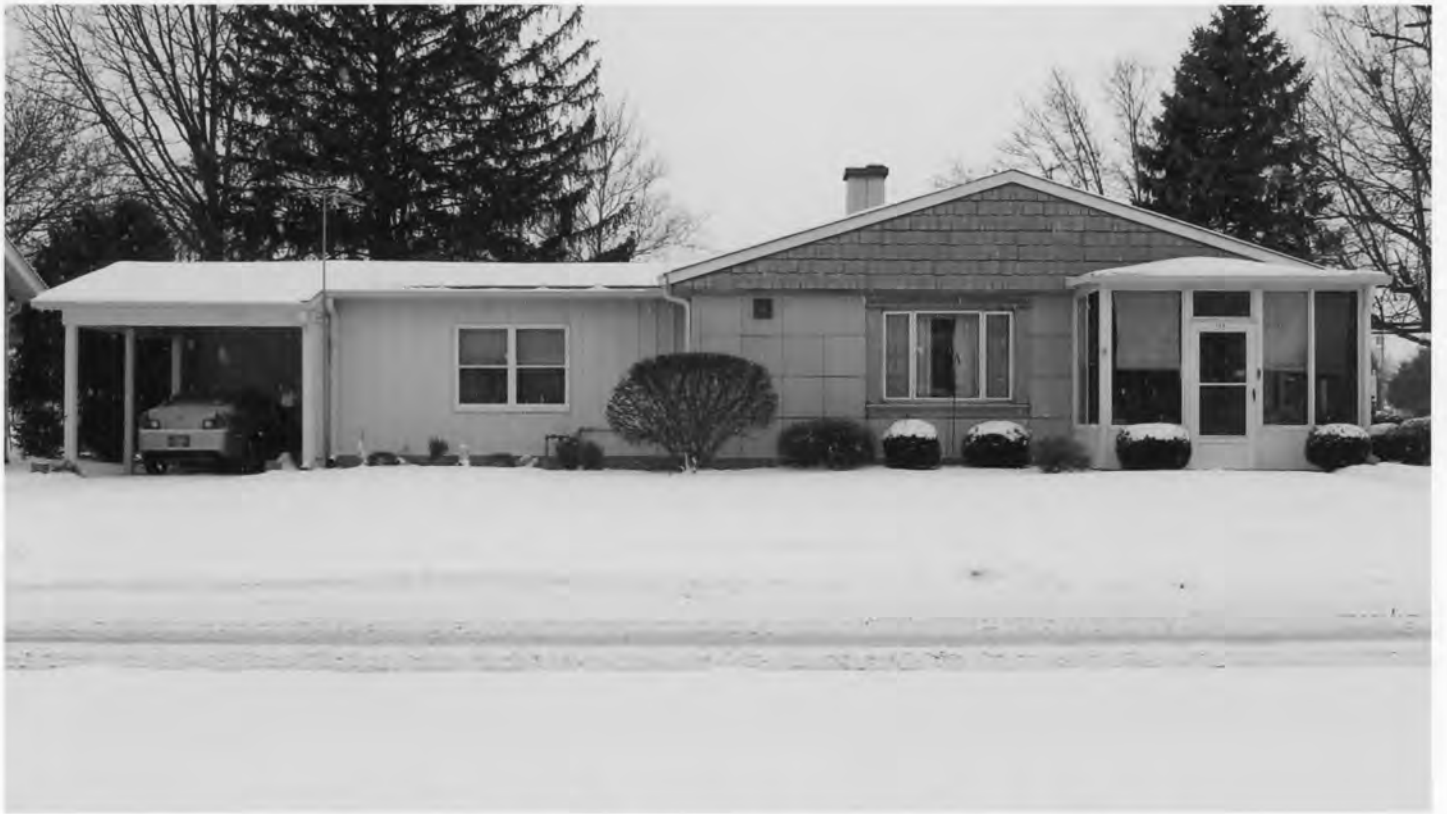
Greenfield Residential Historic District, Hancock Co., IN #0029
