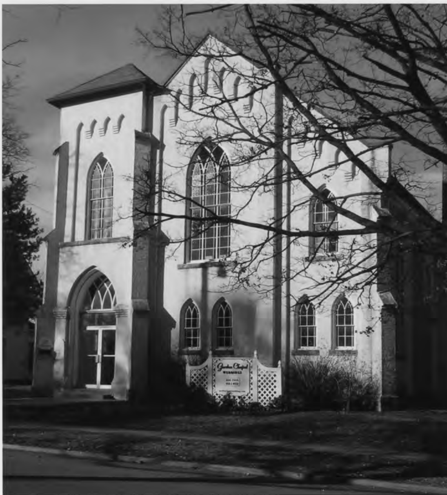
Greenfield Residential Historic District, Hancock Co., IN #0009
