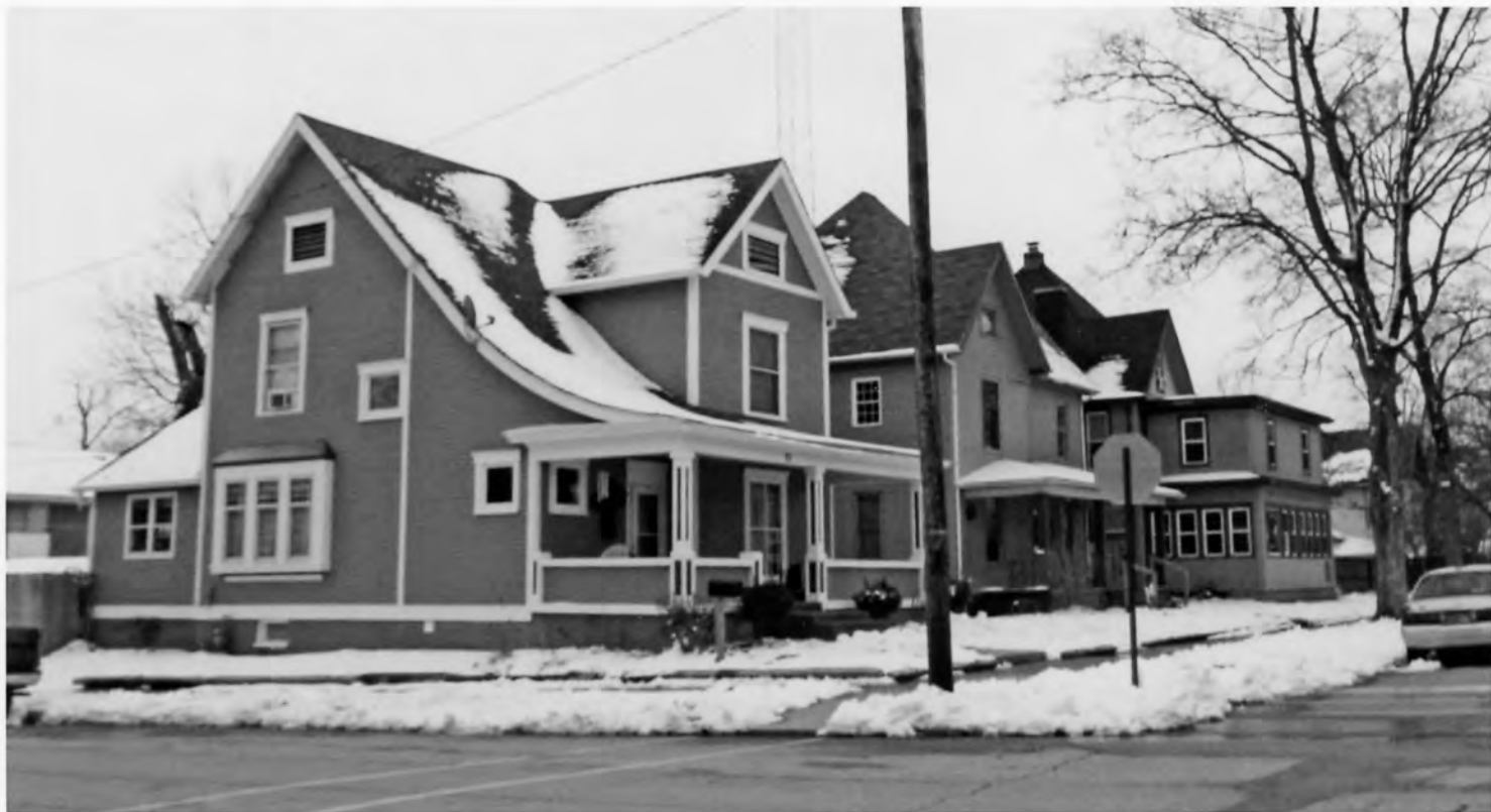
Greenfield Residential Historic District, Hancock Co., IN #0035
