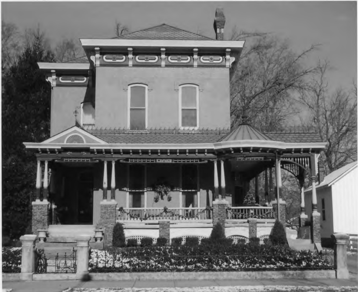
Greenfield Residential Historic District, Hancock Co., IN #0018
