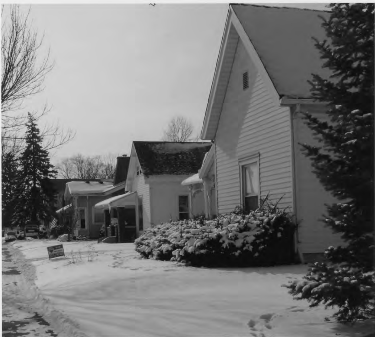
Greenfield Residential Historic District, Hancock Co., IN #0025
