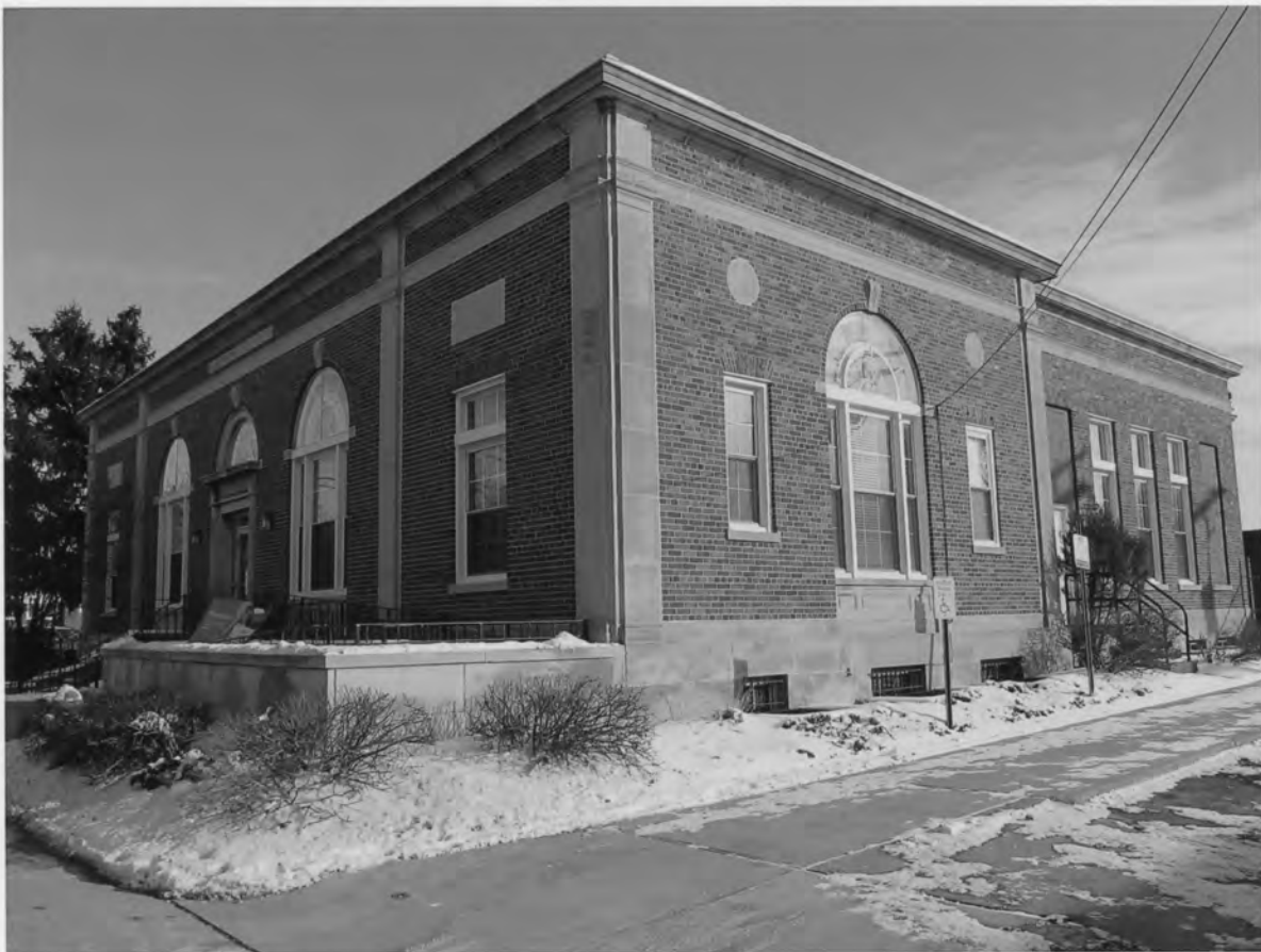
Greenfield Residential Historic District, Hancock Co., IN #0026
