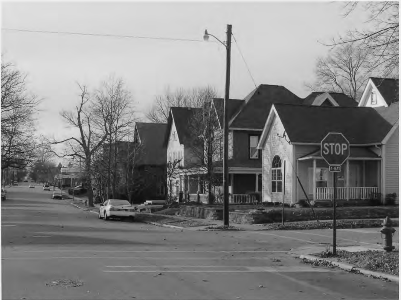
Greenfield Residential Historic District, Hancock Co., IN #0011
