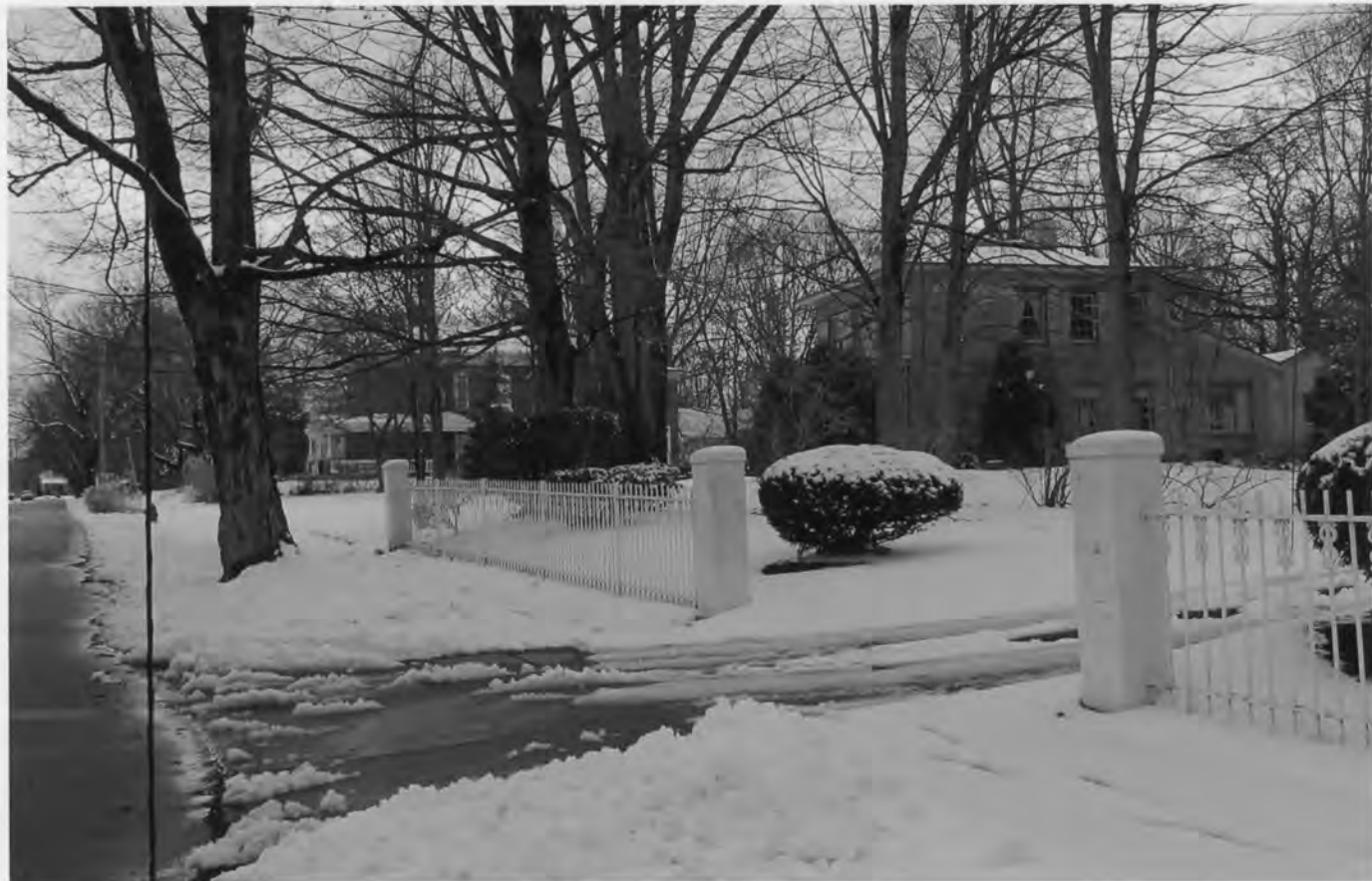
Greenfield Residential Historic District, Hancock Co., IN #0001
