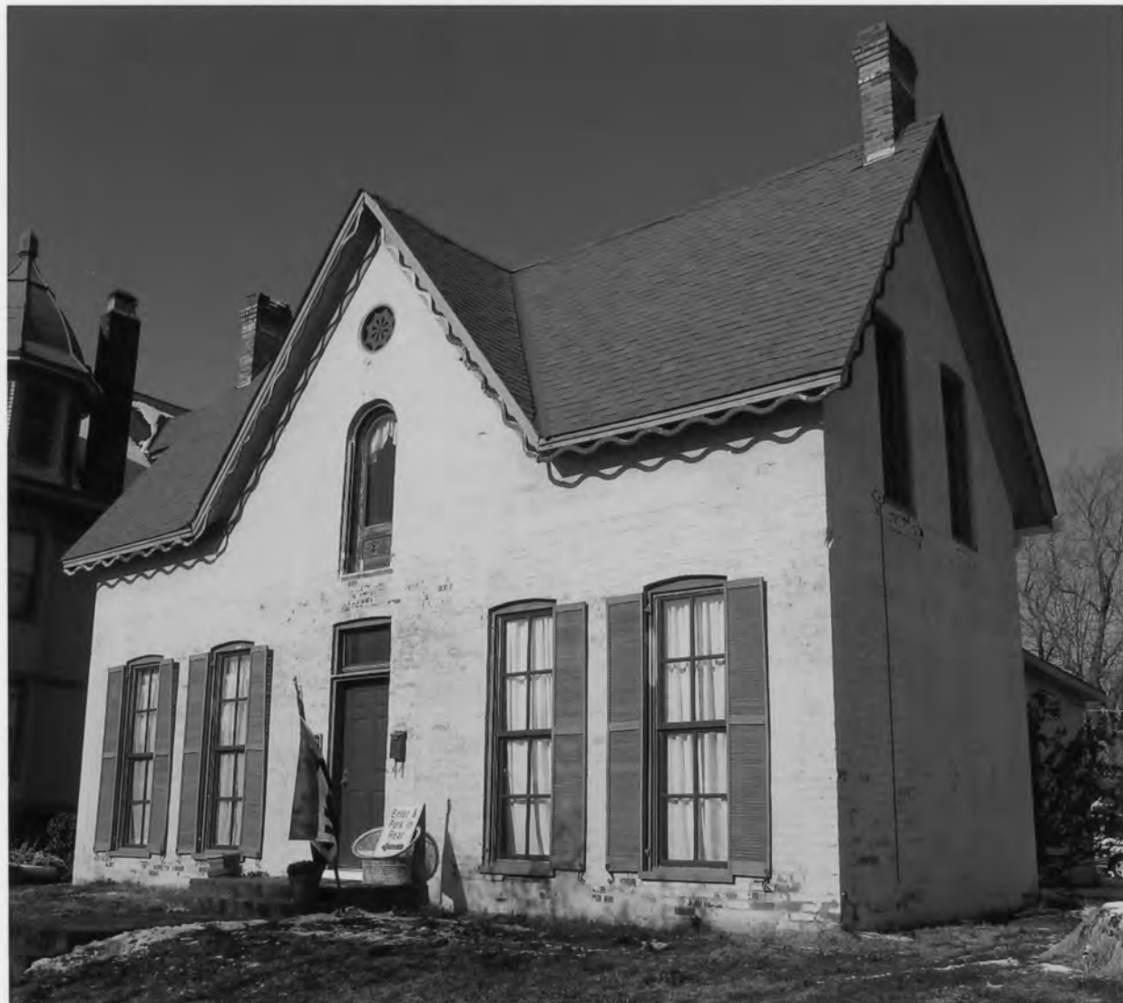
Greenfield Residential Historic District, Hancock Co., IN #0020
