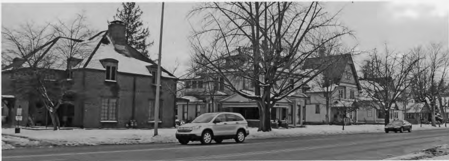
Greenfield Residential Historic District, Hancock Co., IN #0021
