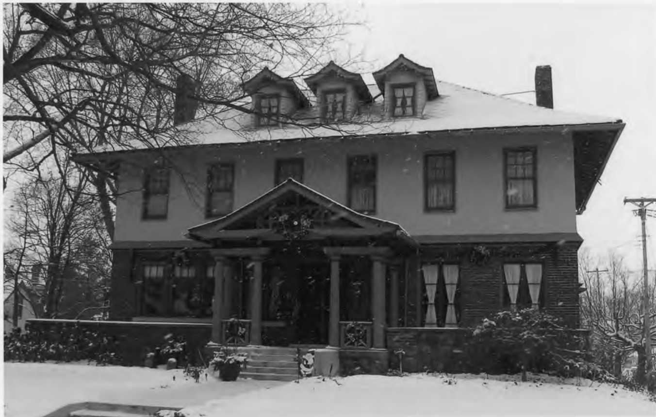
Greenfield Residential Historic District, Hancock Co., IN #0012
