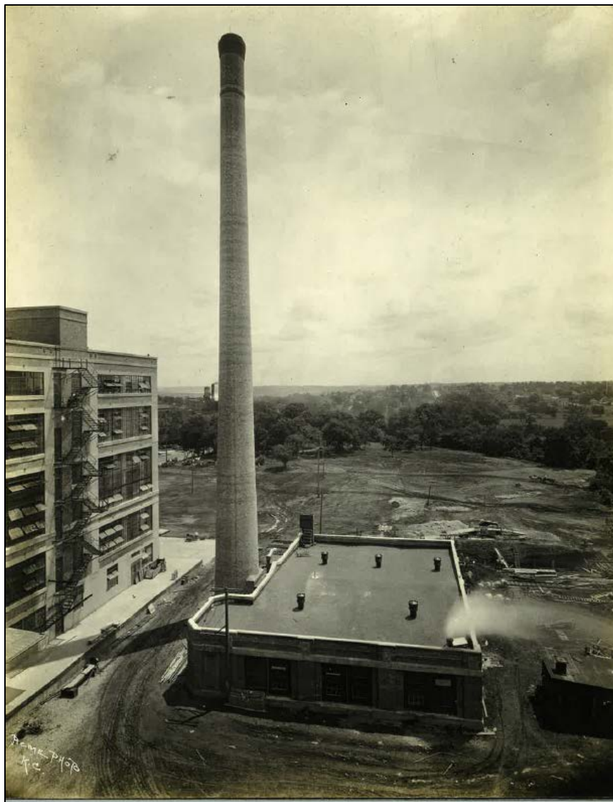
Figure 17: National Cloak & Suit Company Hardesty and Independence Avenues Aerial view of Power House and portion of south façade of Building 'B,' view facing east, c. 1920.
