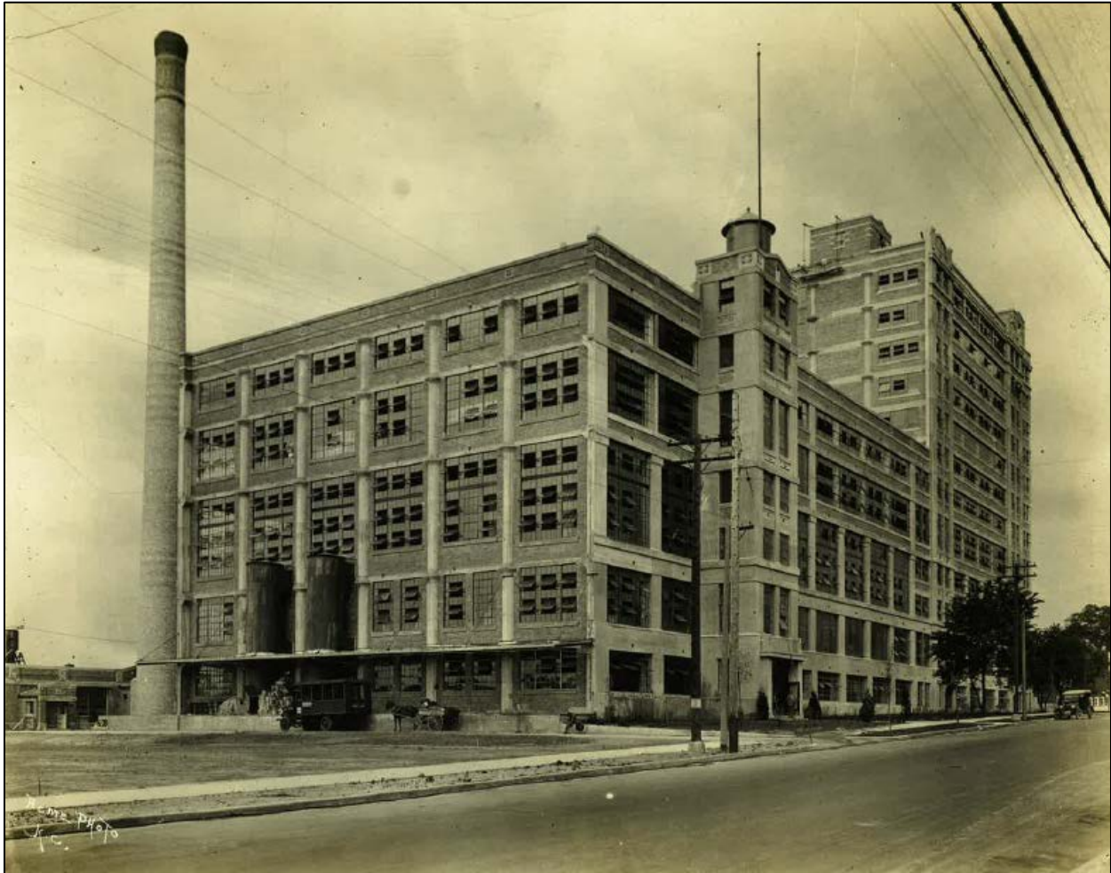
Figure 15: National Cloak & Suit Company Hardesty and Independence Avenues East and north façades and the Power House; view facing southwest, c. 1920
