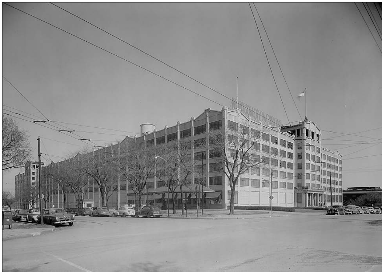
Figure 34: Montgomery Ward Company Building, 6220 St. John Avenue, Kansas City, MO. Frank E. Trask of McKecknie & Trask, architect, 1913-1914 with additions.
