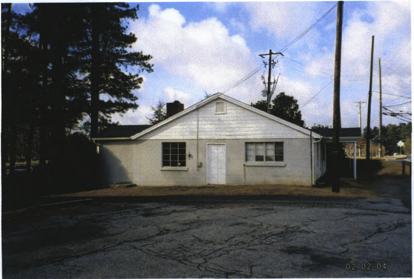
Attachment 2: Newtown Community House Newtown Elementary School, Fulton County, Georgia
