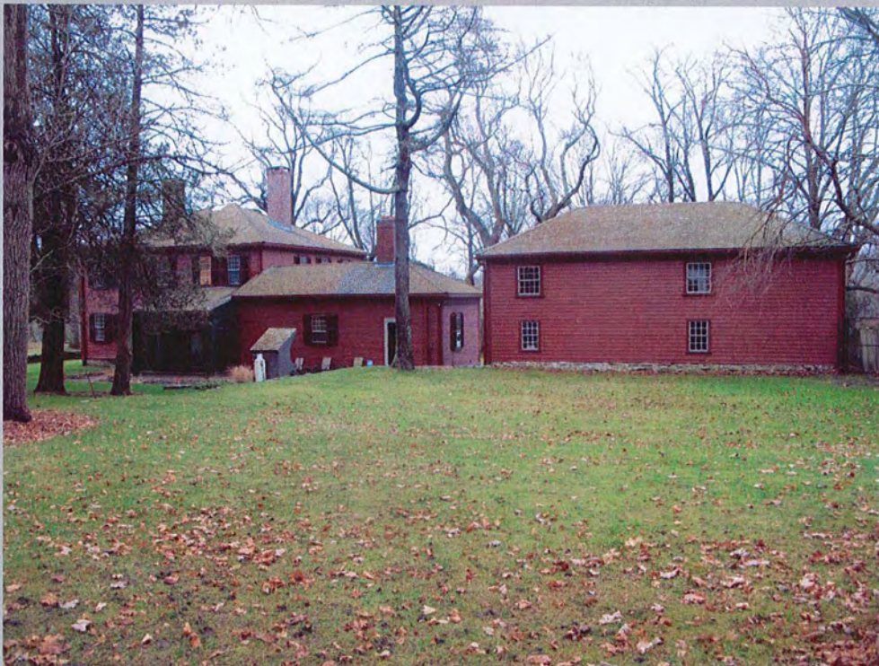
6. Exterior view from northwest, carriage house on right.
