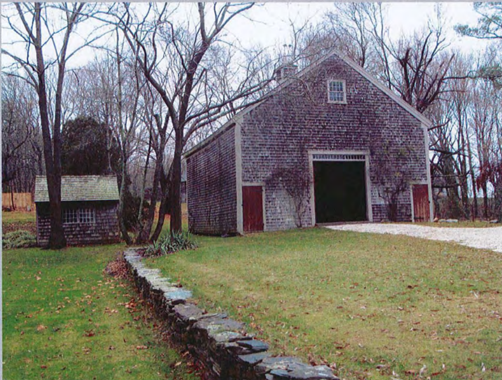
14. Barn exterior from southwest, garden shed on left.
