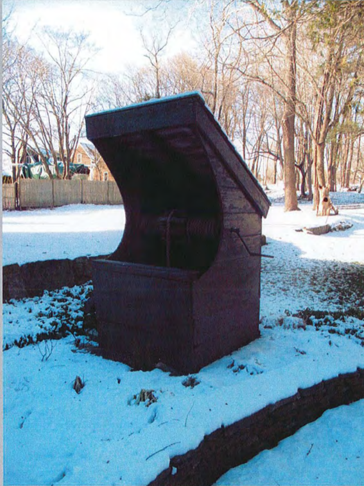
17. Well house from southeast.
