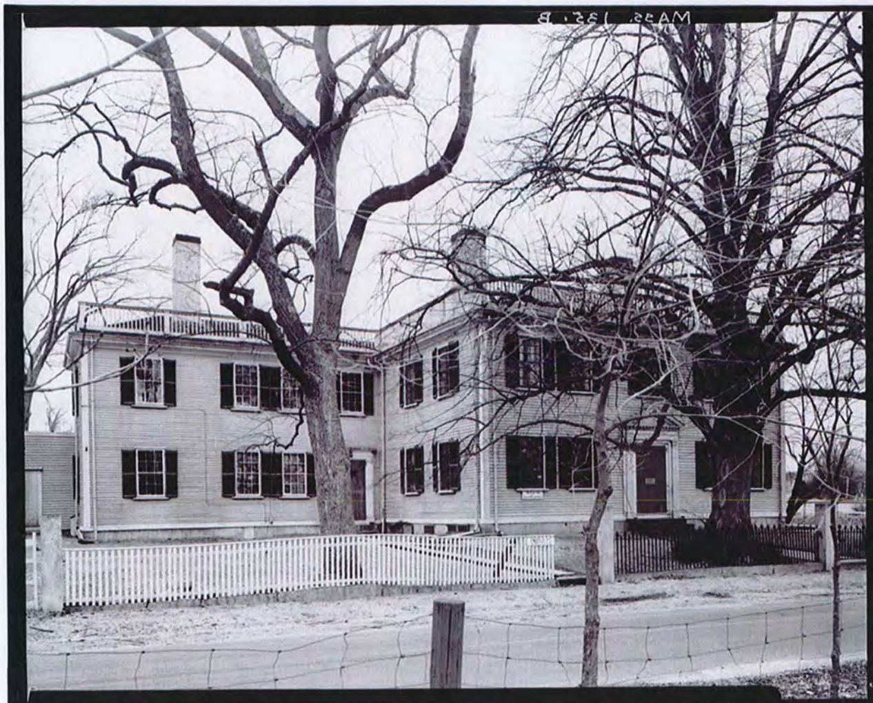
Fig.2: Exterior view from SW, Arthur C. Haskell, photographer, Historic American Buildings Survey (HABS), 1936..
