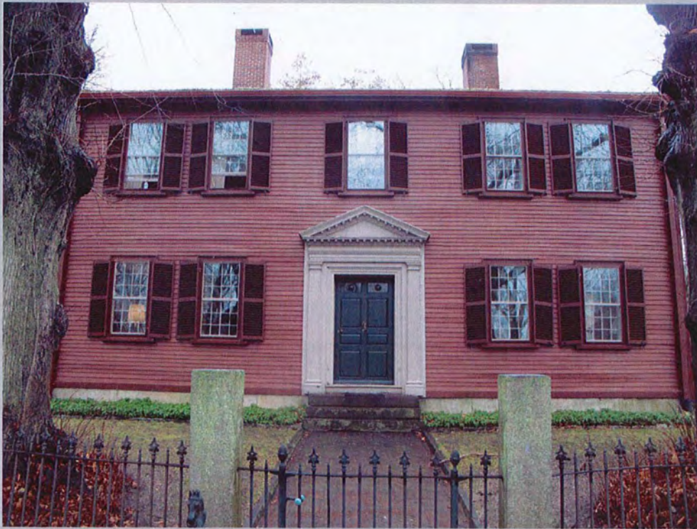
3. Detail of front façade from south.
