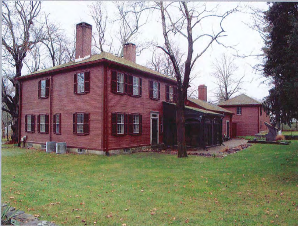
5. Exterior view from northeast.
