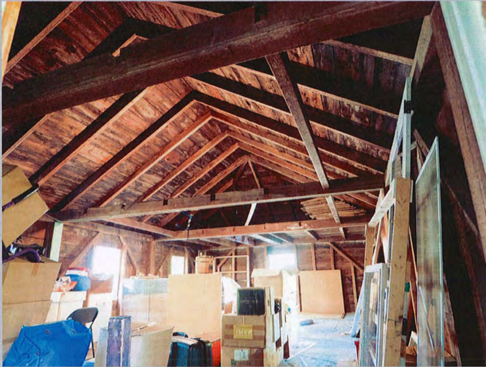
13. Carriage house interior, upper story.
