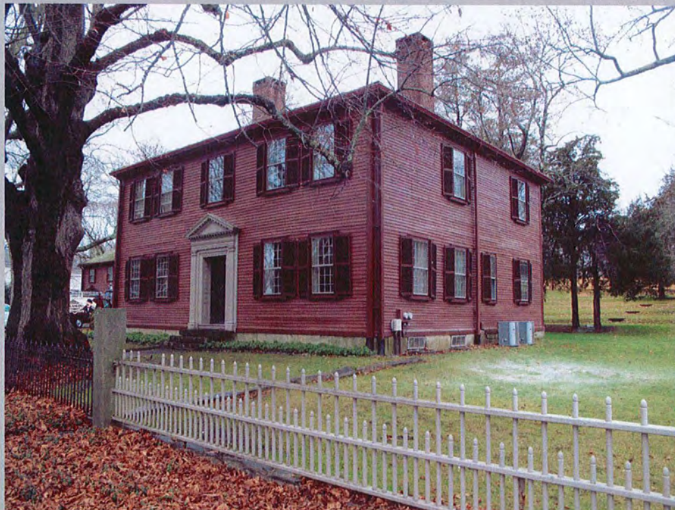
4. Exterior view from southeast.
