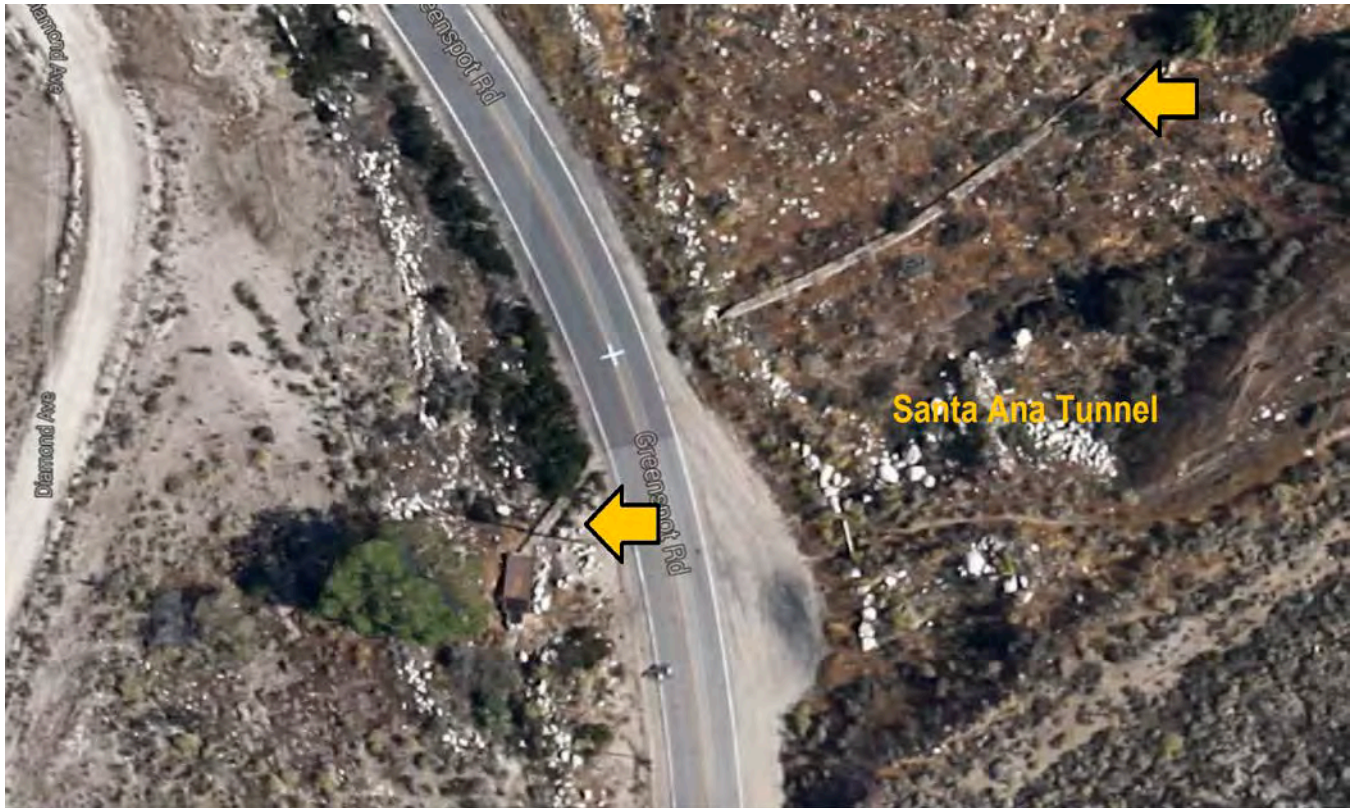
Figure 7. Aerial View, Yellow arrows indicate Santa Ana Tunnel crossing Greenspot Road
