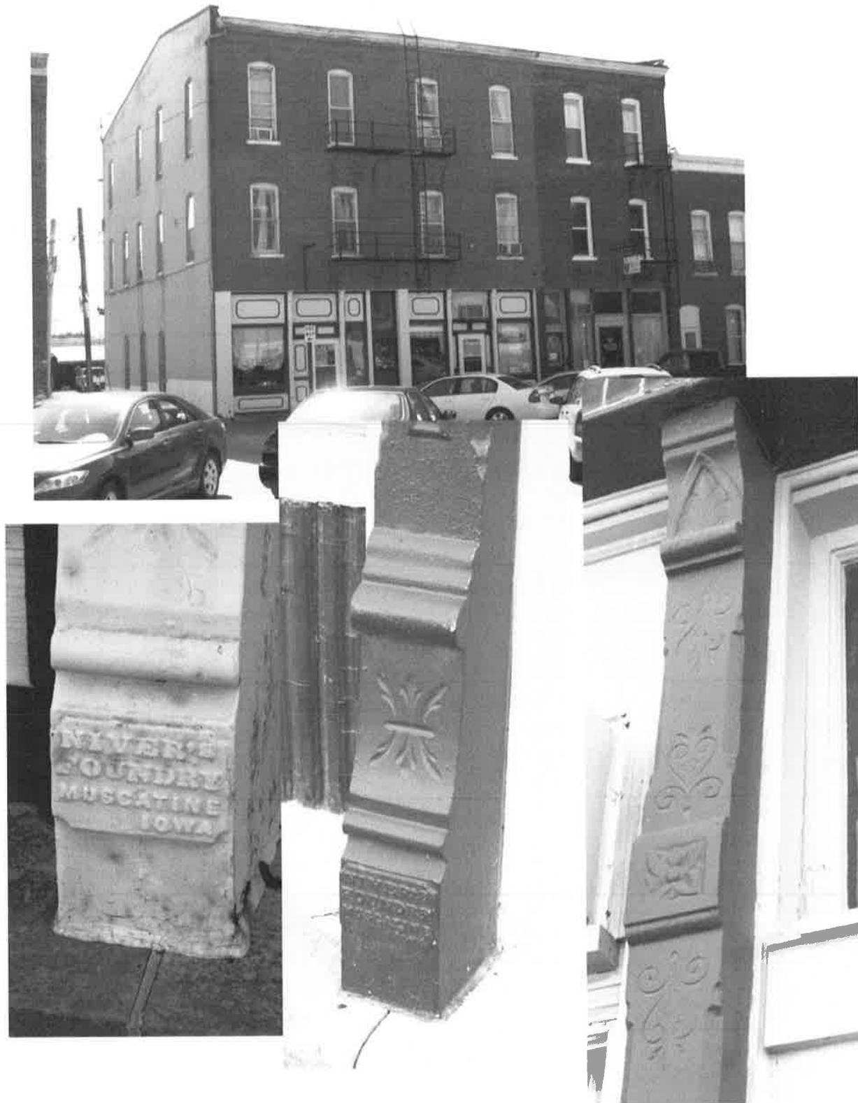
**Figure 19. Kerchner Block built in 1892, detail of storefront columns from Niver's Foundry (Map #5) (McCarley 2011).**
