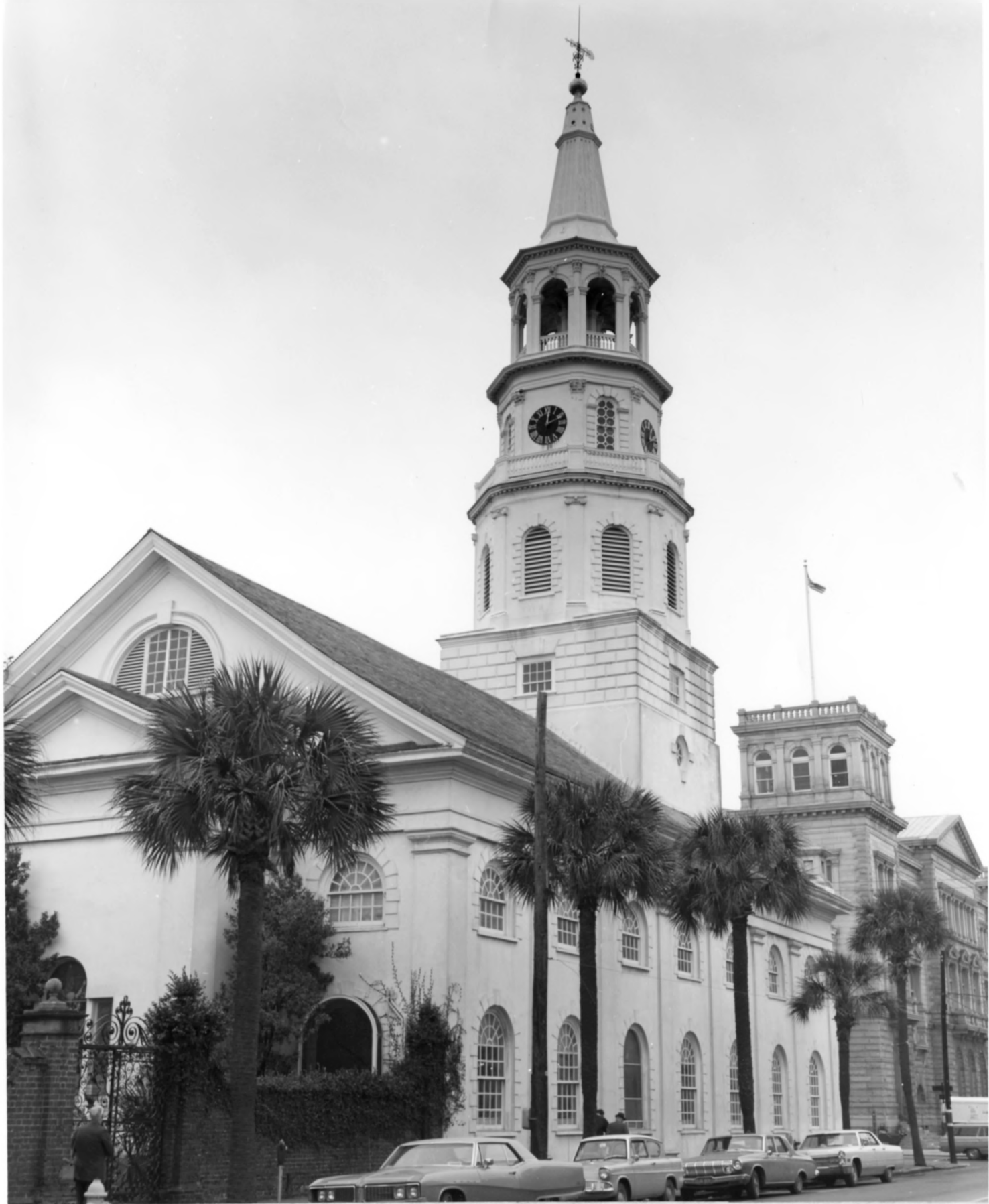
St. Michael's Church, Charleston, South Carolina
