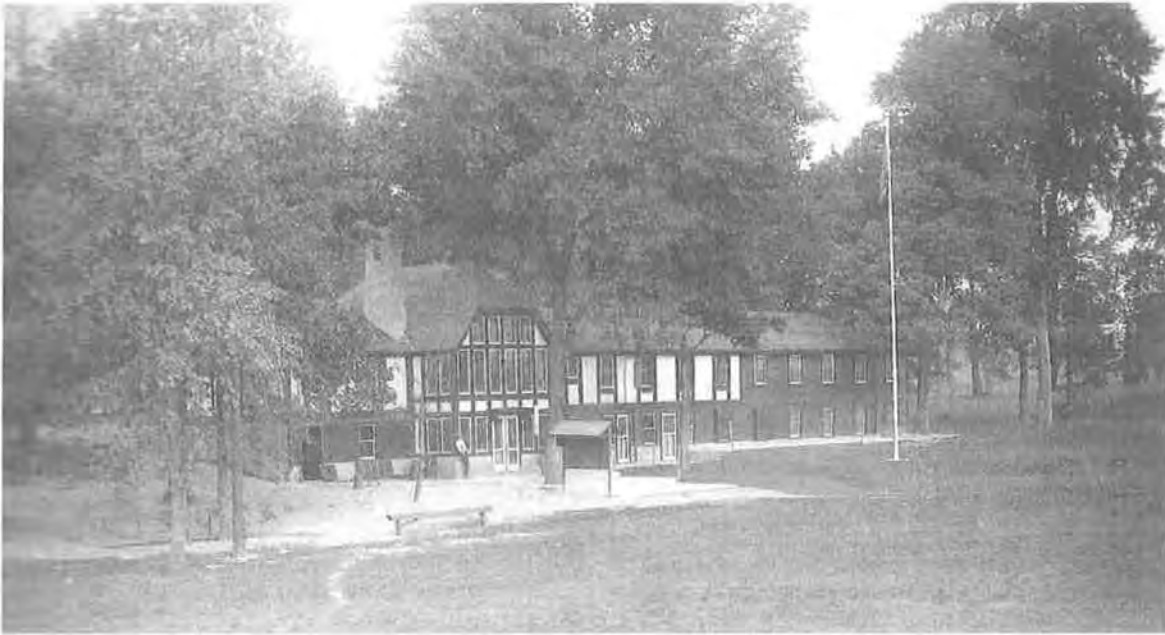
Figure #16 Image of the Olmsted Brothers designed clubhouse c. 1923. Location Art Work of Dayton, Ohio , Gravure Illustration Co.
