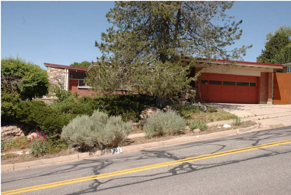
Photograph 1 East elevation of house. Camera facing west.
