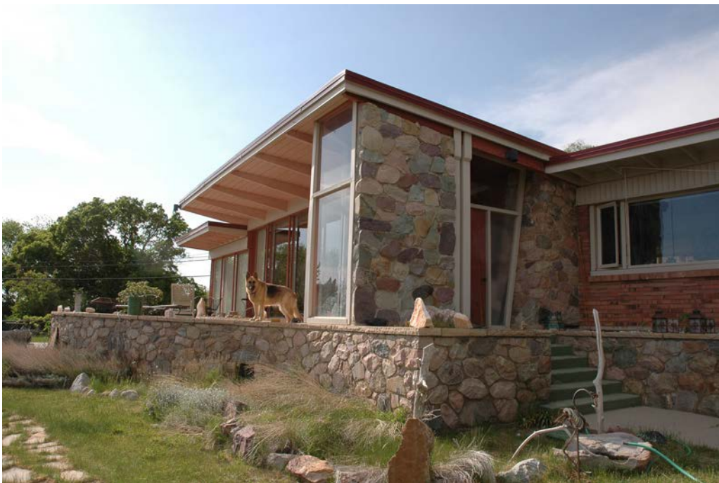
Photograph 4 South and east elevations of house and patio. Camera facing northwest.
