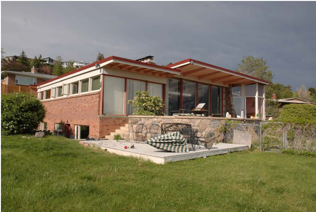
Photograph 5 South and west elevations of house. Camera facing northeast.
