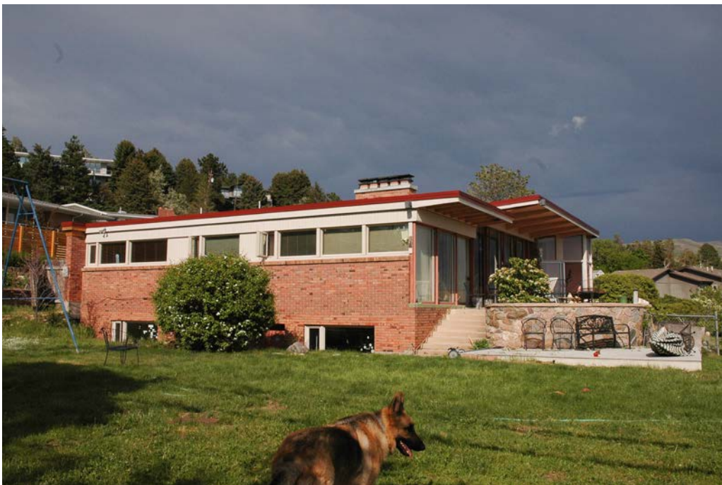
Photograph 6 West elevation of house. Camera facing east.
