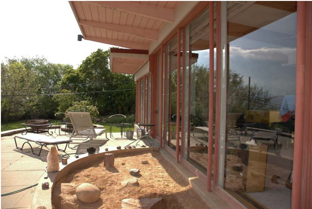
Photograph 9 South elevation of house, patio and planter detail. Camera facing west.
