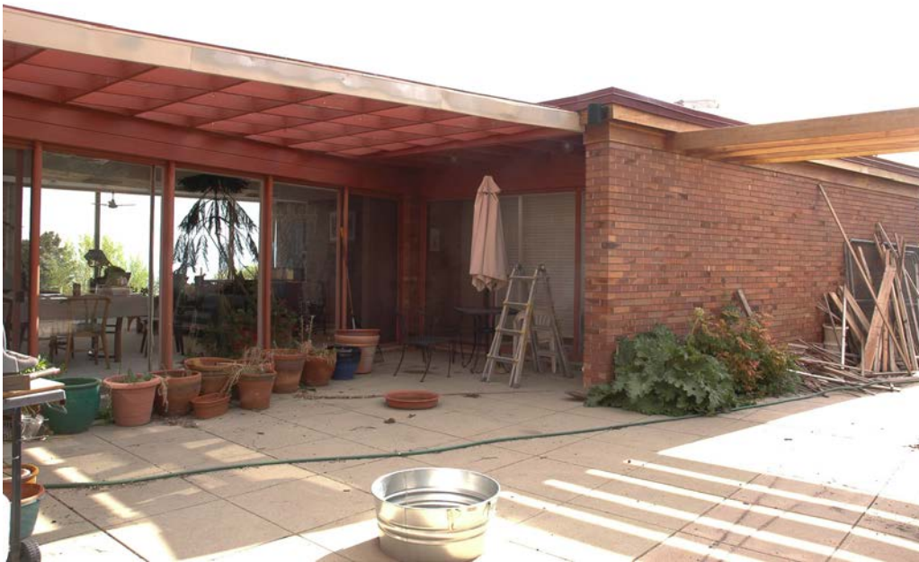
Photograph 8 North elevation of house and patio. Camera facing southwest.
