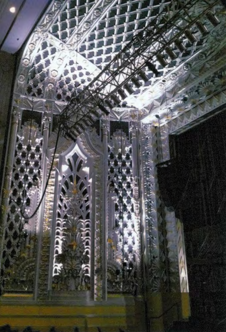
CA_Los Angeles County_Fox Wilshire Theatre_ 0013
