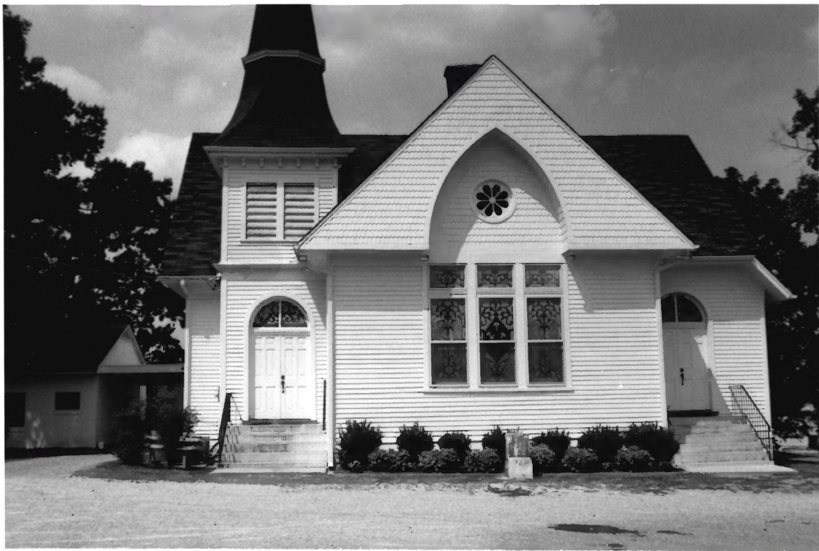
Asbury Methodist Episcopal Church, South Knox Co. TN 1 of 18
