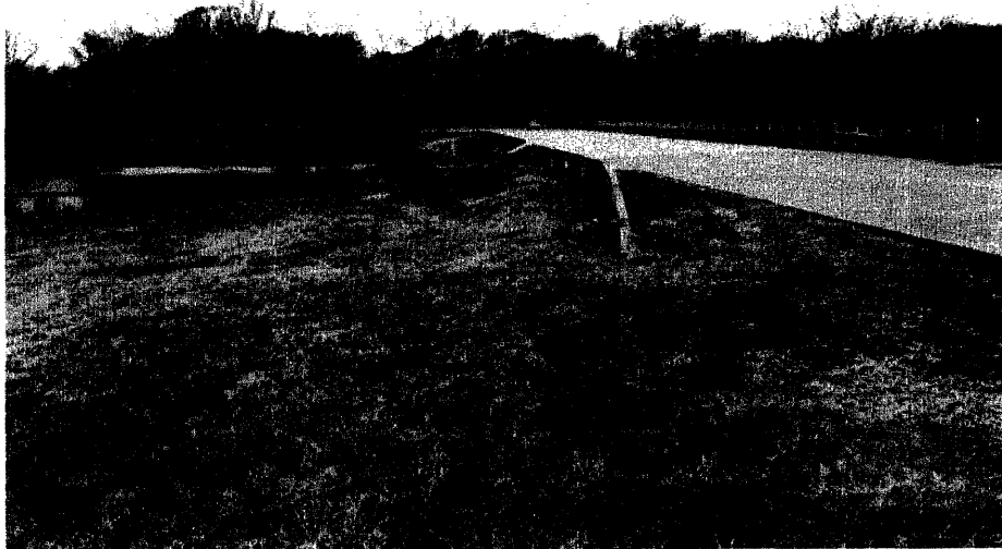
Contemporary view of Felgates Creek (1996). Note no trees or plantings at bridge abutments. LANDSCAPES.
