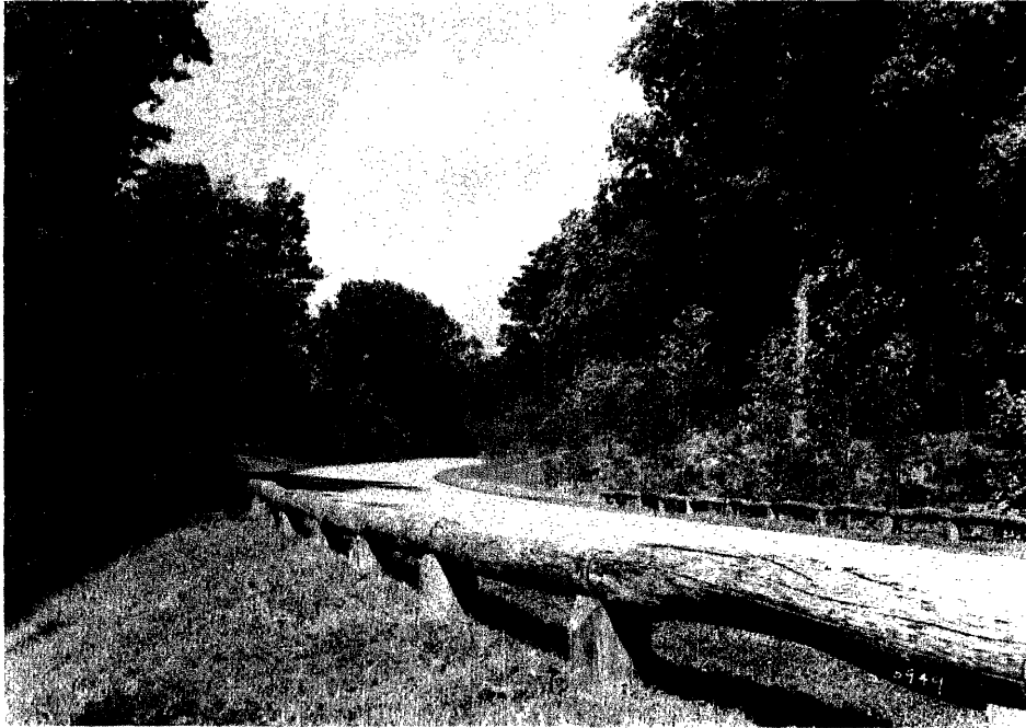
Historic view of 1930s peeled-log guard rail (c.1938). National Park Service, Colonial National Historical Park.
