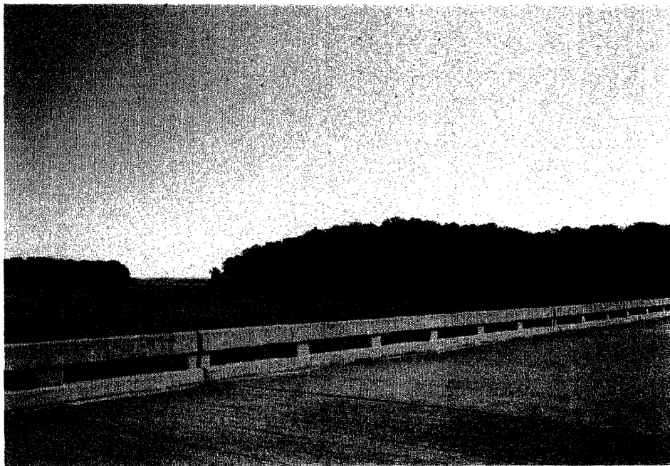
Contemporary view of 1980s bridge railing detail which replaced the historic railing seen above (1996). LANDSCAPES.
