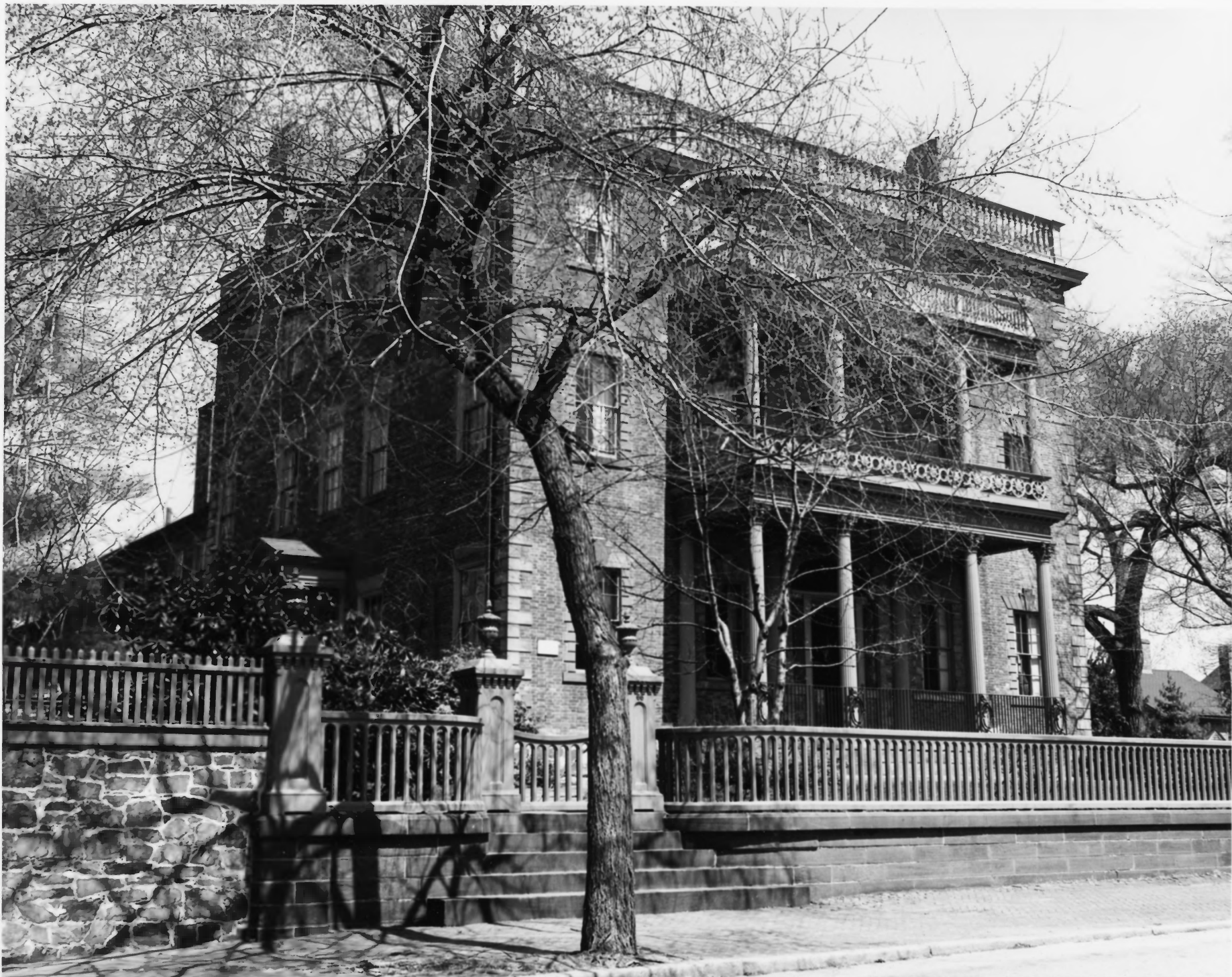
Edward Carrington House, Providence, Rhode Island
