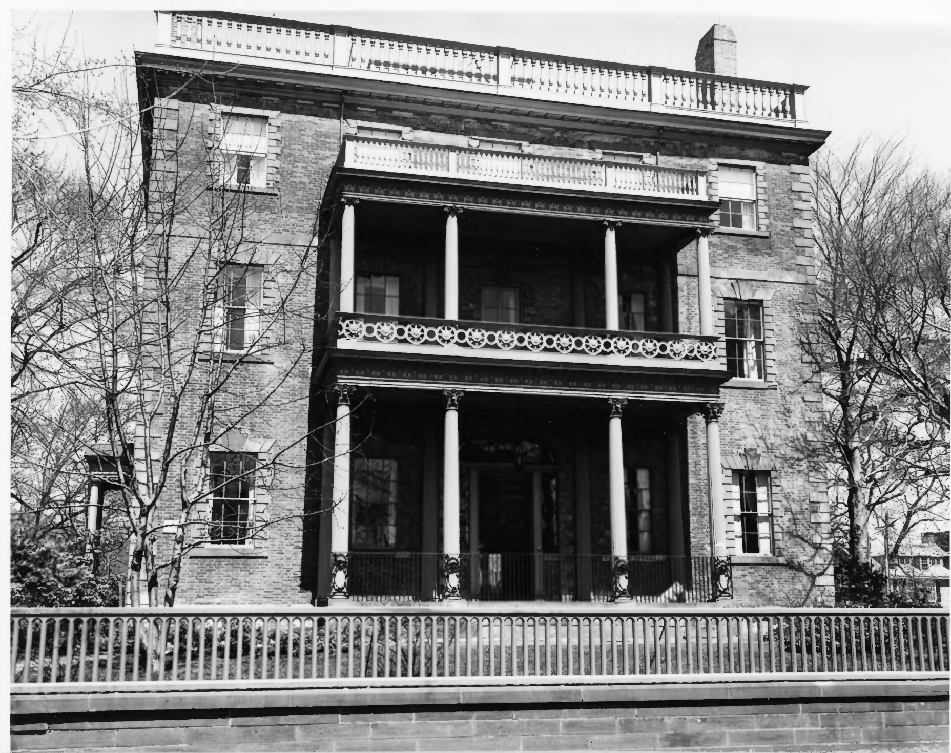
Edward Carrington House, Providence, Rhode Island
