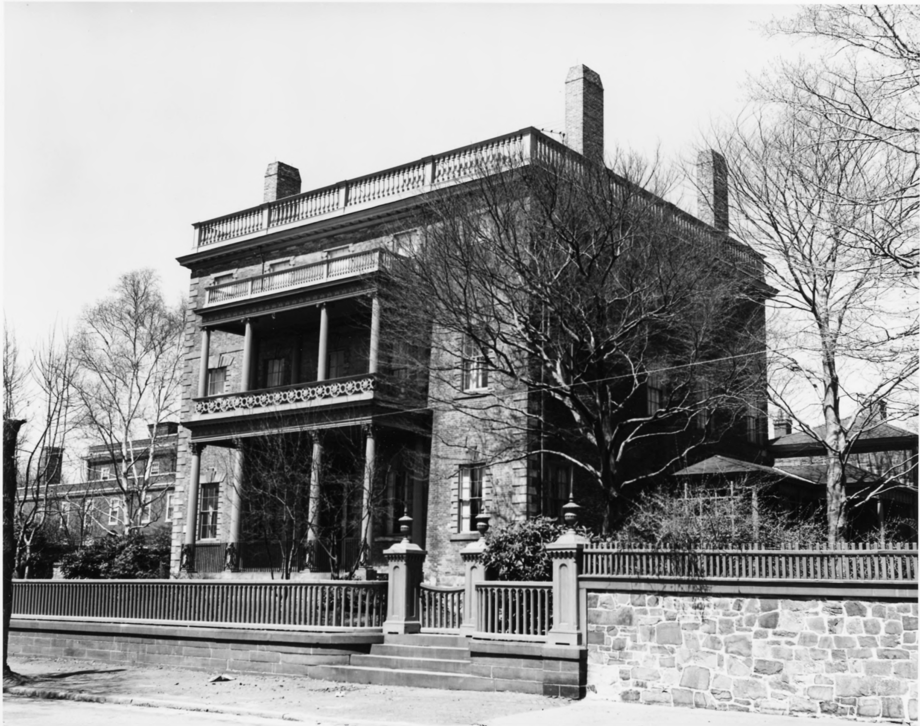
Edward Carrington House, Providence, Rhode Island
