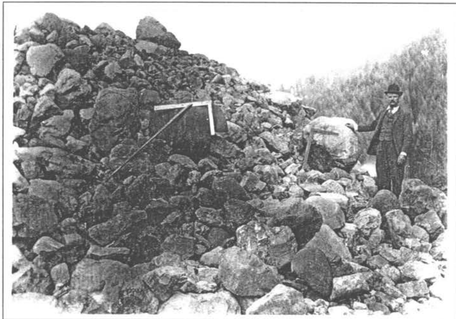
Plate 24. Bill Ruble with 2-foot measure showing the size of boulder that could be stacked with the Ruble Rock Elevator. Used with permission, McLane.
