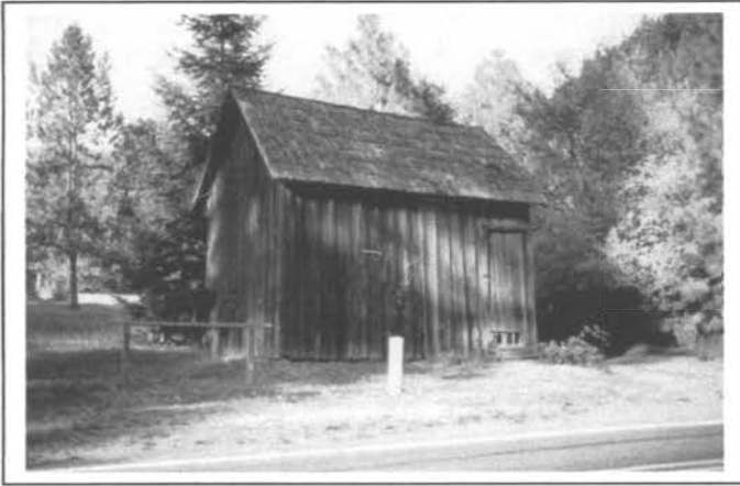
Plate 9. Grain bin looking north.
