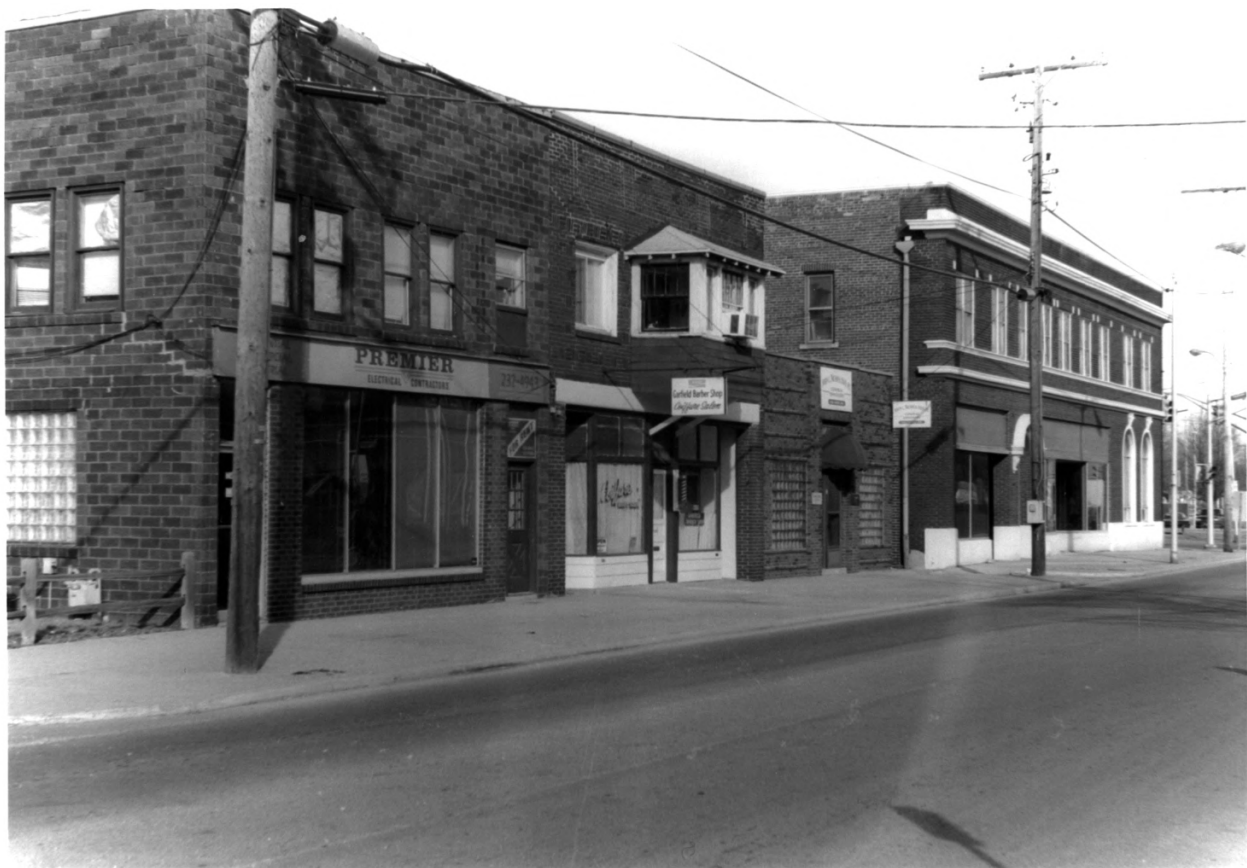
1240, 1242-1244, 1250-1256 MAPLE AVE 12 PTS. H.D., VICO Co., IN PHOTO No. 1
