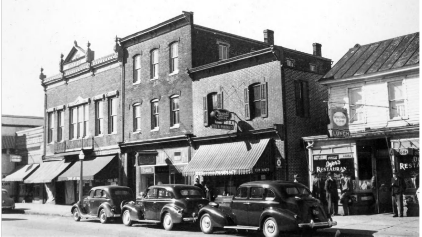
Figure 17: View of the west side of Commerce Street near the intersection with Clark Street, 1947 (Courtesy of the Hagley Digital Archives).
