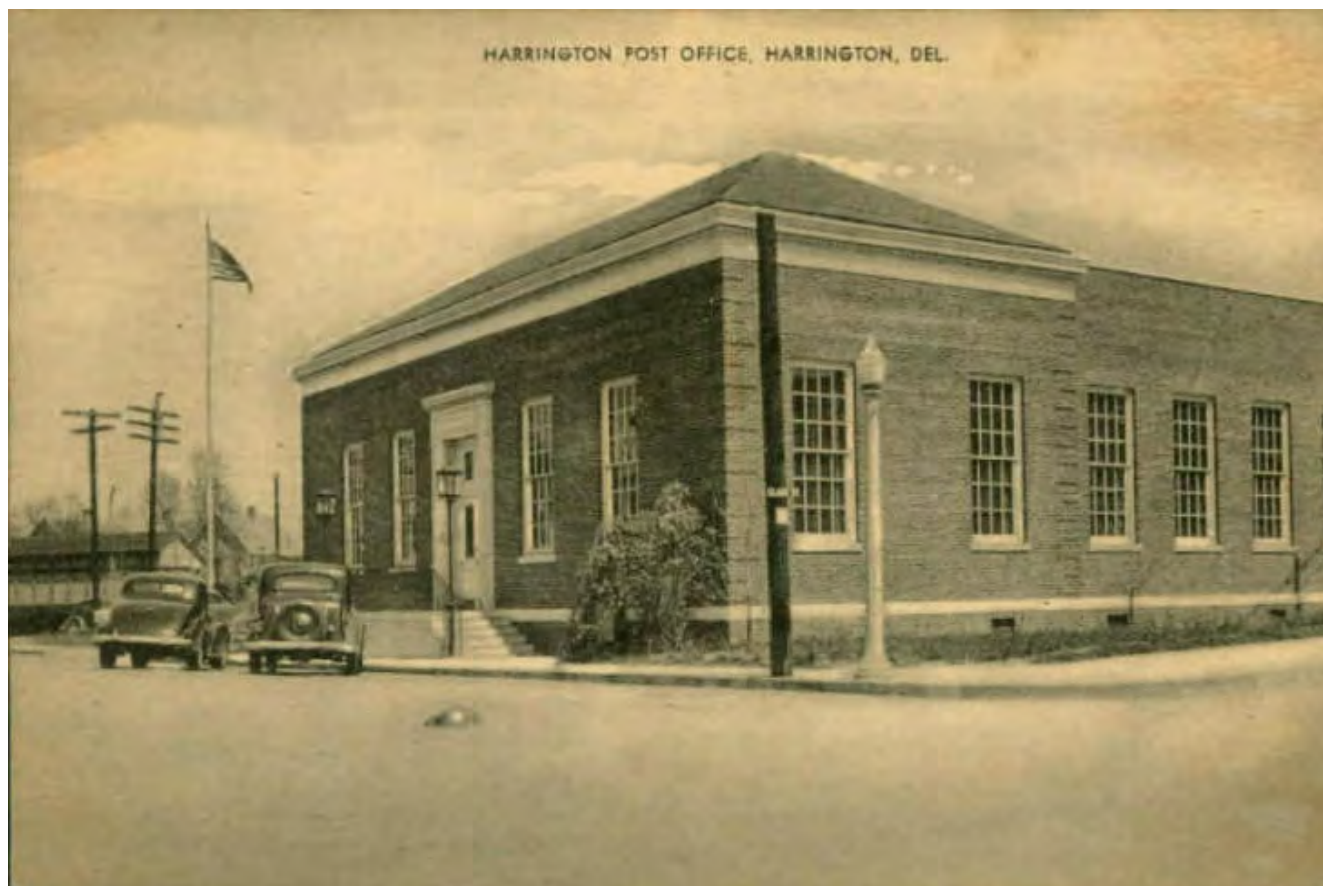
Figure 19: Harrington Post Office at 2 Commerce Street, c. 1940 (Courtesy of the Delaware Public Archives).
