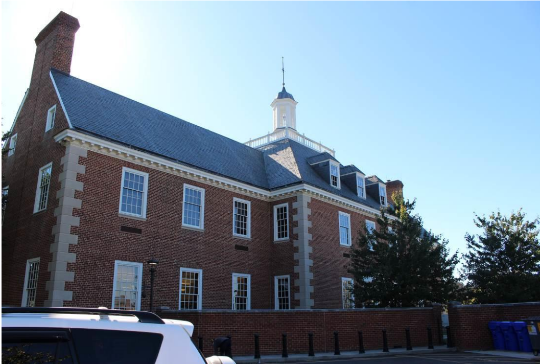
Photo 6: DC_Petworth Neighborhood Library _0006.tif West (rear) elevation of Central Block_Looking Southeast
