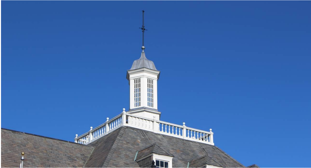
Photo 4: DC_Petworth Neighborhood Library_0004.tif Cupola, Looking Northwest
