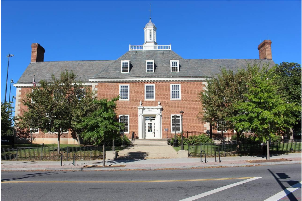
Photo 2: DC_Petworth Neighborhood Library, _0002.tif East Elevation, Looking Northwest
