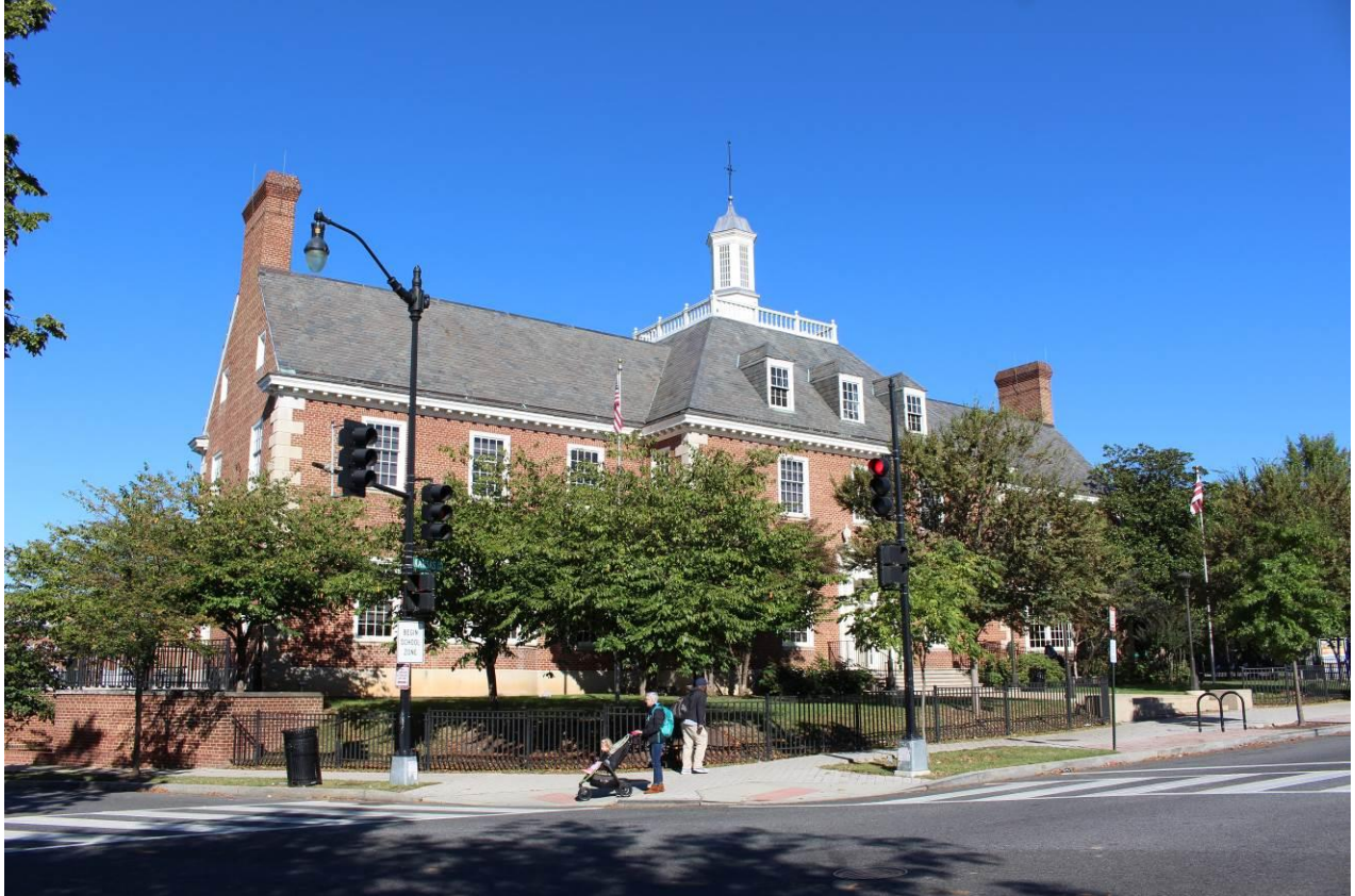
Photo 1: DC_Petworth Neighborhood Library_0001.tif East and South Elevations, Looking Northwest
