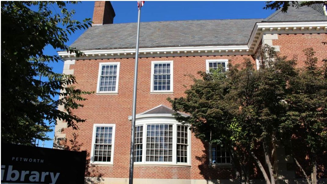
Photo 9: DC_ Petworth Neighborhood Library_0009.tif South Wing East Elevation, Looking Northwest
