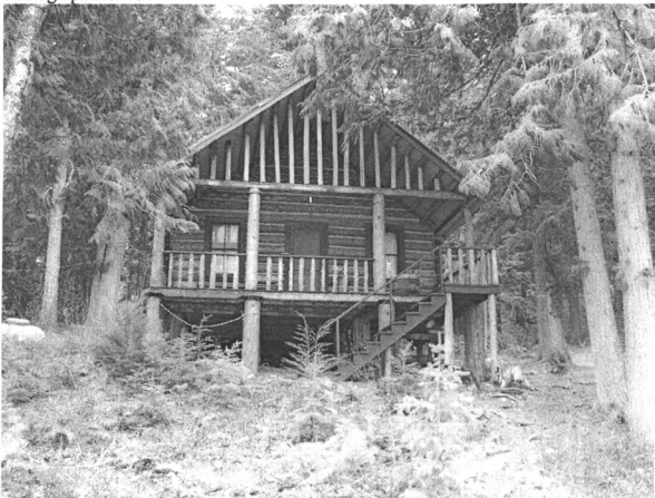
Cabin 2 View of east (front) side of Cabin 2 Photograph No. 17
