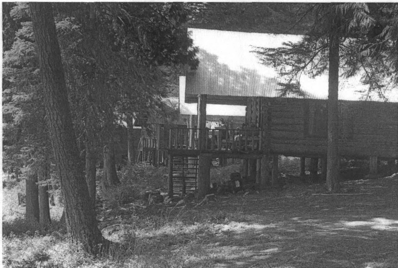
Cabins 1, 2, 3 and 4 (front to back), Kelly's Camp Historic District Glacier National Park, Flathead County, Montana Photograph No.7
