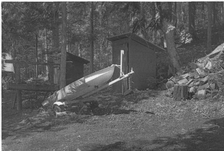
Privies behind Cabin 1, Kelly's Camp Historic District Glacier National Park, Flathead County, Montana Photograph No. 15
