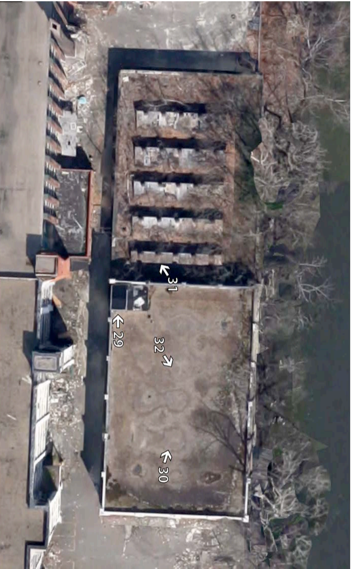
Interior – Building 4, First and Second Floors.
