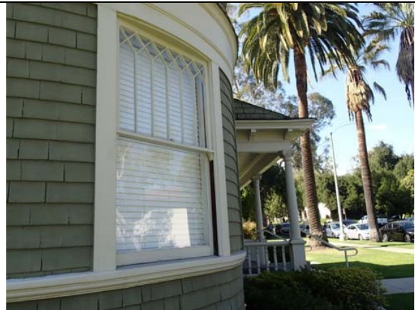
Detail of turret window at southeast corner.
