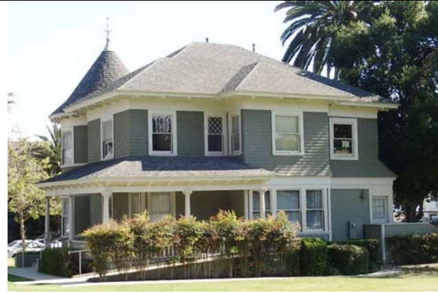
View southwest of north façade.
