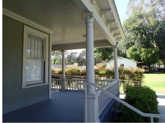
View north of front porch columns and railing.
