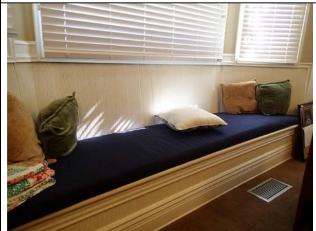
Detail of built-in bench in dining room.
