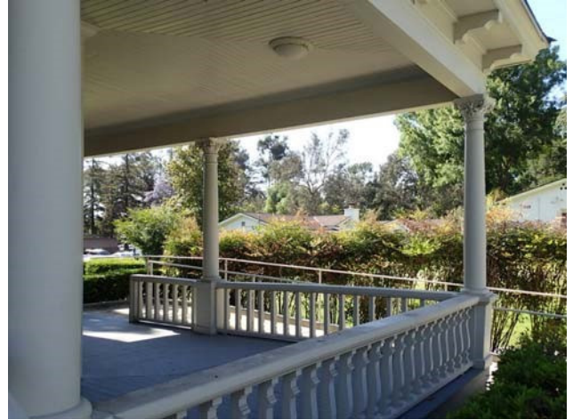
View northwest of porch railing.
