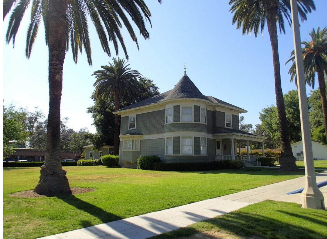
Renwick House, view northwest from corner of College Ave. and Second St. Land in foreground is a part of the original extent of the property.
