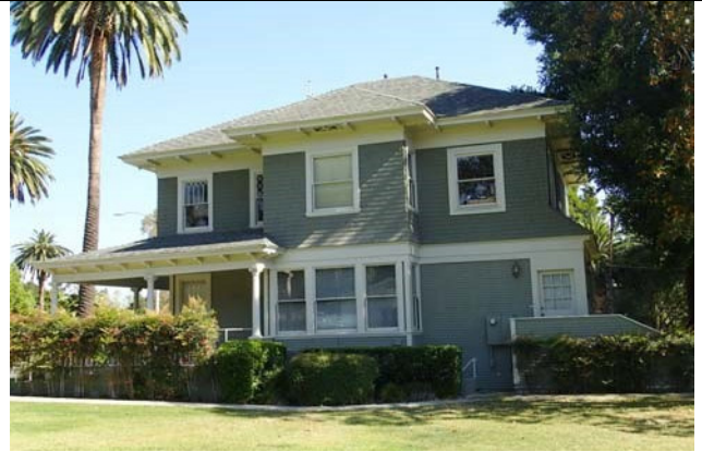
View south of north façade.
