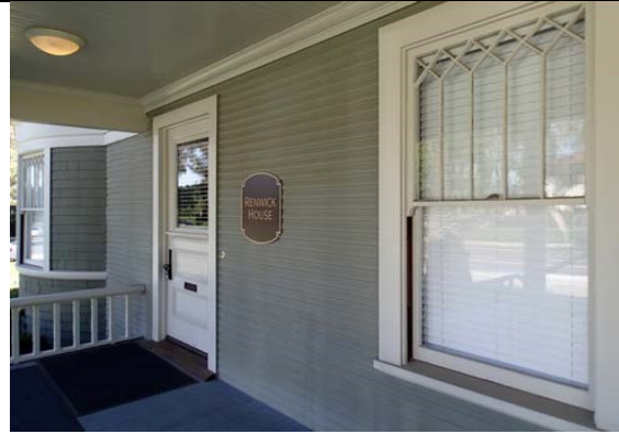
View south of front door within porch.
