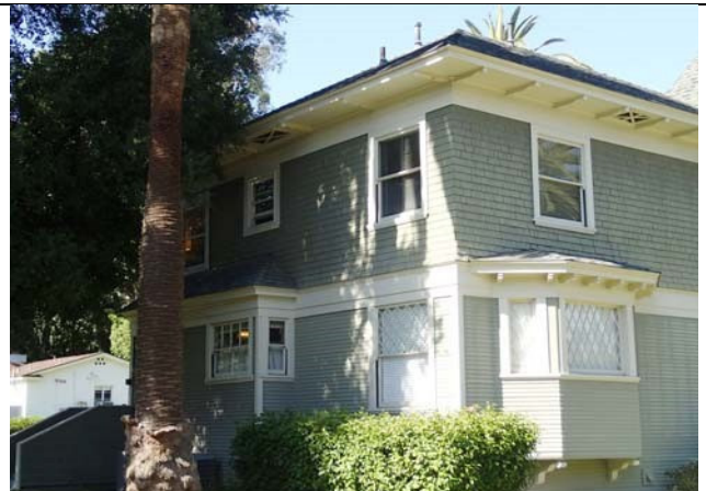
View northeast of west and south facades.
