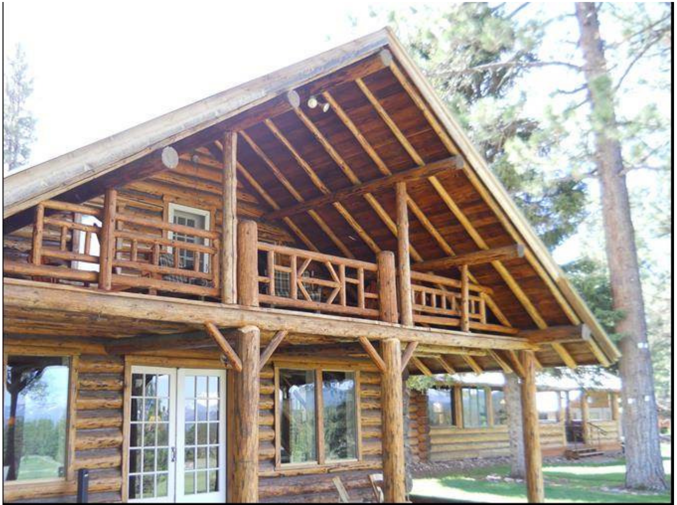
Photo 0009. Detail of balcony railing. View to the southwest.
