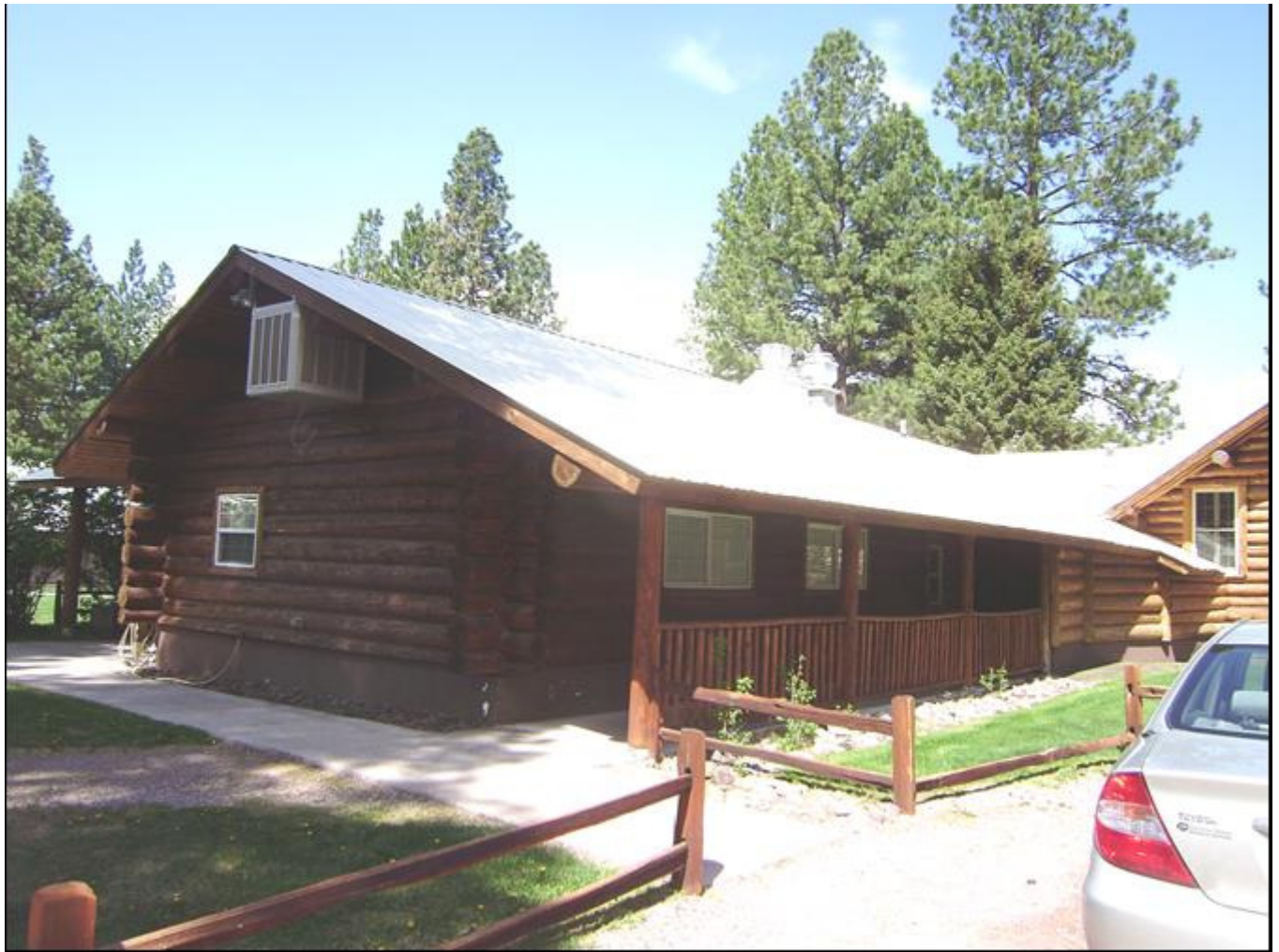
Photo 0015. South elevation and east side of 2002 addition. View to north-northwest.
