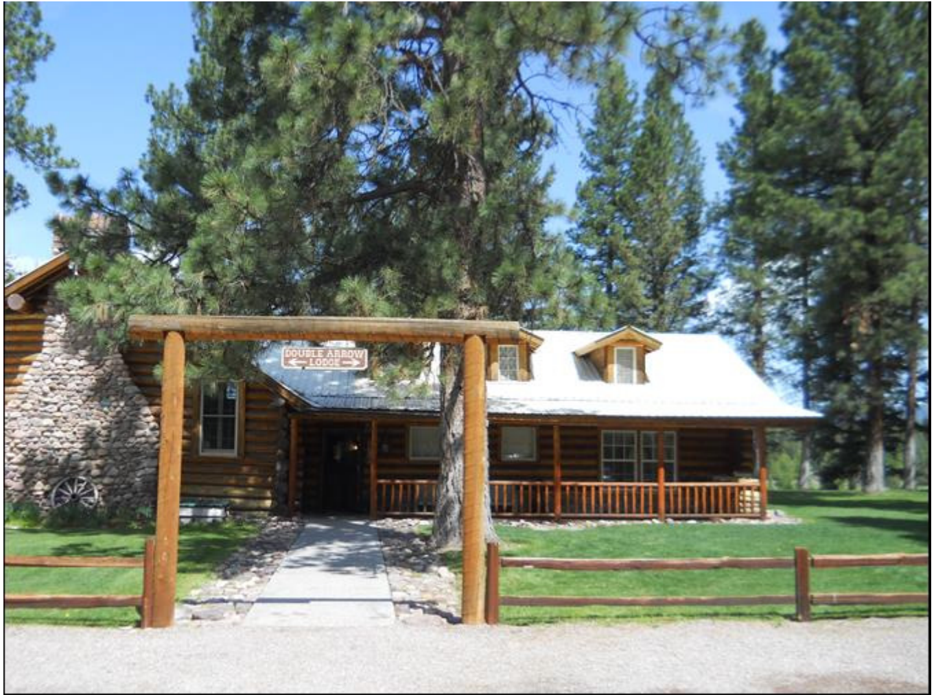
Photo 0002. Façade of Double Arrow Lodge. View to north.
