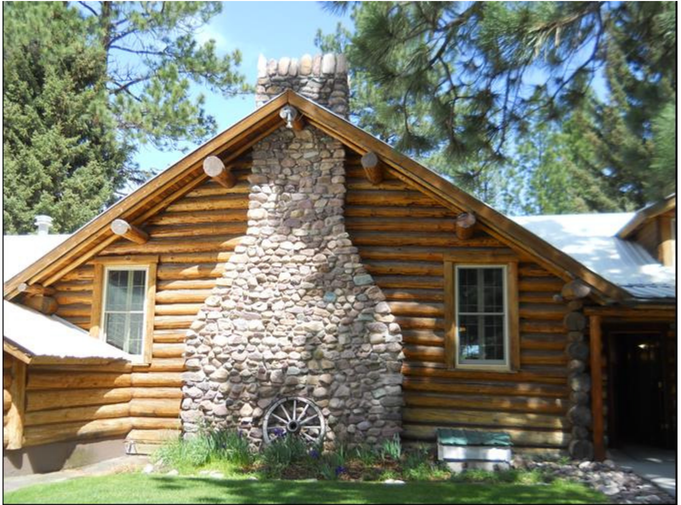
Photo 0004. Detail of cobblestone chimney. View to north.
