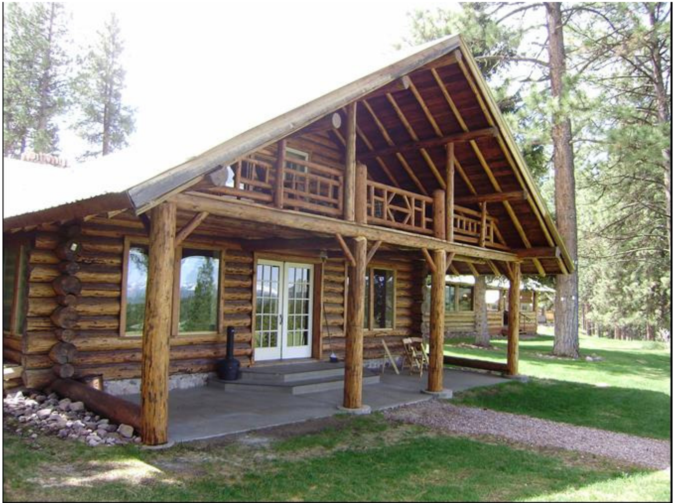
Photo 0008. Detail of north patio and balcony. View to southwest.
