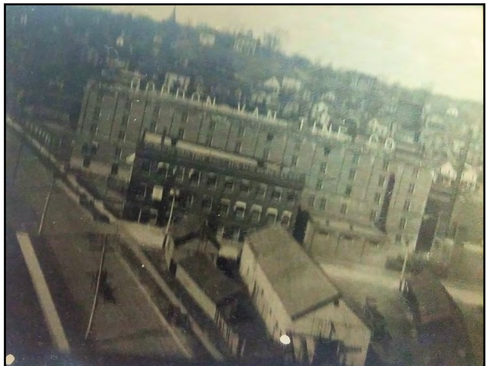
Figure22 Early photograph of the Gordon-Van Tine Buildings Facing Federal Street, c.1910-15 (Courtesy of Ralph Christian)
