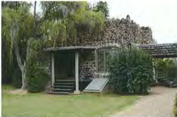
Figure 11. Northwest porch, kitchen window and cellar door, looking south-southeast.
