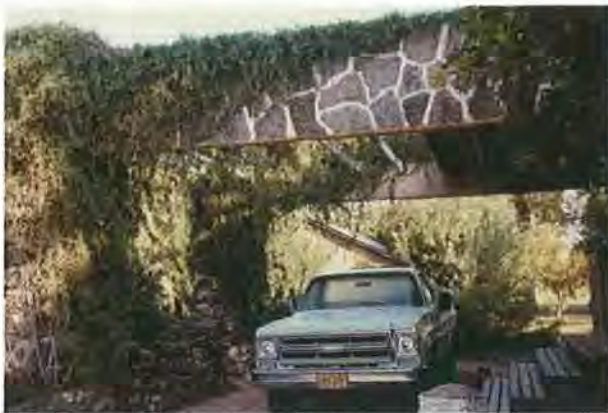
Figure 13. Porte cochere before replacement, looking north.
