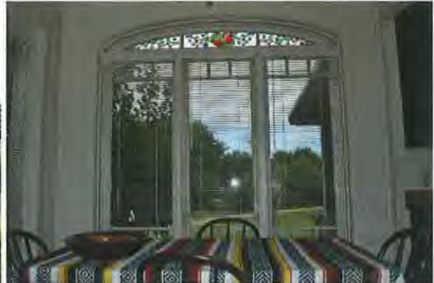
Figure 12. North kitchen window, looking north.
