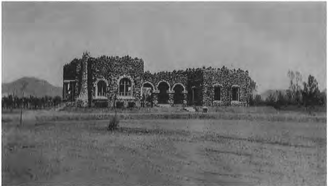
Figure 2. Hilgeman House nearing completion, looking north-northeast, circa 1924.
