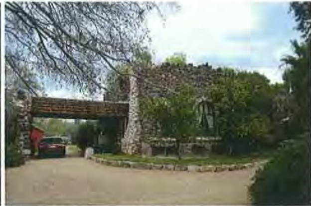
Figure 14. Porte cochere after replacement, looking north.
