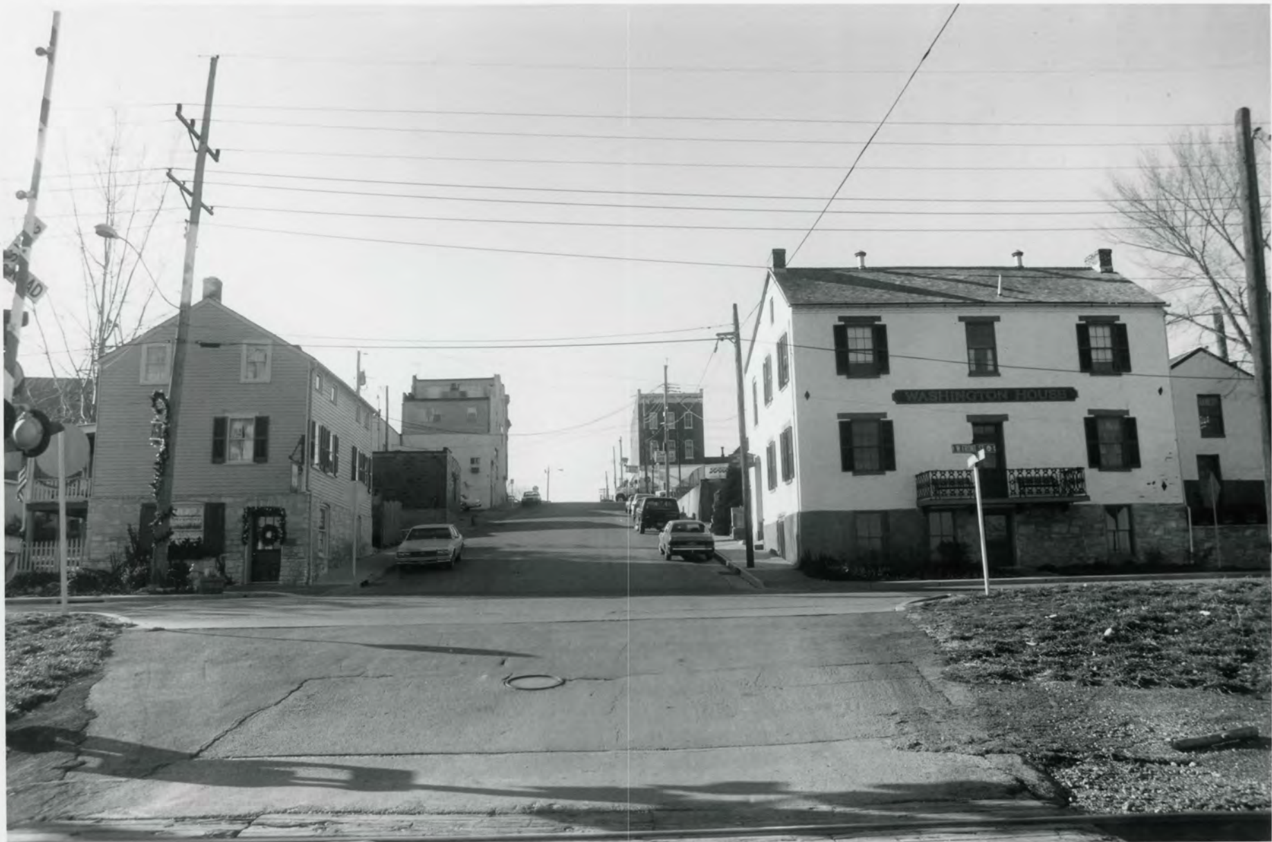
1 Intersection Front & Lafayette, Downtown Washington Historic District Franklin Co., MO camera facing south
