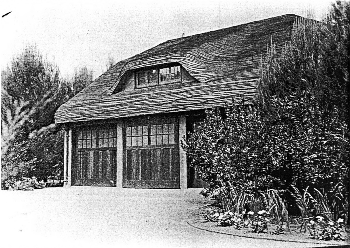
Historic view of Ainsley House garage (carriage house) in original location circa mid-1930s, viewed looking northwest. Original on file at Campbell Historical Museum and Ainsley House.
