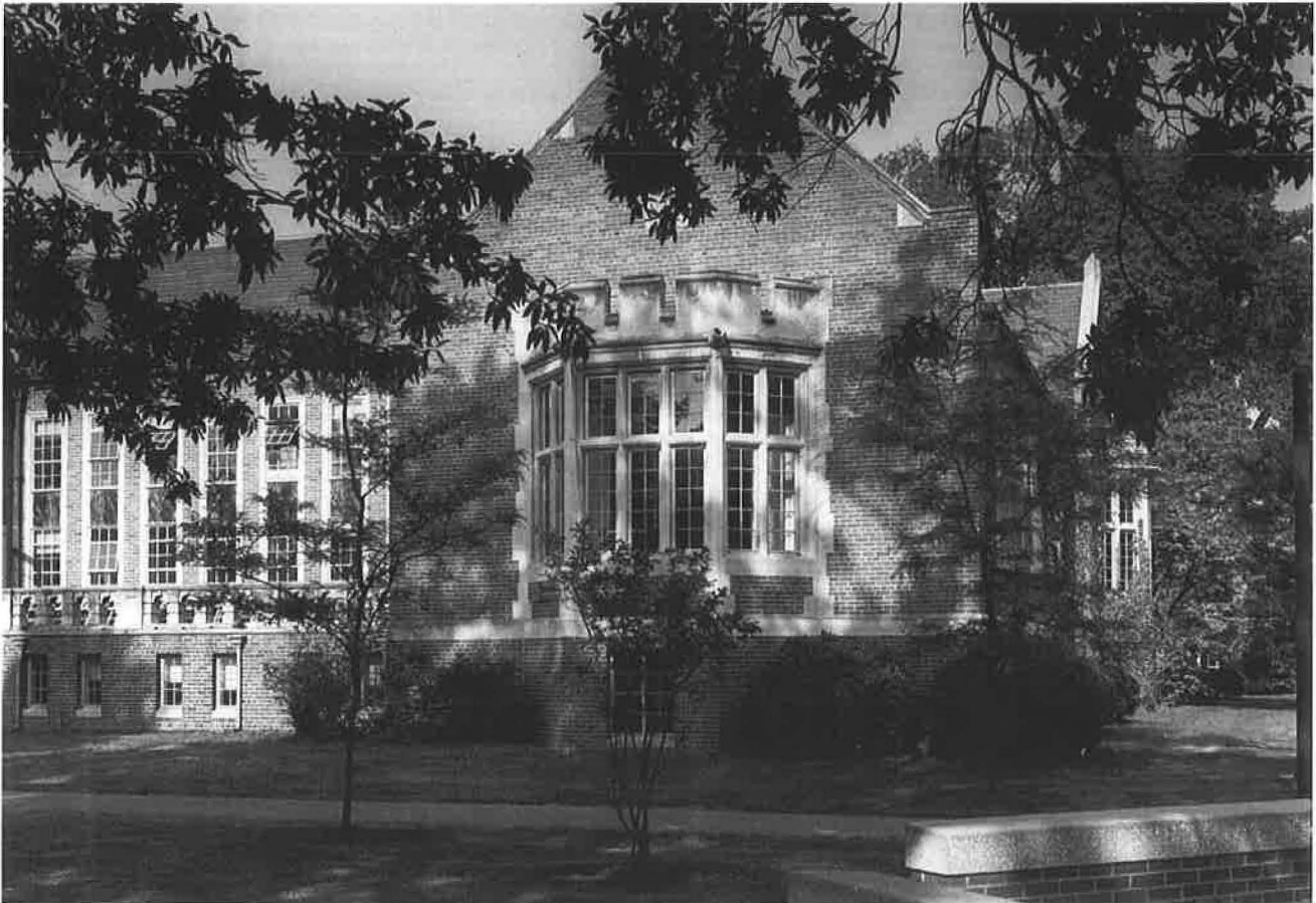
FIGURE 23 – Rudolph Memorial Library c.1980, before rear glass enclosure added; Capital University Archives.
