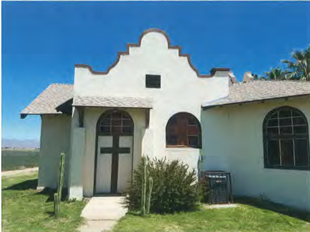
Image 1 – South Elevation showing original primary entrance, and the Mission Revival parapet, the signature detail that establishes the stylistic identity.
