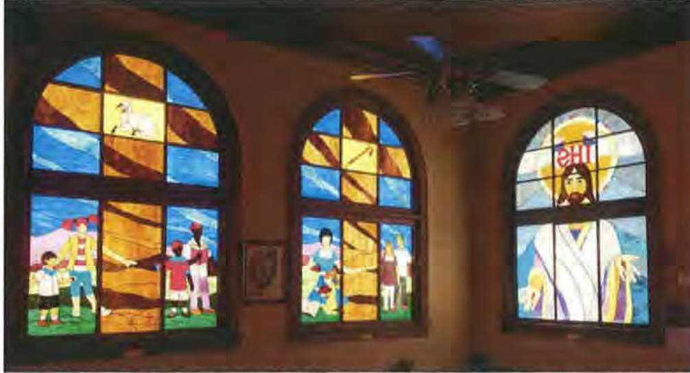
Image 4: Stained-glass installed within the form and framing of the original window sash and muntins. These windows are located on the north and east-facing walls of the sanctuary.
