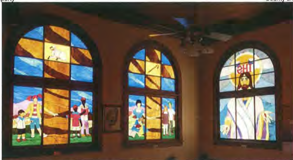
Image 4: Stained-glass installed within the form and framing of the original window sash and muntins. These windows are located on the north and east-facing walls of the sanctuary.
