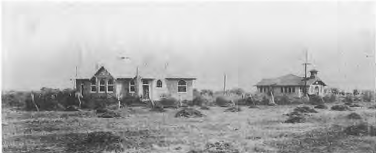
Image 5 – The Liberty United Methodist Church (south elevation) stands in the foreground. The Liberty School stands immediately to the east. They are in close proximity and have always been mutually supportive. The school dates to 1910, completed just prior to the church. (Photo from Liberty Church archives)
