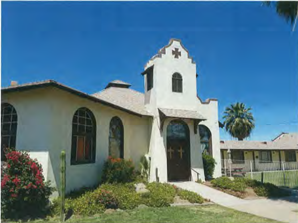
Image 2: Bell tower, and current entry, facing the southeast. Note the new stained glass windows over the door, and to the left and right.
