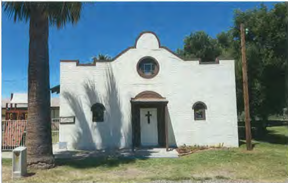
Image 8 Façade of Memorial Hall/Fellowship Hall, completed in 1948. The Mission parapet clearly mimics the south elevation and stylistic features of the church.
