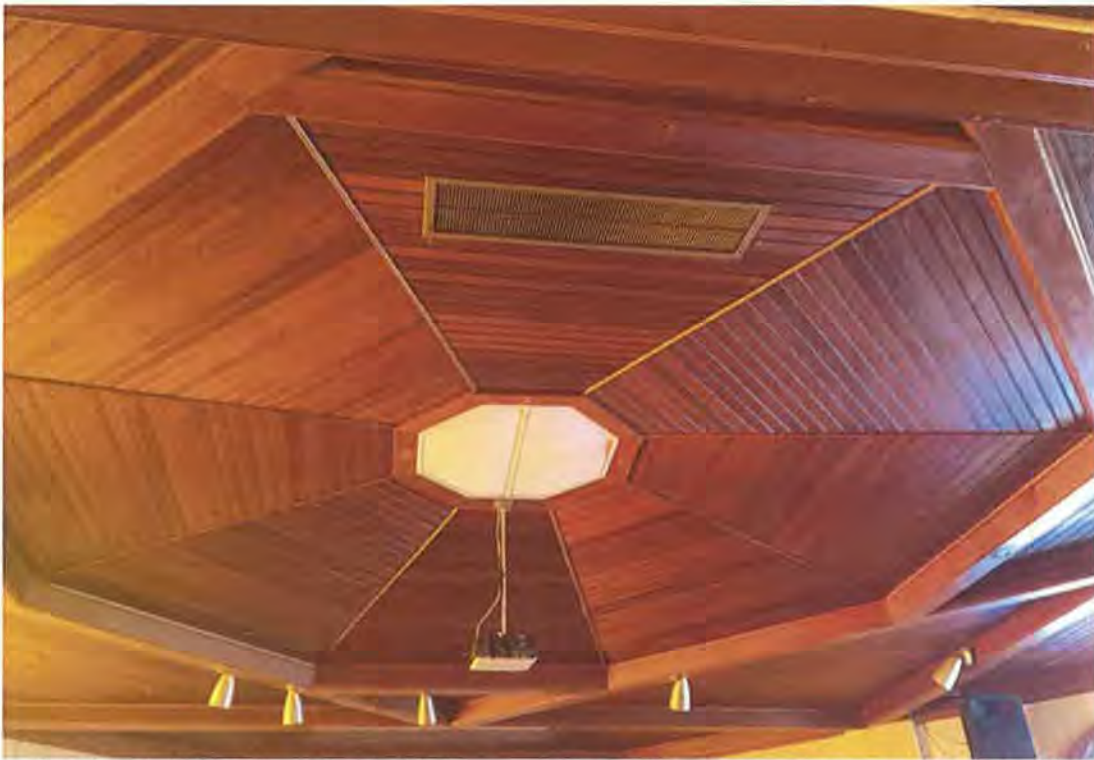
Image 3: The ceiling is oak, laid in an octagonal pattern that corresponds with the ceiling framing that allows the clear-span over the main sanctuary. (The ceiling is below a standard pyramidal roof, the actual roof structure is not an octagonal form.)
