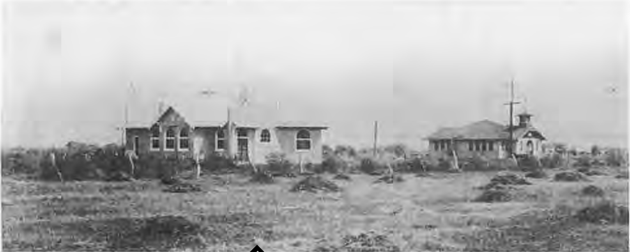
Image 5 - The Liberty United Methodist Church (south elevation) stands in the foreground. The Liberty School stands immediately to the east. They are in close proximity and have always been mutually supportive. The school dates to 1910, completed just prior to the church. (Photo from Liberty Church archives)
