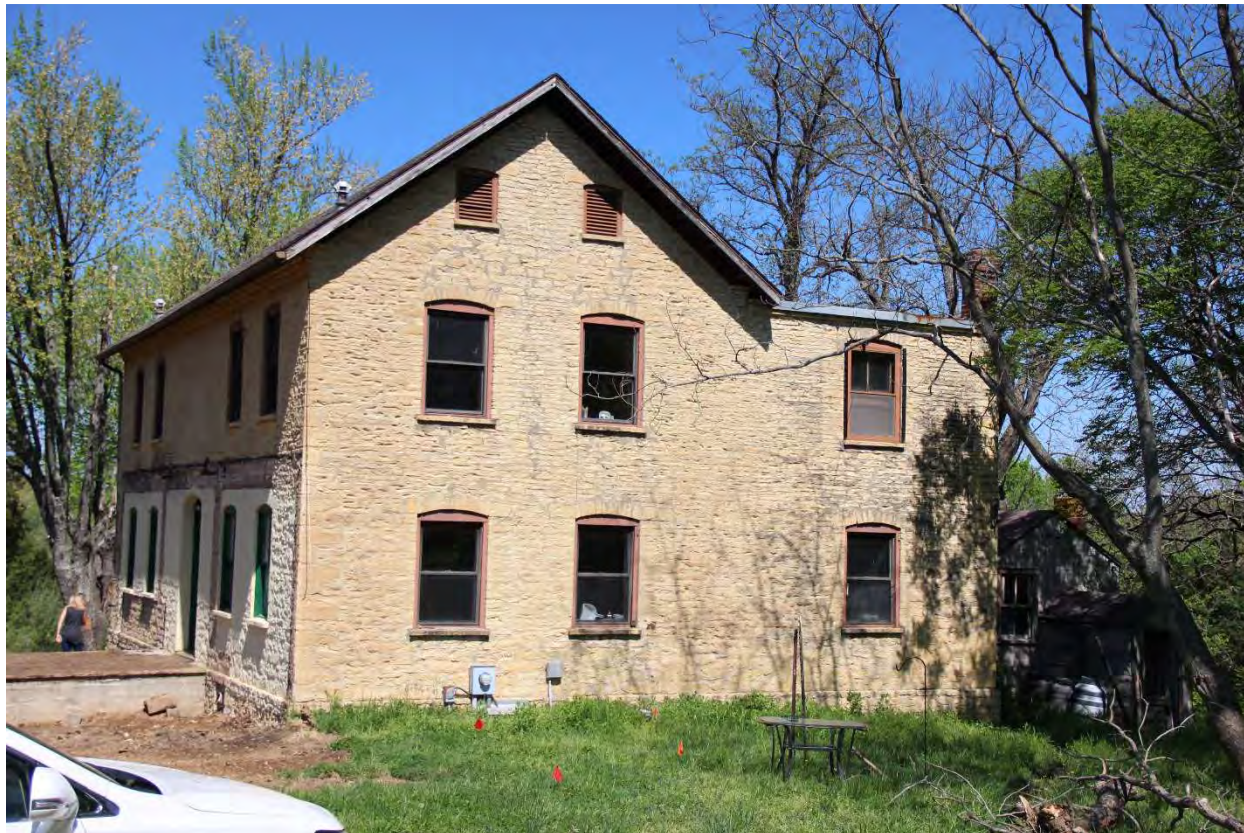
9 of 16: House, East Wall. Camera facing northwest.
