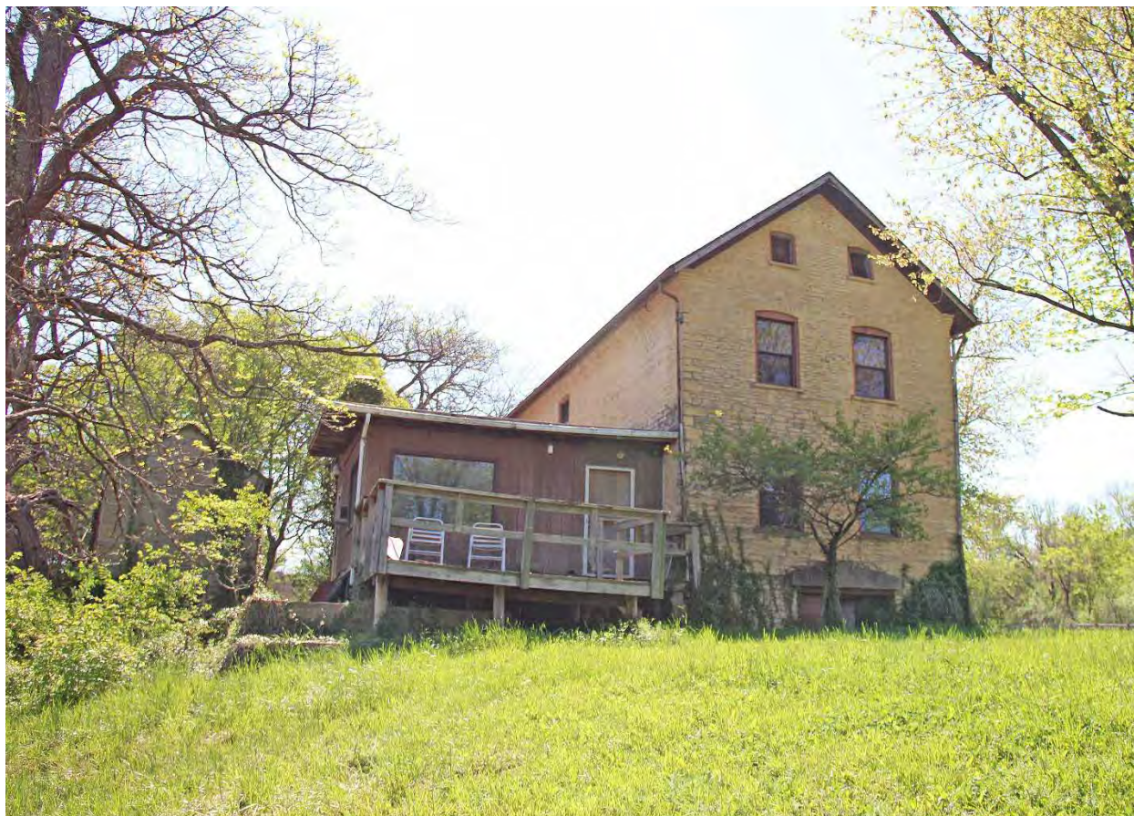
4 of 16: House, West Wall. Camera facing southeast.
