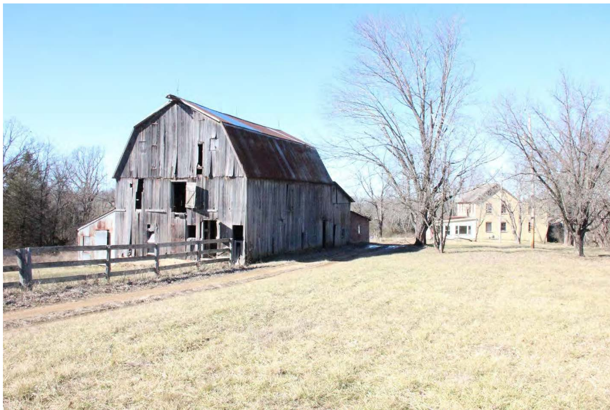
14 of 16: Barn. Camera facing northwest.
