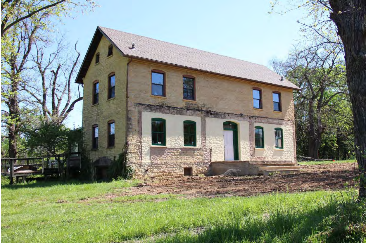
3 of 16: House, Southwest Corner. Camera facing east.
