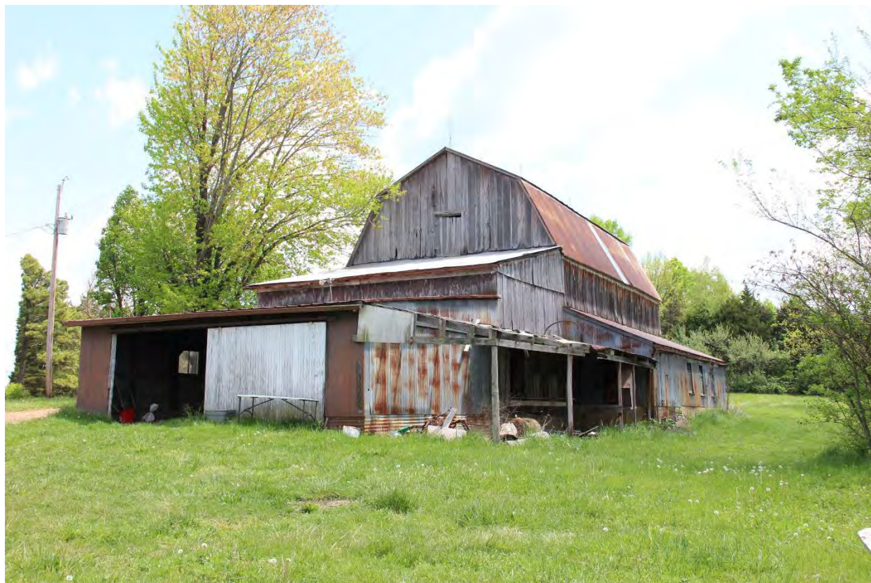
15 of 16: Barn. Camera facing east.
