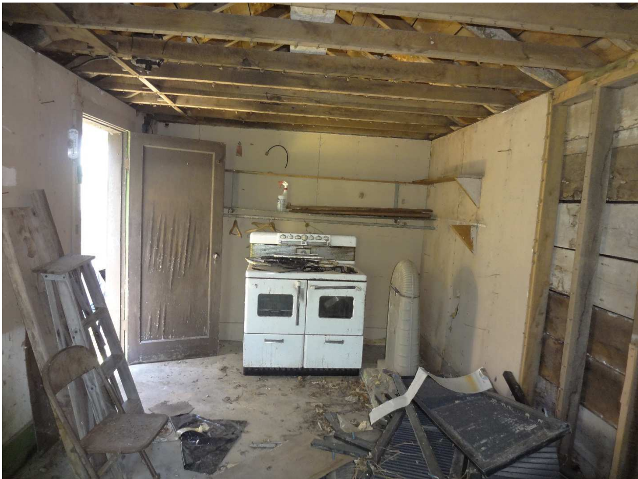
7 of 16: Summer Kitchen, interior. Camera facing northwest.
