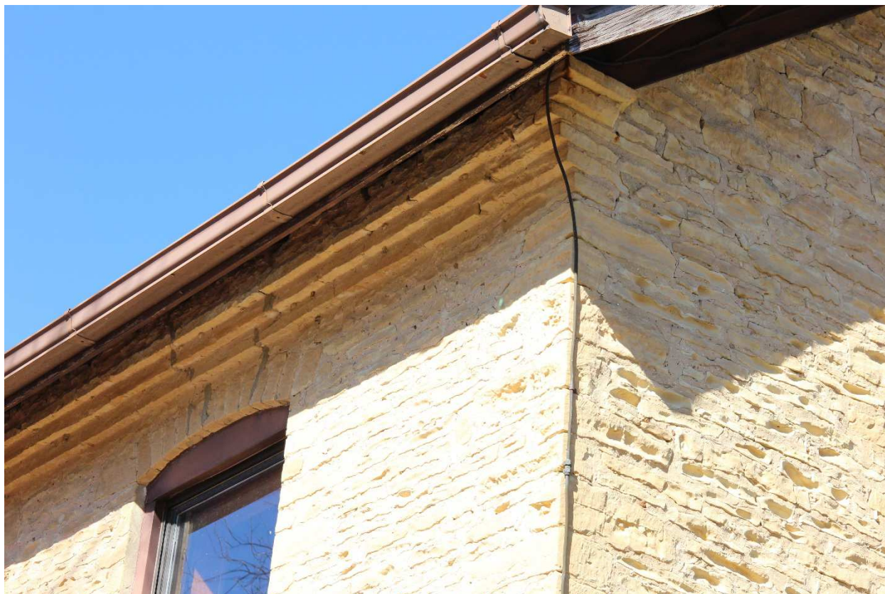
10 of 16: House, Southeast Corner, Stone Detail. Camera facing northwest.
