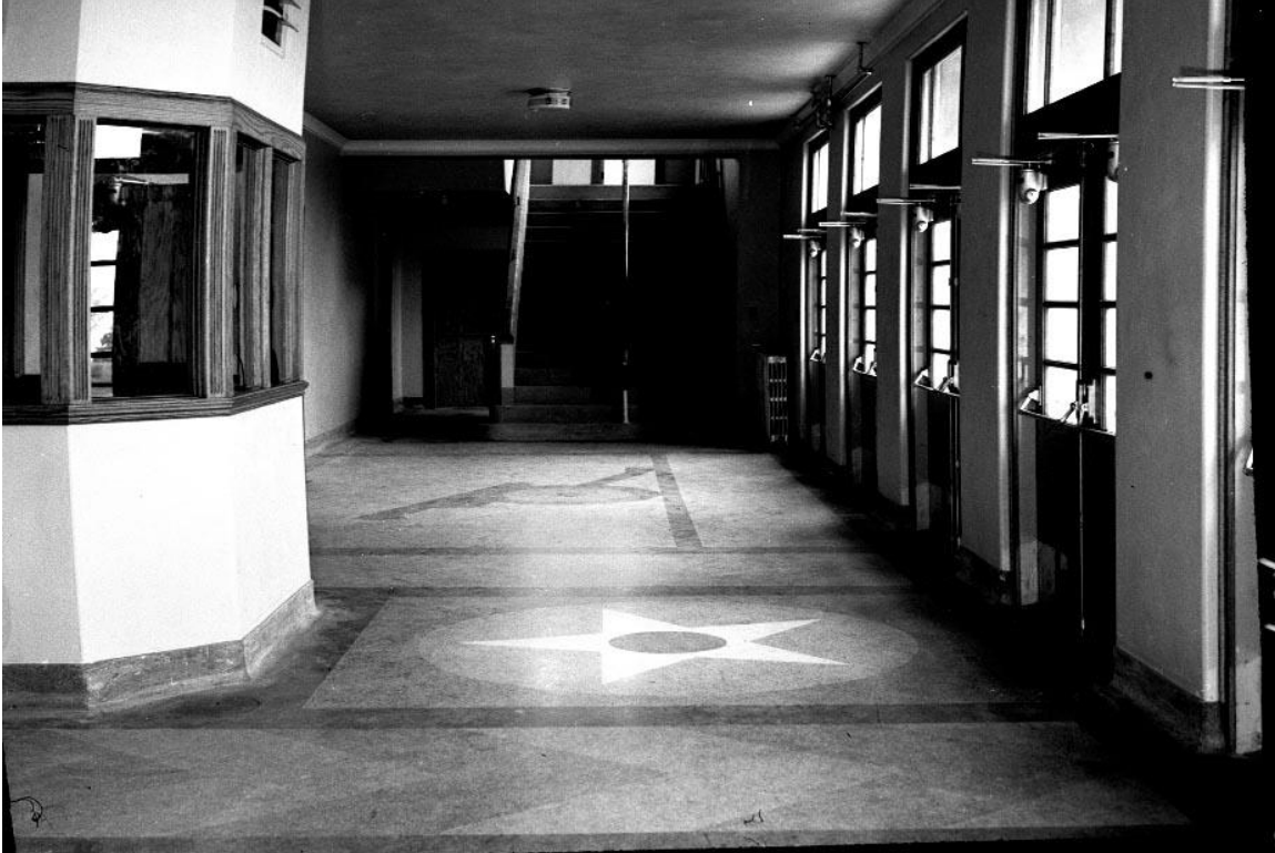
Figure 9: Sheboygan Municipal Auditorium and Armory upon completion - Lobby, Summer 1942. Photo Courtesy of the Sheboygan County Historical Research Center.
