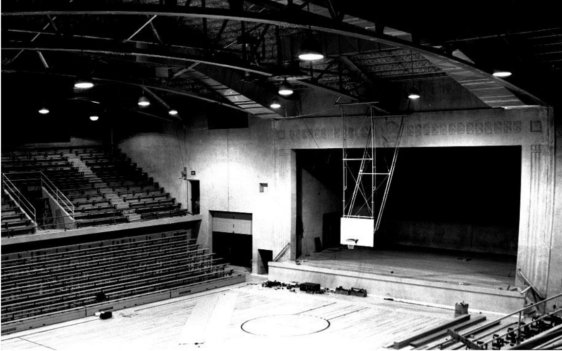
Figure 10: Sheboygan Municipal Auditorium and Armory upon completion -Drill Hall, Summer 1942. Photo Courtesy of the Sheboygan County Historical Research Center.
