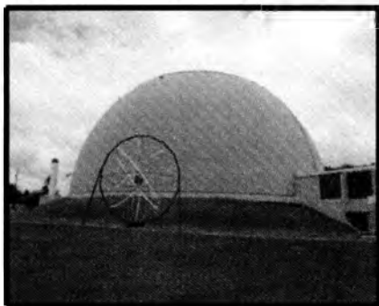
Fig. 3. The Domed Building
