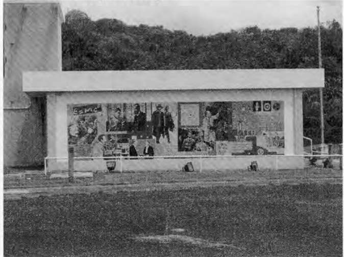
Entrance Building, west wing.
