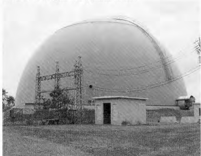
Domed Building and relay power station.
