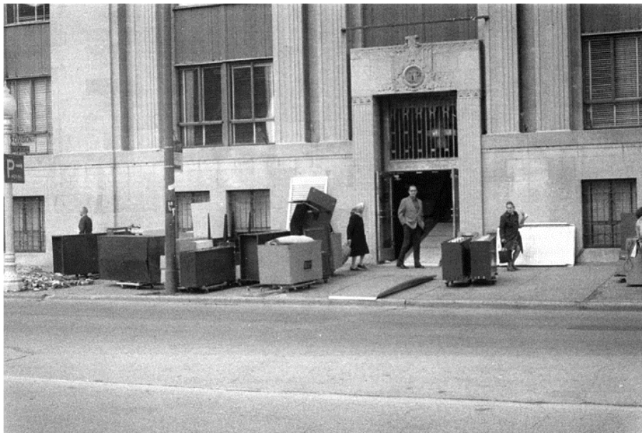
Figure 07. Main entrance circa 1976, looking north (photo courtesy of the Polish National Alliance)
