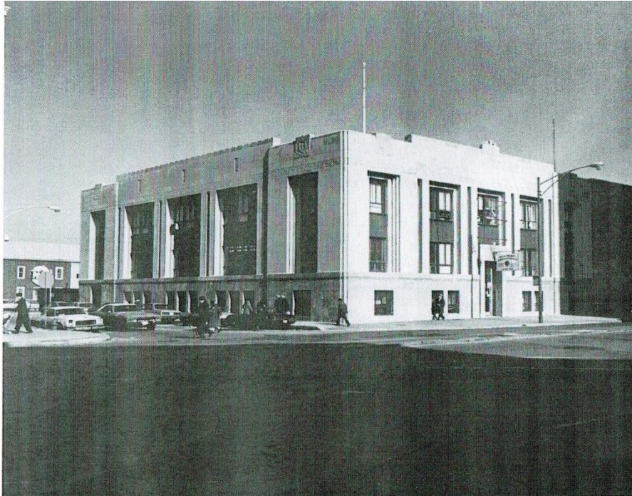
Figure 06. South and east elevations circa 1976, looking northwest along West Division Street (photo courtesy of the Polish National Alliance)
