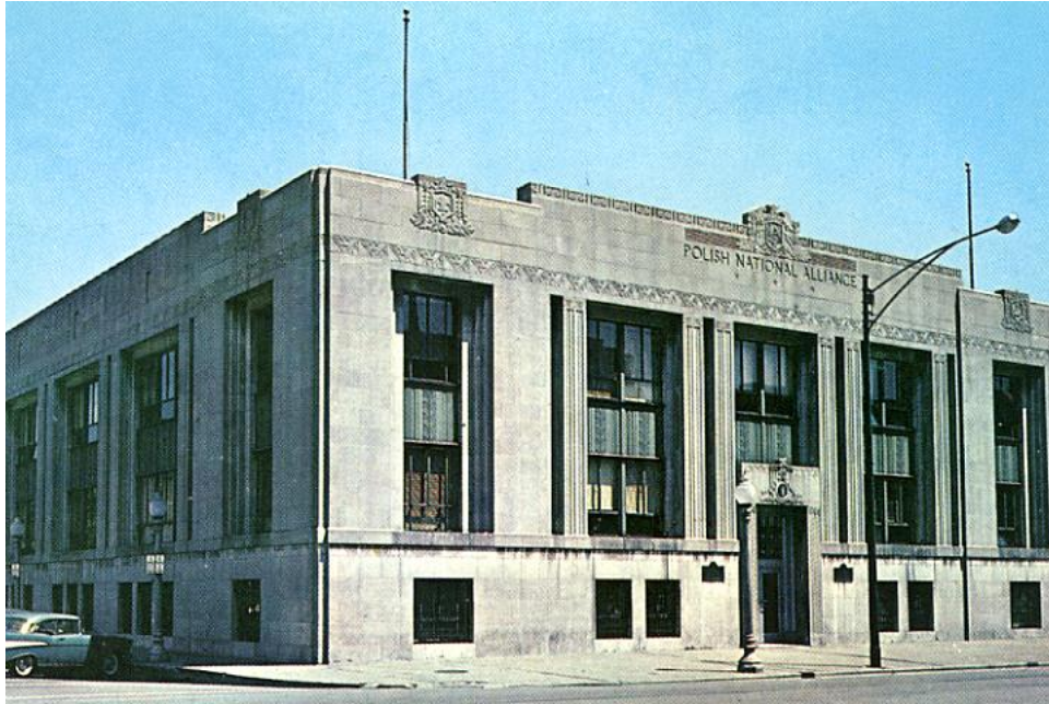
Figure 04. South elevation circa 1976, looking northeast along West Division Street
