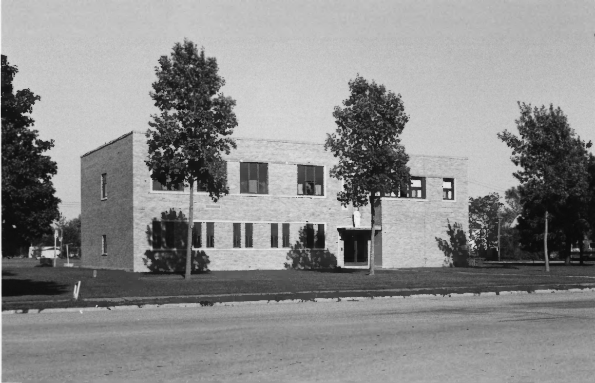
ST. PETER'S CATHOLIC CHURCH, JEFFERSON, UNION COUNTY, SD, PHOTO # 1
