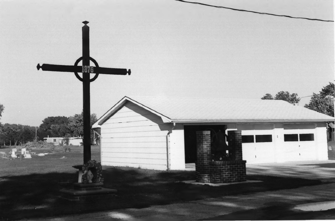
ST. PETER'S CATHOLIC CHURCH, JEFFERSON, UNION COUNTY, SD, PHOTO # 13
