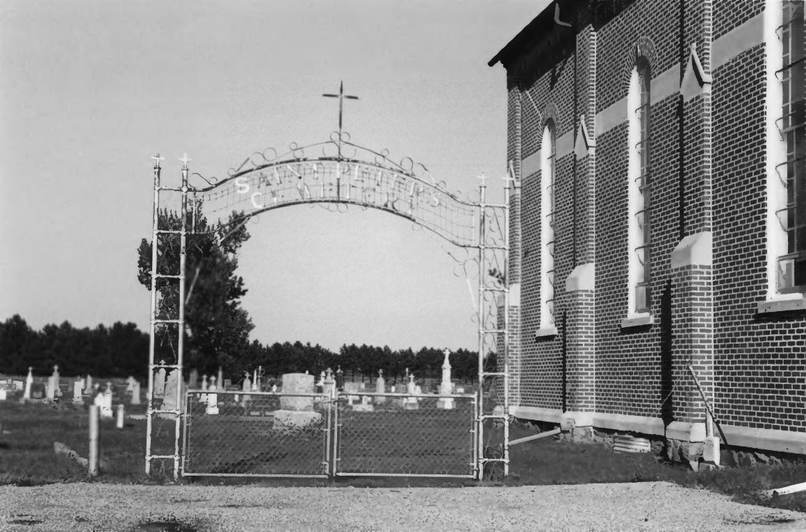
ST. PETER'S CATHOLIC CHURCH, JEFFERSON, UNION COUNTY, SD, PHOTO # 10
