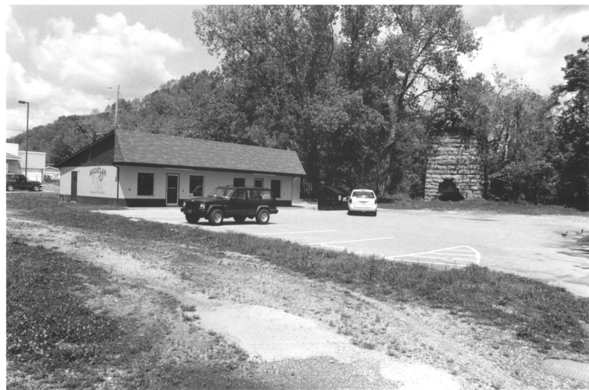
QUARRY LIMEKILN HOUSTON COUNTY TN
