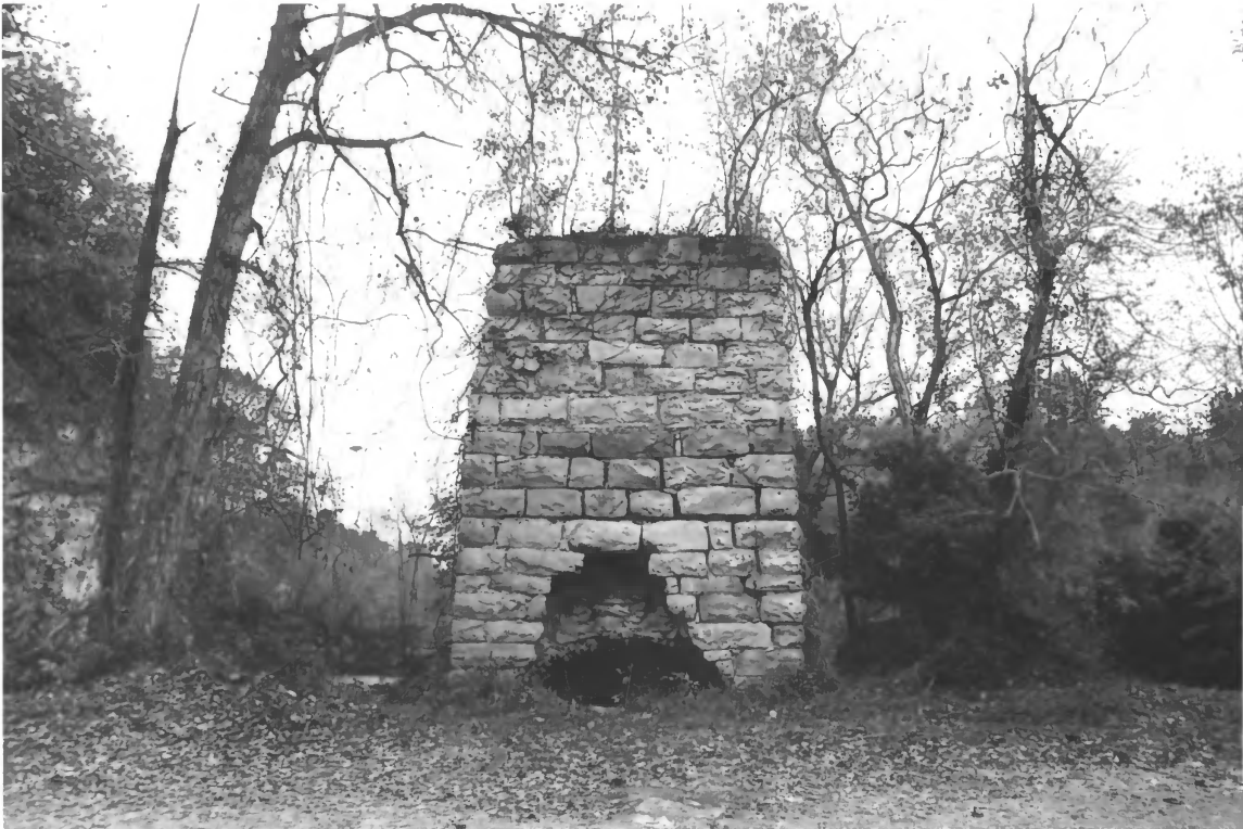
QUARRY LIMEKILN HOUSTON COUNTY TN
