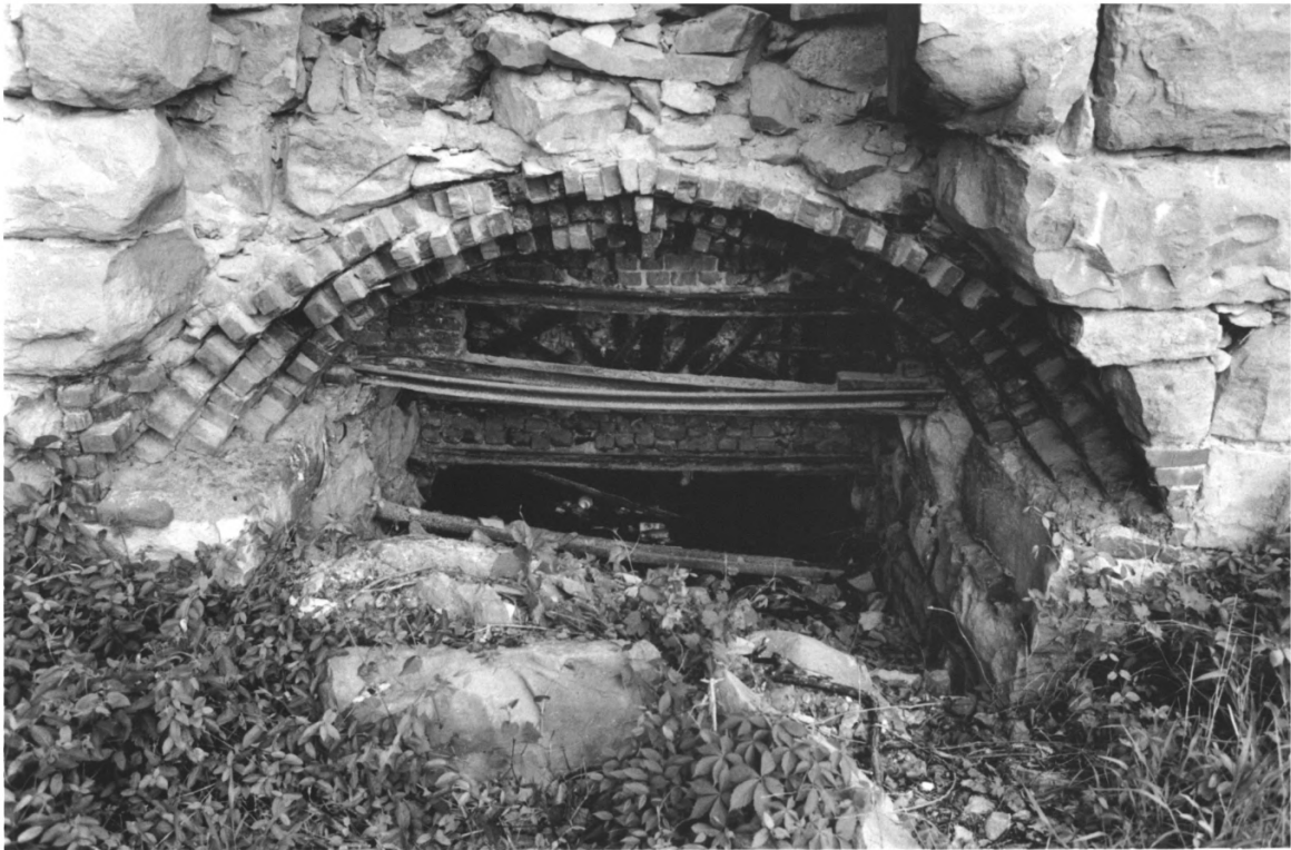
QUARRY LIMEKILN HOUSTON COUNTY TN
