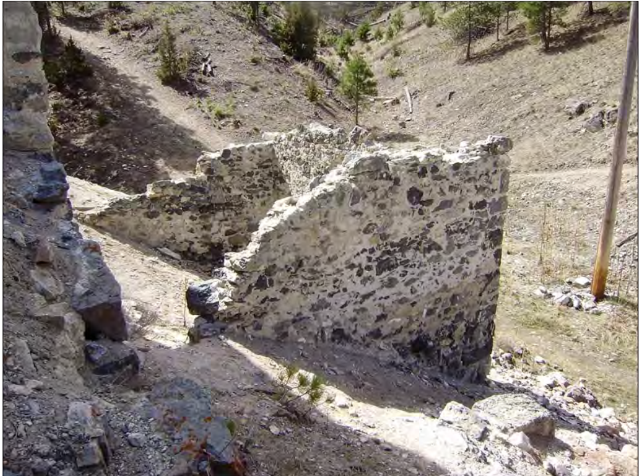
Photo #0006: The Grant-Marshall Lime Kiln Historic District. Cooling shed. View to the southwest. Photo date: April 4, 2017.
