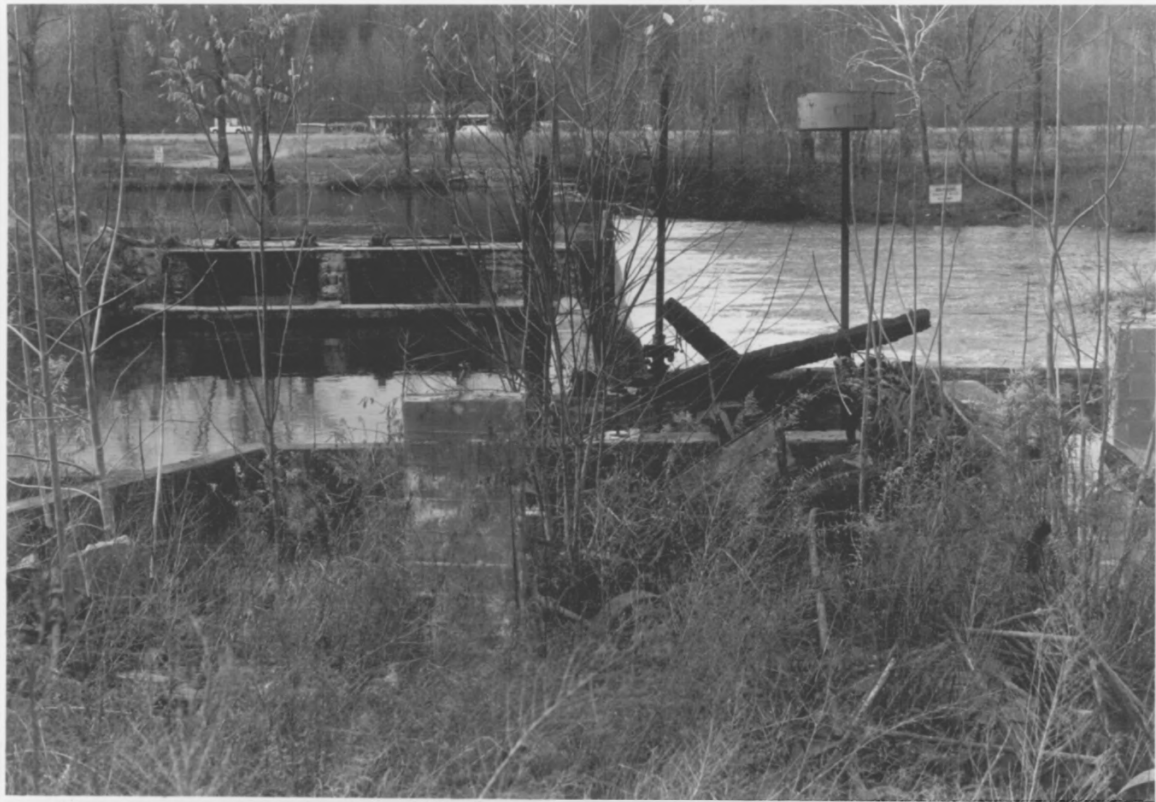
Peery Mill Site, Blount Co., TN, Photo 1 of 2
