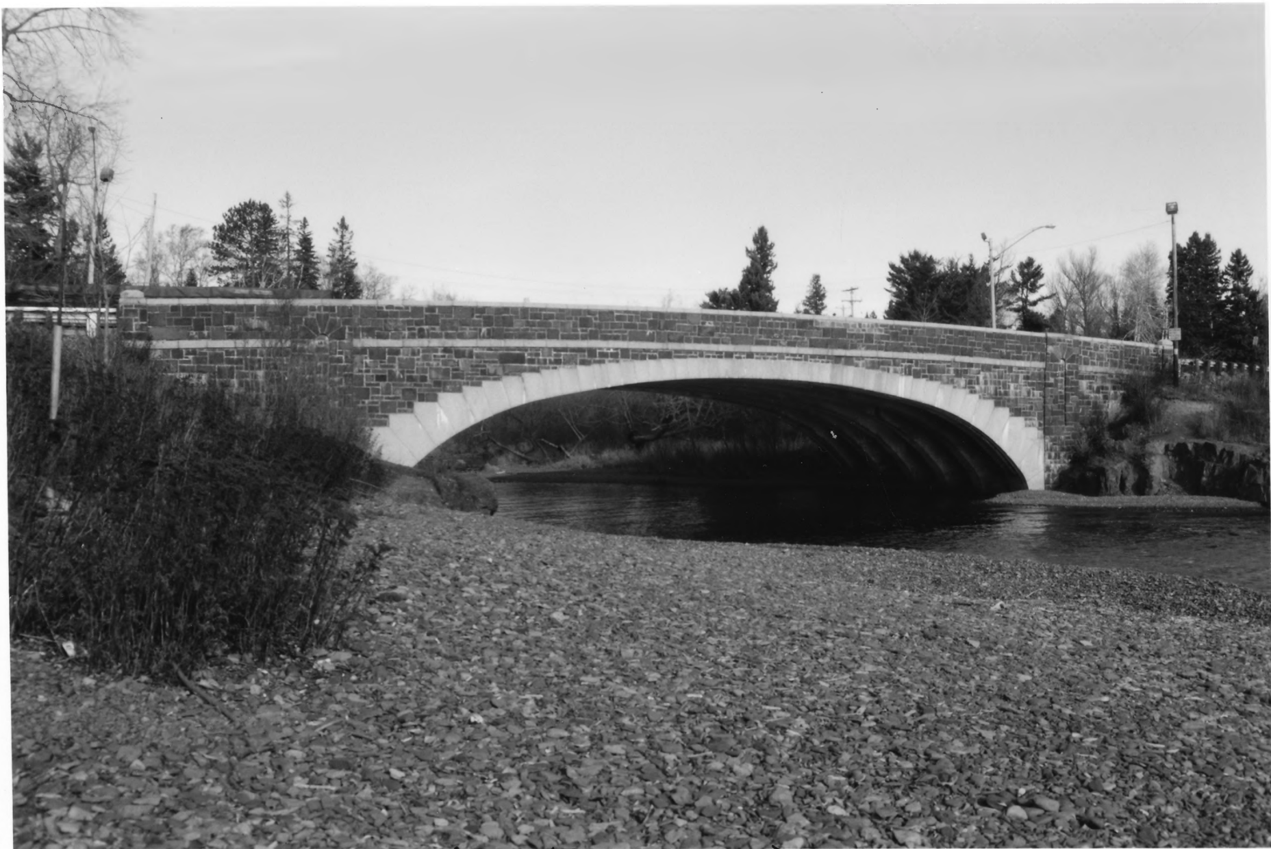
Lester River Bridge (Bridge no. 5772) St. Louis Co., MN
