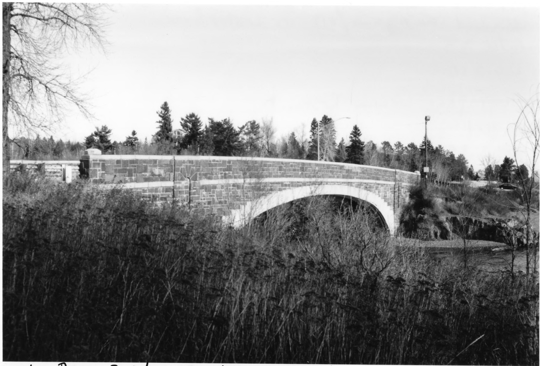
Lester River Bridge (Bridge No. 5772)
