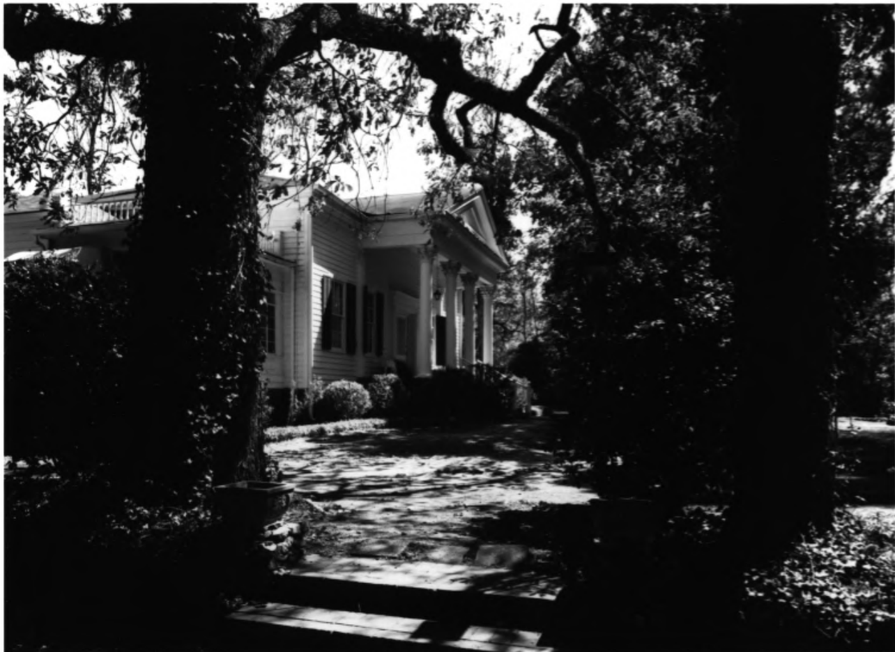
FORT-HAMMOND-WILLIS HOUSE BALDWIN COUNTY, GA PHOTO 2 OF 18
